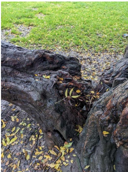
Large limb fallen from T17. Cracked at base.
