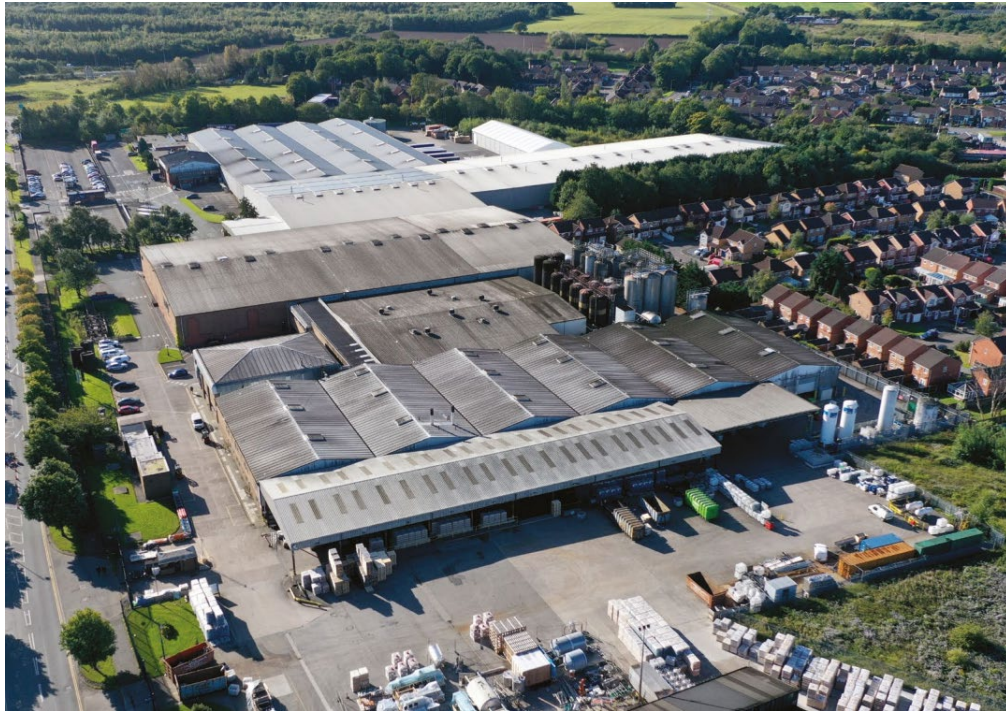
Figure 3 – Aerial view of Existing Site
