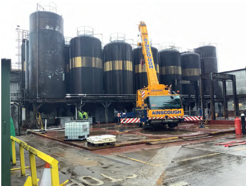
Photo Plate No. 09: Removal of distilling and process plant.
