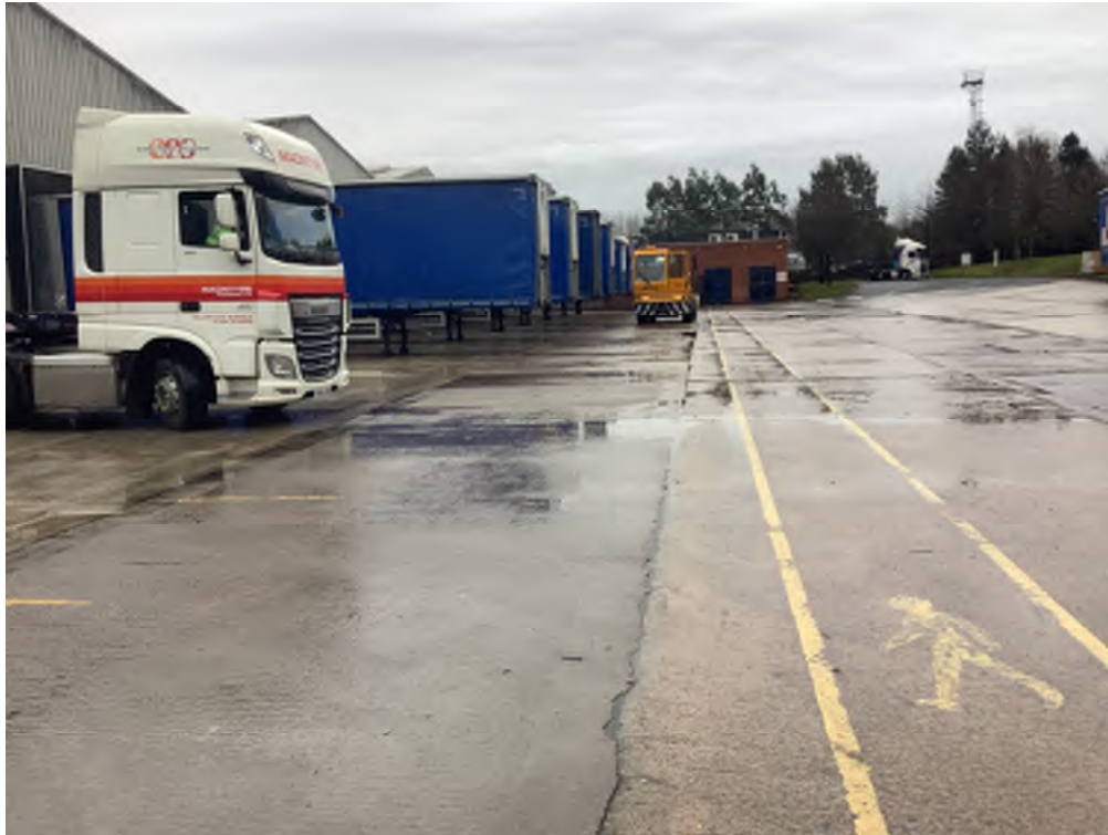
Photo Plate No. 17: Docking levelers for the wagons
