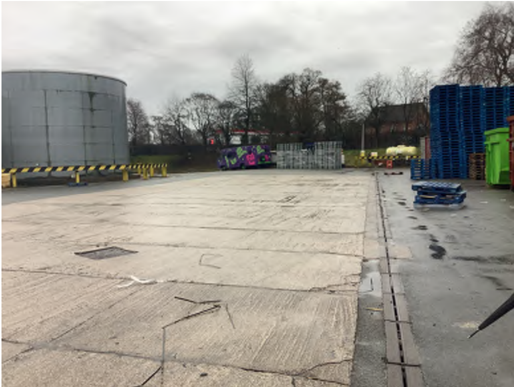
Photo Plate No. 15: Fire water tank , further propane tanks & LPR canisters.
