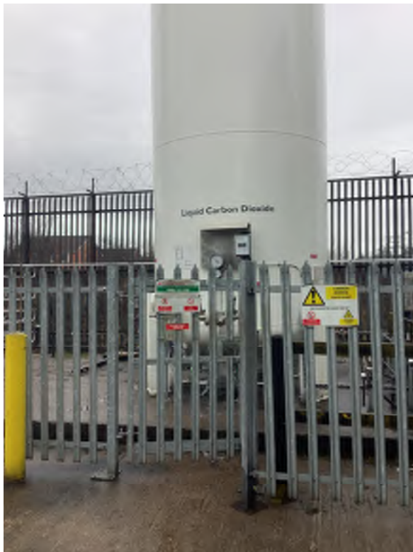
Photo Plate No. 07: Liquid Carbon Dioxide & Liquid Nitrogen Tanks
