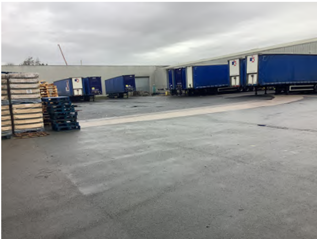
Photo Plate No. 16: Storage area
