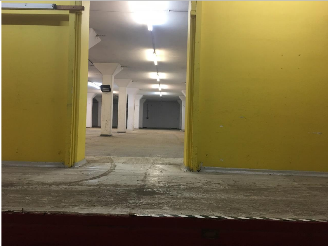
PLATE 7 INSIDE THE NORTHERN BUNKER
