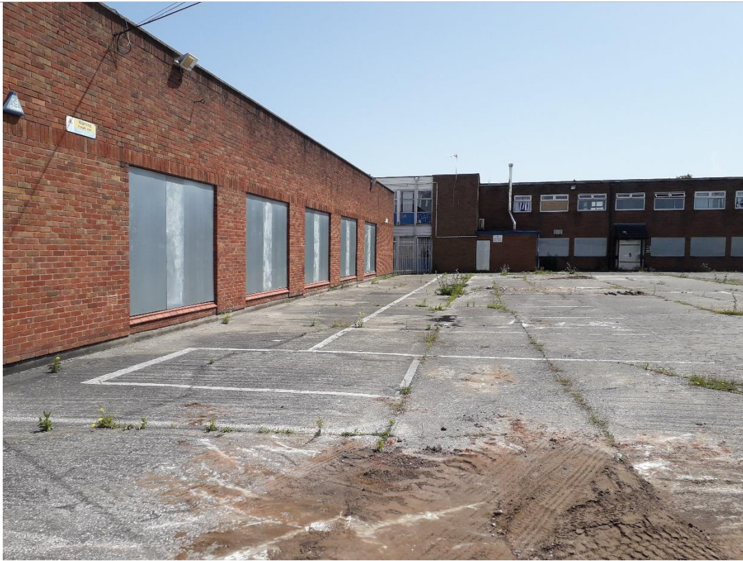
PLATE 3 THE CURRENT BUILDING IN THE NORTH OF THE SITE
