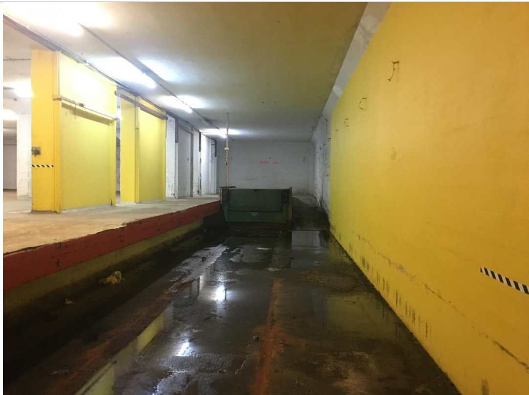
PLATE 5 INSIDE THE NORTHERN BUNKER
