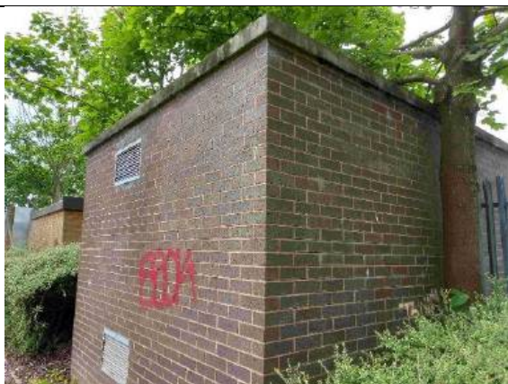
Photograph 19: Electrical substation (TN2)
