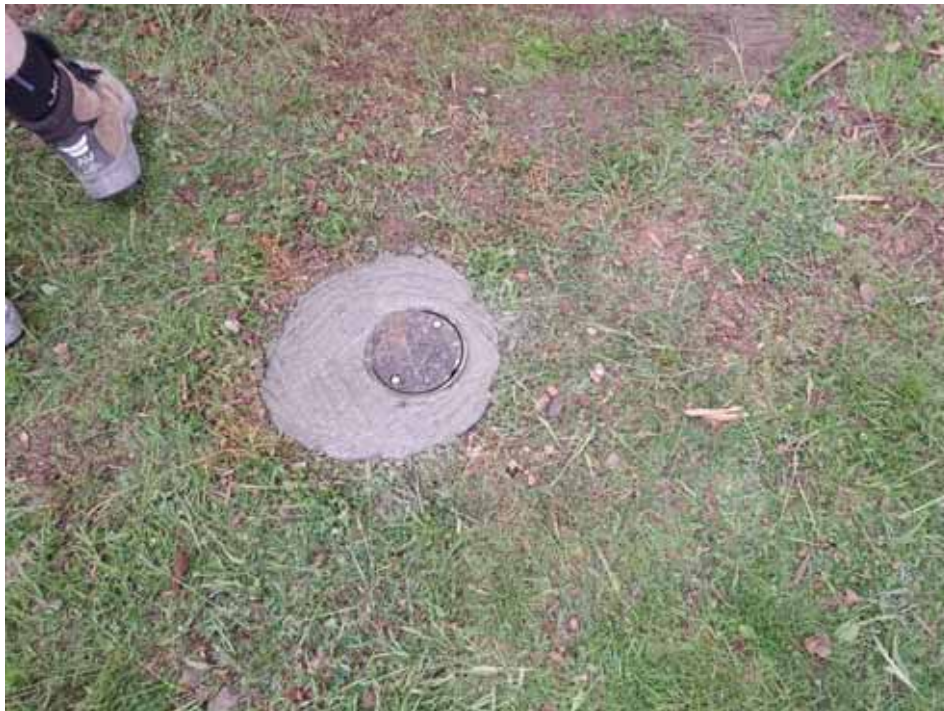
Photograph 13 WS106 following installation
