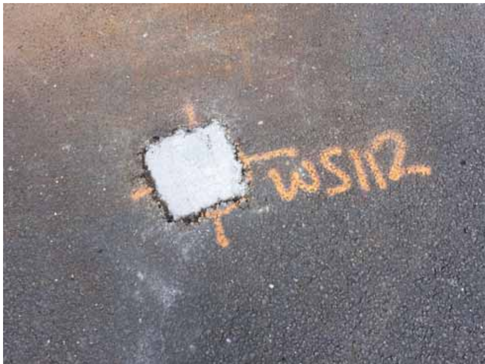
Photograph 26 WS112 following reinstatement
