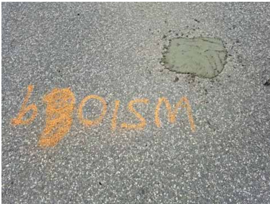
Photograph 18 WS109 following reinstatement
