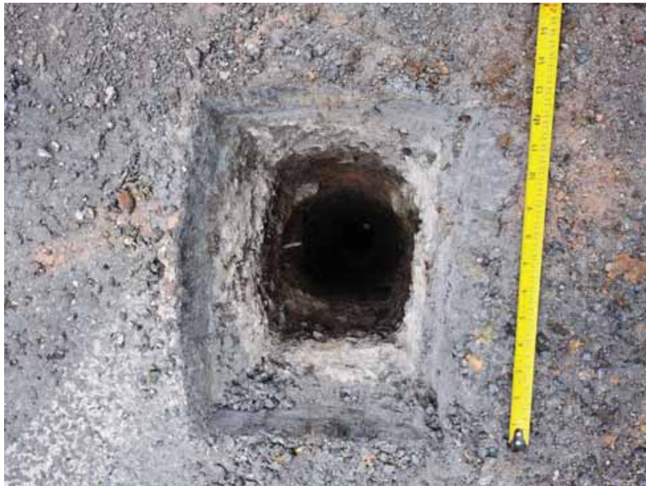
Photograph 19 WS110 inspection pit
