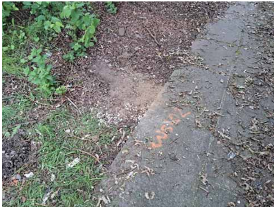
Photograph 3 WS102 following reinstatement
