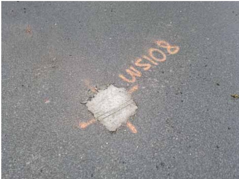
Photograph 16 WS108 following reinstatement
