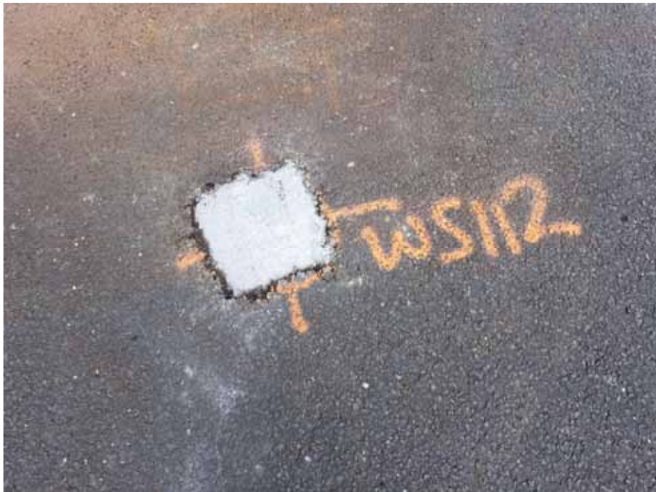
Photograph 26 WS112 following reinstatement
