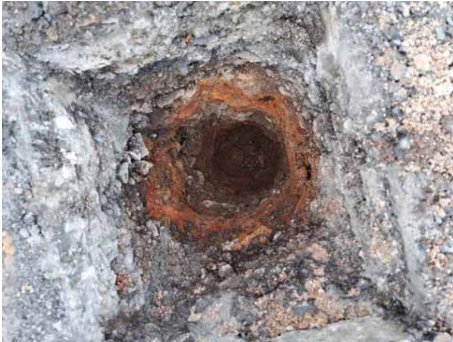
Photograph 15 WS108 inspection pit
