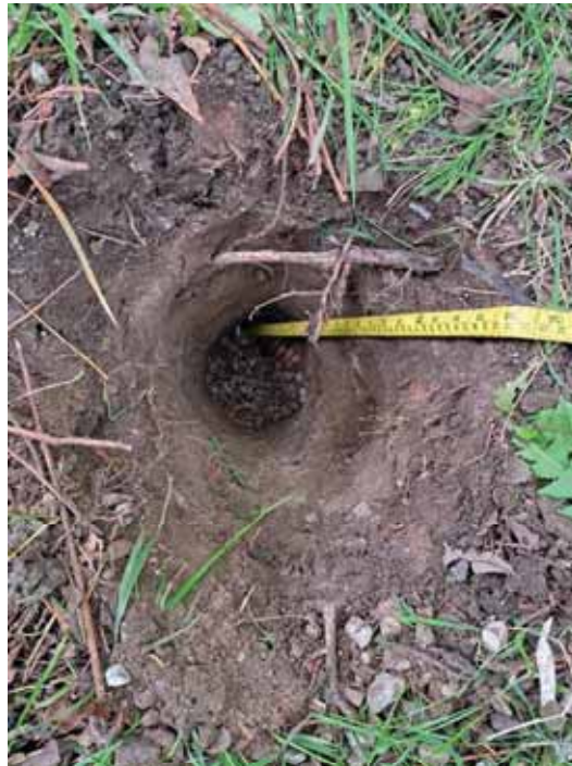
Photograph 1 WS102 inspection pit
