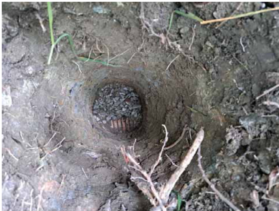
Photograph 2 WS102 inspection pit showing plastic utility at base of pit
