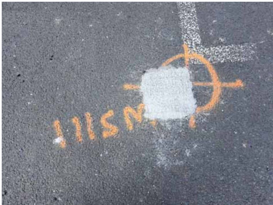
Photograph 24 WS111 following reinstatement
