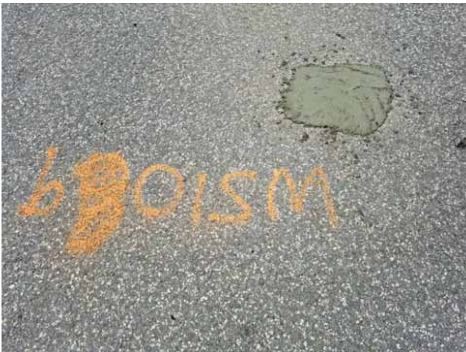
Photograph 18 WS109 following reinstatement
