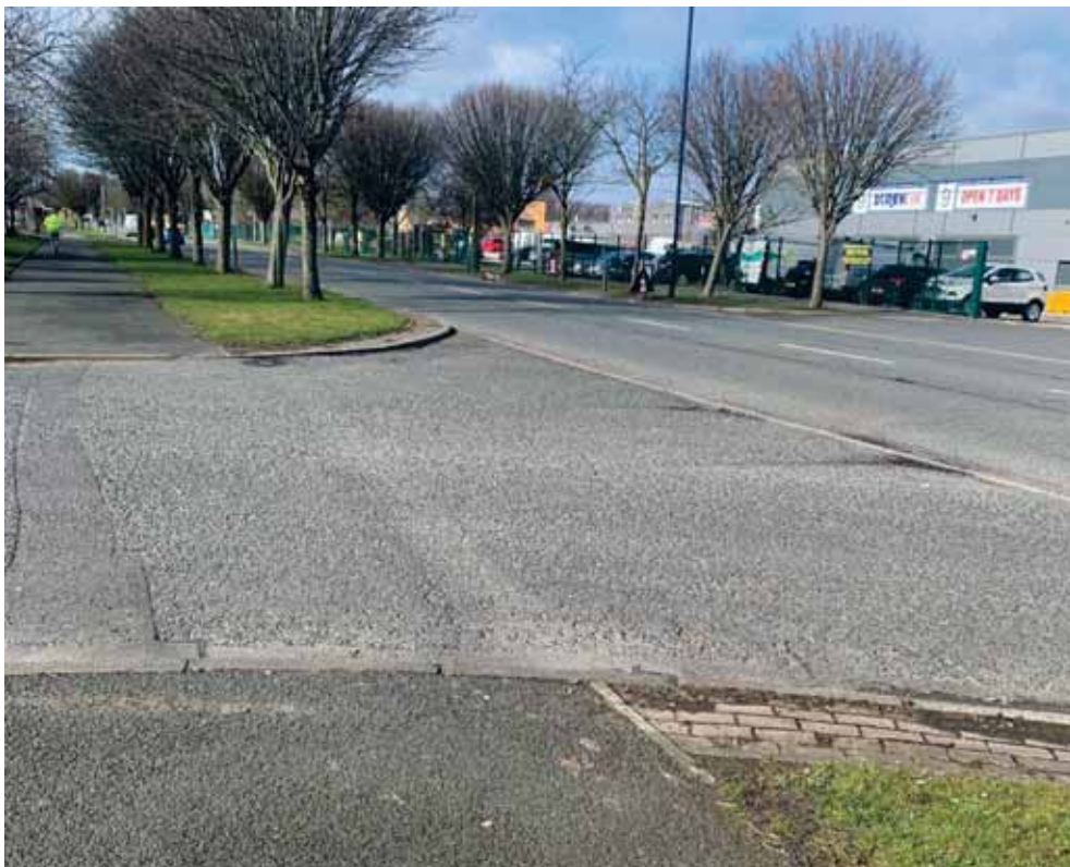
Photograph 8 Existing access from Wilson Road in the north-east.
