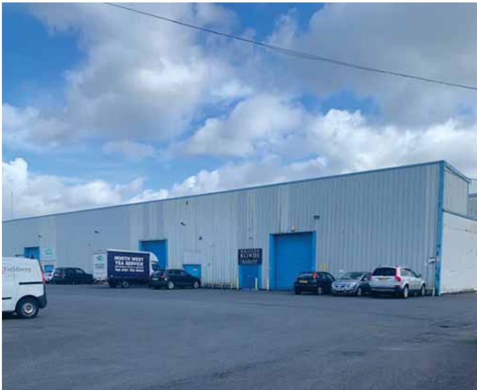
Photograph 12 Typical structures in the central site area.
