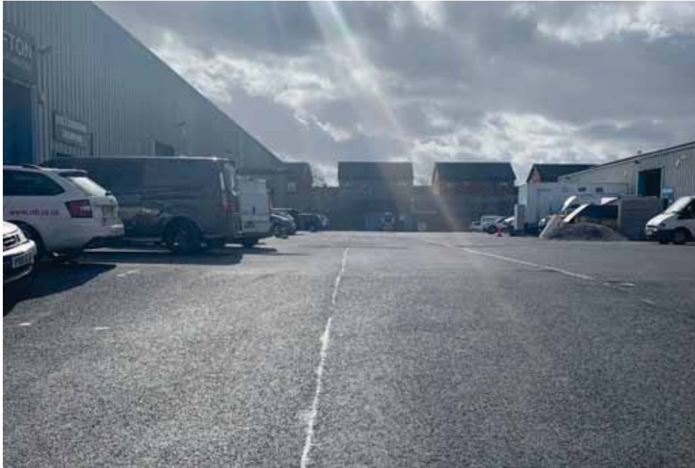
Photograph 9 View south-west across southern section of the development area.
