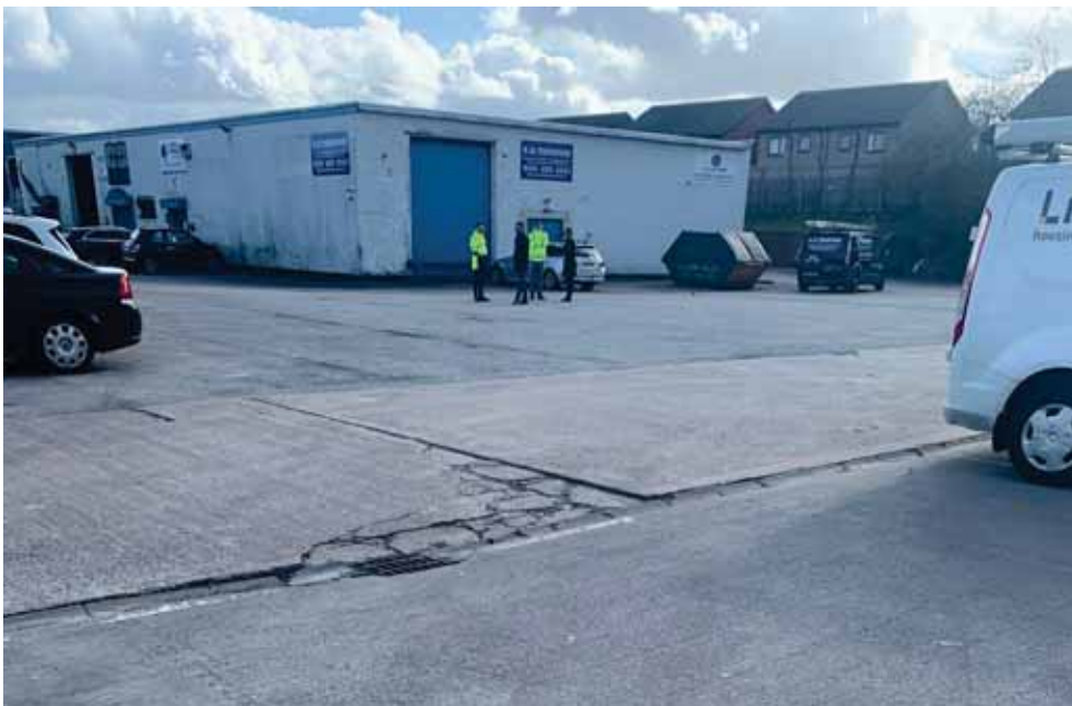
Photograph 6 Single-storey steel frames structure close to the south-western site boundary.
