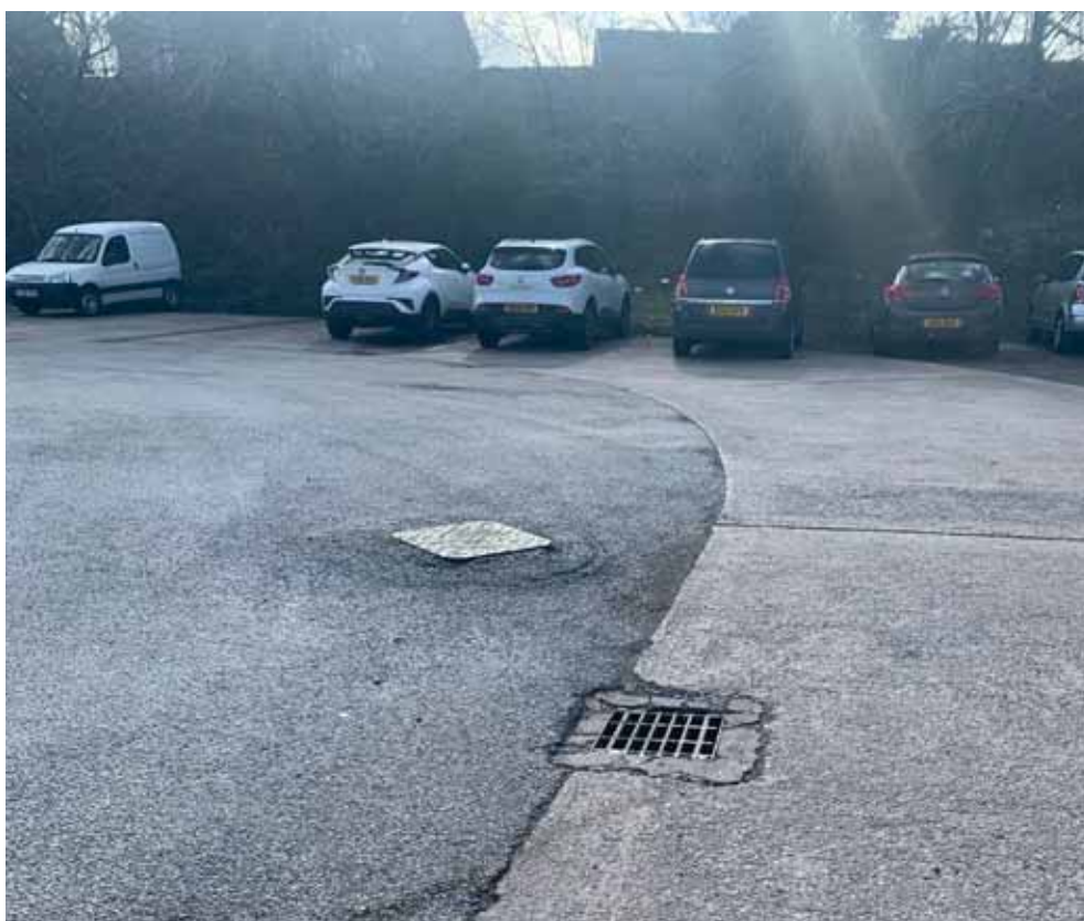
Photograph 4 Mixed concrete and asphalt hardstanding in the western site area.
