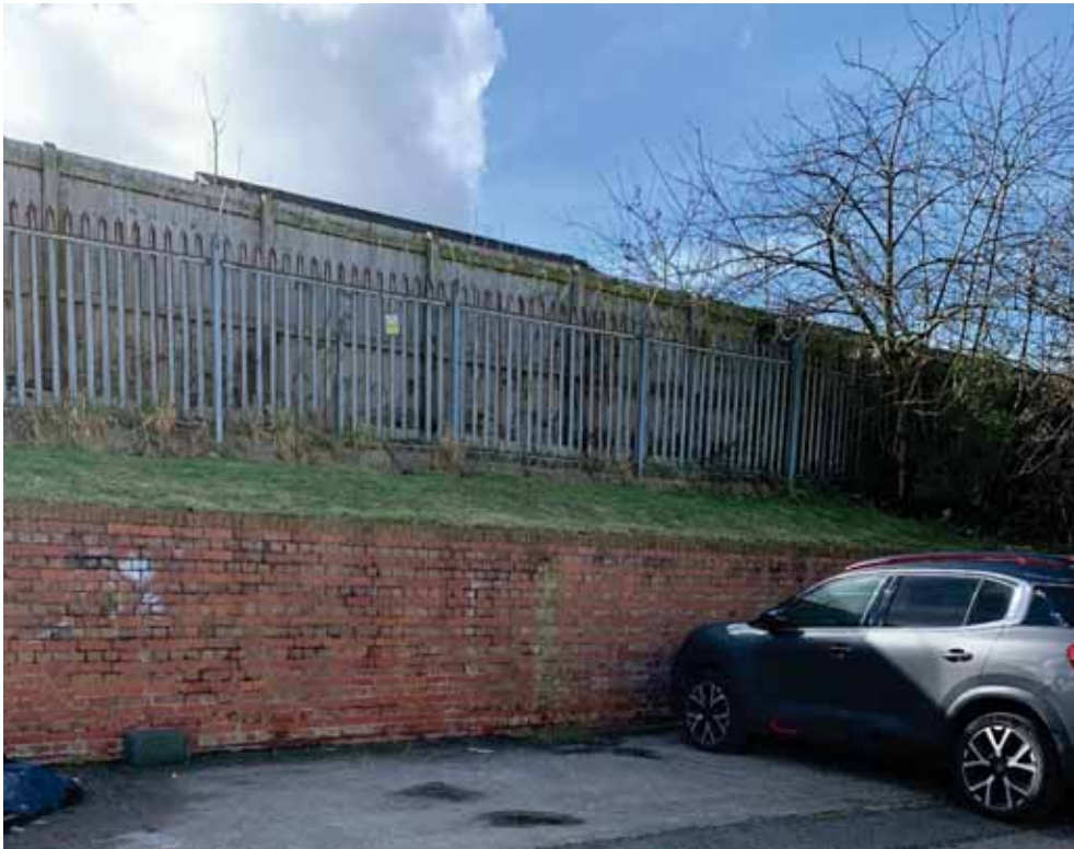
Photograph 2 Typical section of brick retaining wall to the south-western site boundary.
