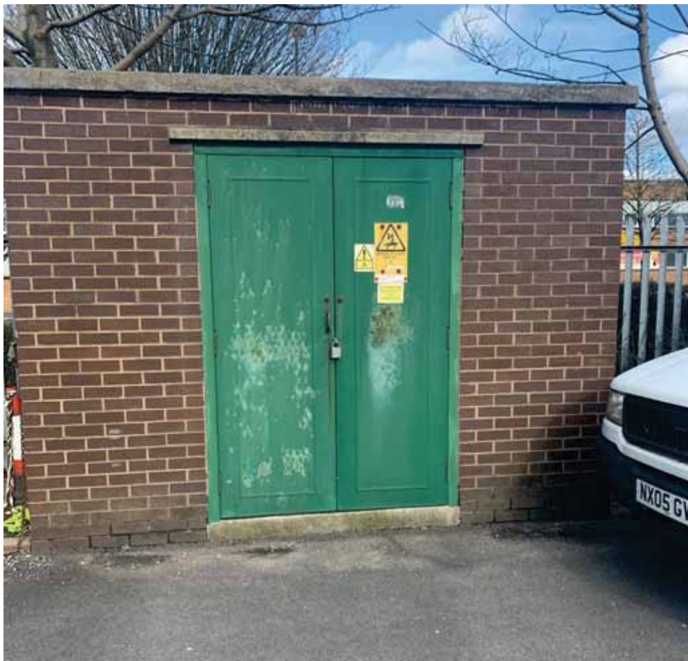
Photograph 10 Smaller of the two electricity sub-stations close to the gas governor on the north-eastern site boundary with Wilson Road.
