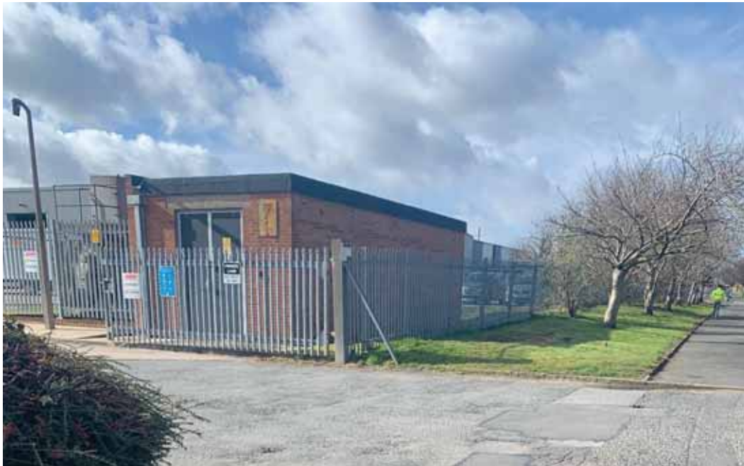
Photograph 7 Larger of the two electricity sub-stations, adjacent to Wilson Road at the north-eastern site boundary.
