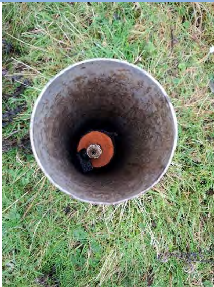
Photograph 9: Previous gas monitoring well
