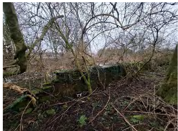
Photograph 6: 3ft high brick wall
