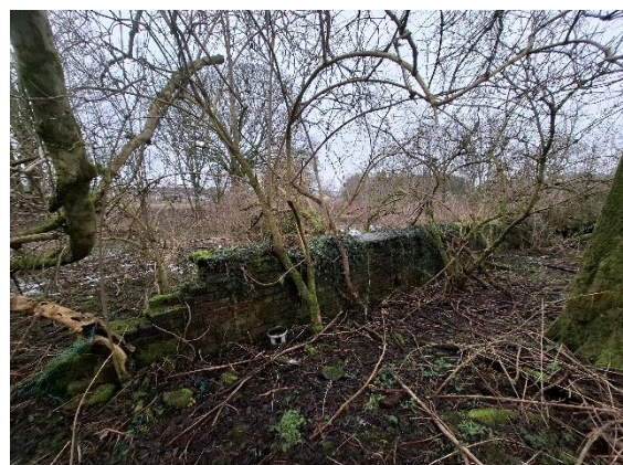
Photograph 6: 3ft high brick wall
