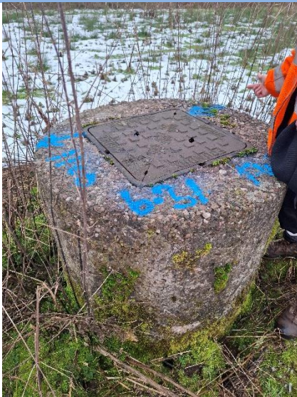
Photograph 3: Above ground manhole
