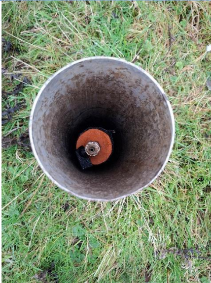
Photograph 9: Previous gas monitoring well
