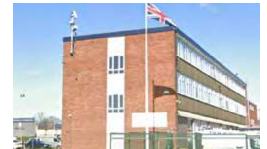
Vertical banding between windows
