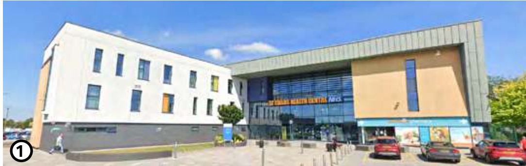
① St. Chads NHS Health Centre
