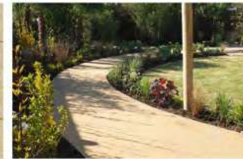
PATHS Resin bonded gravel to paths
