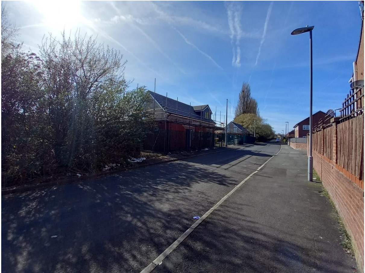
ADJACENT SITE FORMER OFFICES BEING CONVERTED TO DWELLINGS
