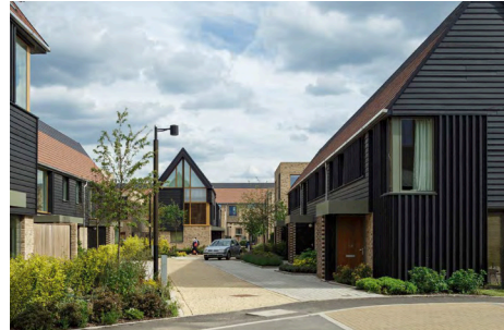
① Timber to First Floor Accommodation
