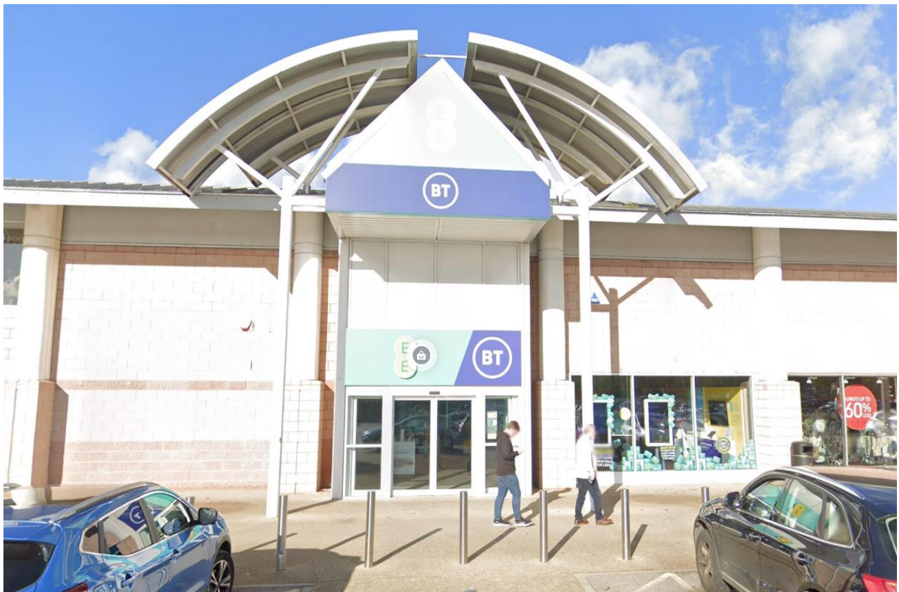
Photo above shown the front elevation of the property, with previous tenants signage
