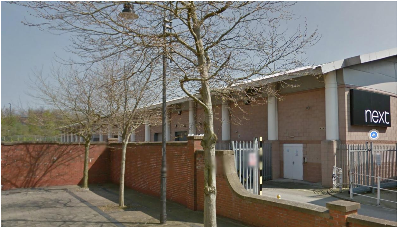
Image above shows the rear of the building. The AC will be well out of sight with the service area.
