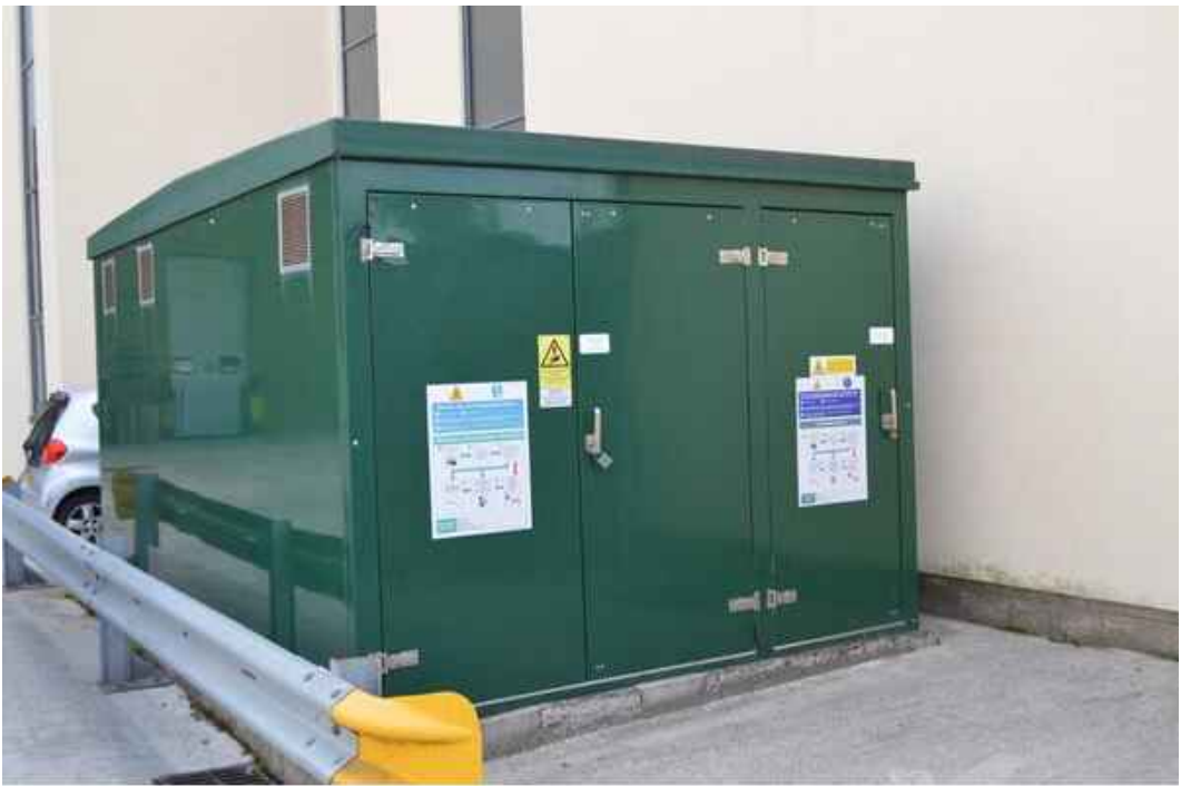
Extract C: Typical GRP Housing Gas Kiosk: 2m x 1.5m (Sizes TBC by specialist)
