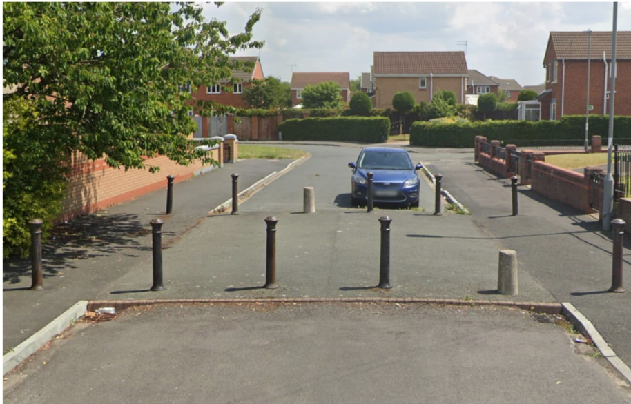
Figure 2-5 - Bollards on Roseheath Drive
