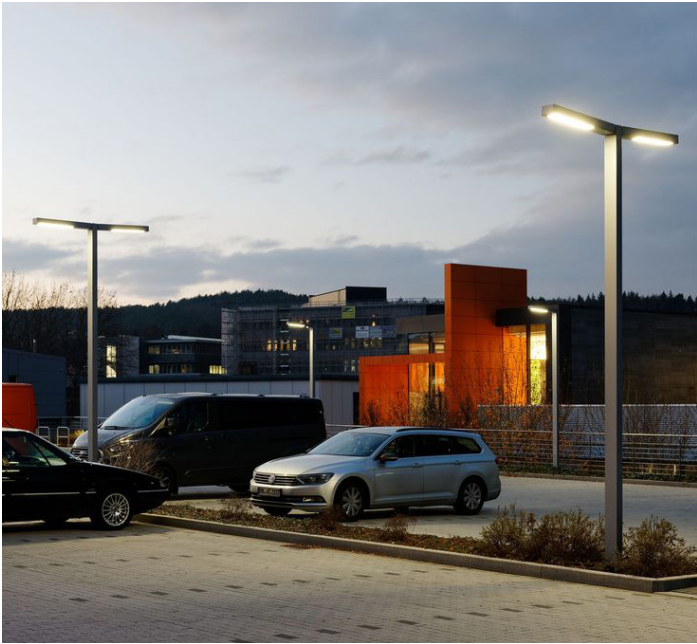
Utilising multi-head lighting columns for car park
