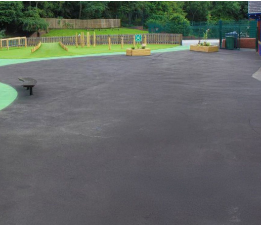
Bitmac surfacing to footways in car park and sports pitch footway areas
