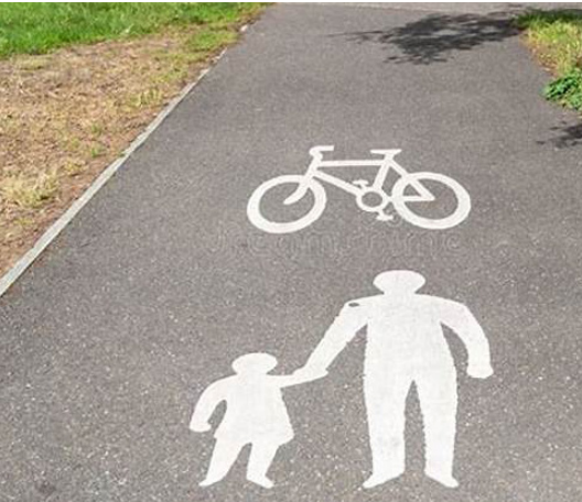
Bitmac surfacing to Shared Use route with thermoplastic marking where required for LTN 1:20
