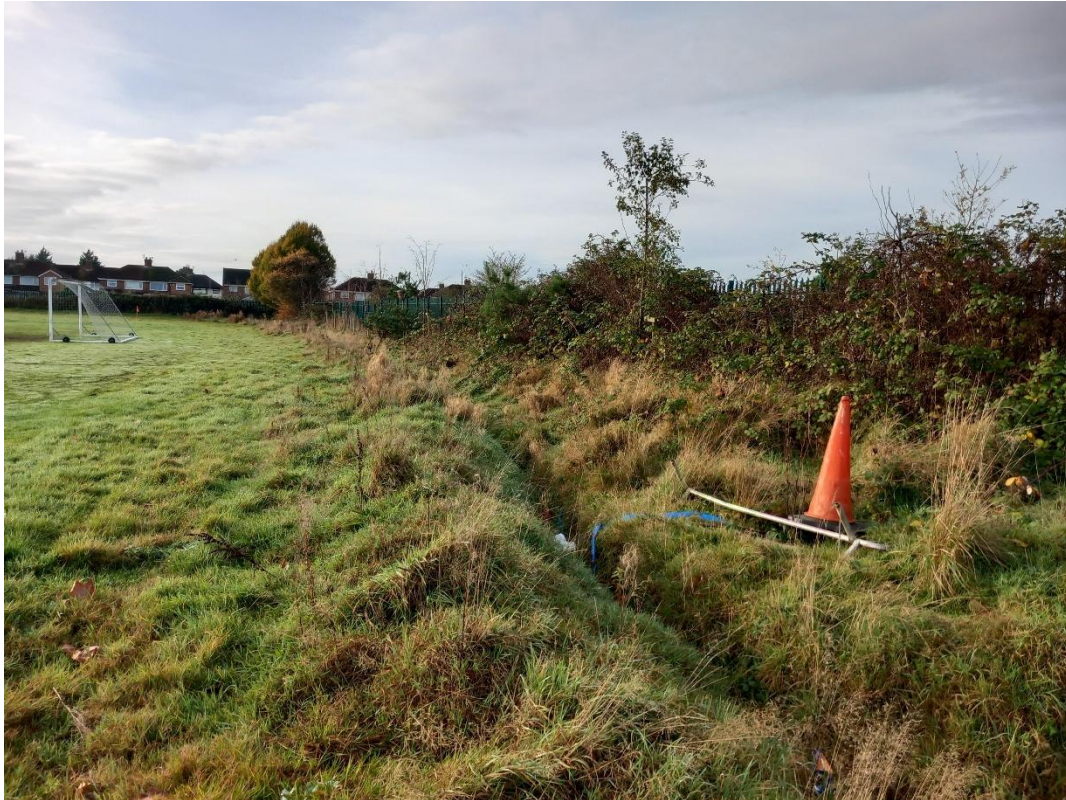
Photo 5: Existing drainage ditch
