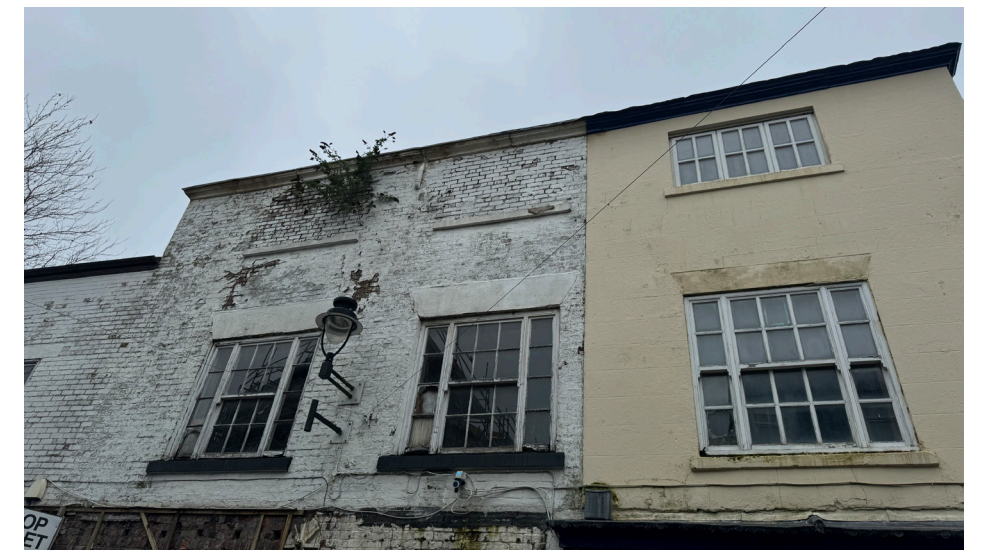
08. View of existing buildings condition
