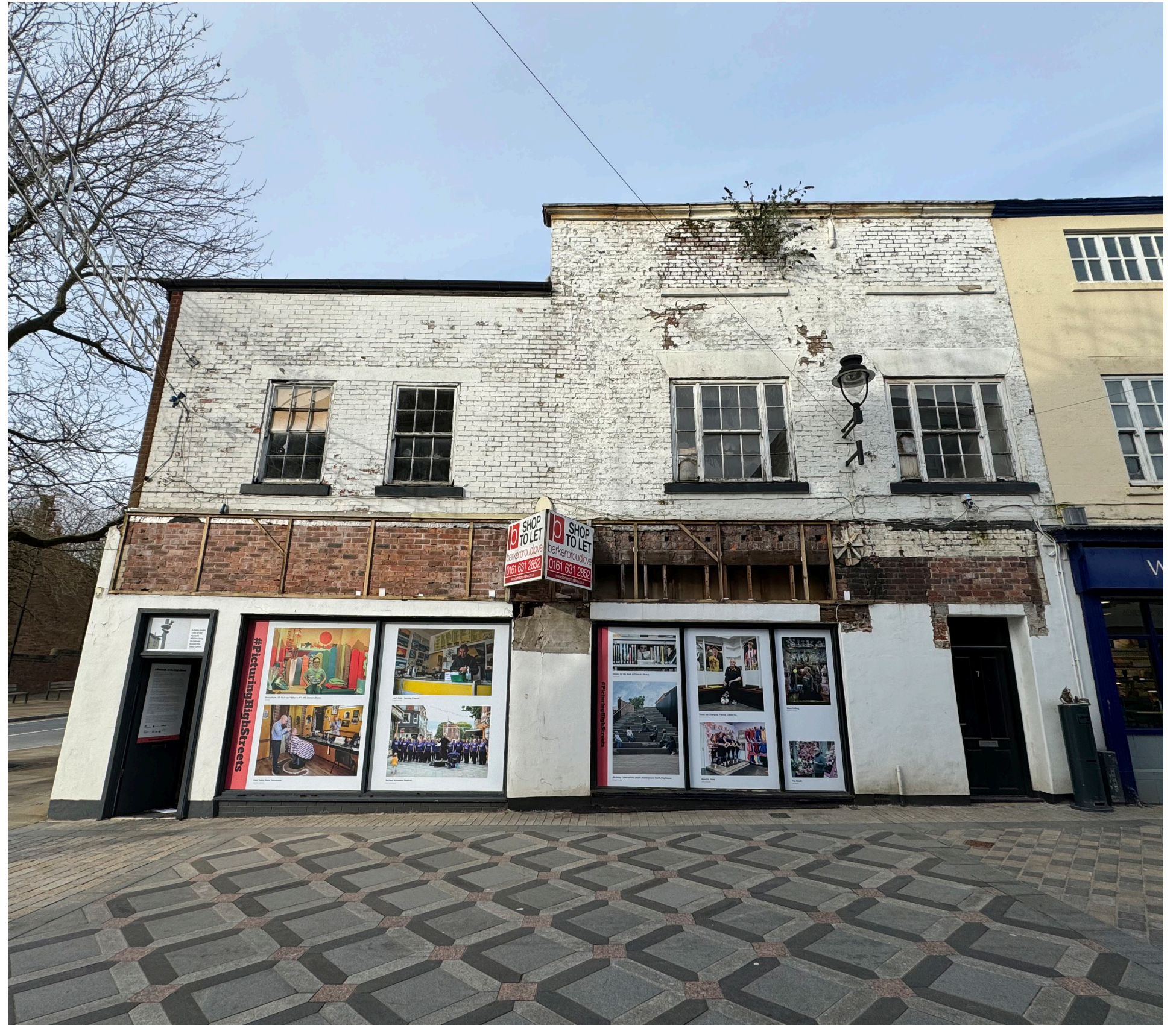
01. Photograph of existing building on site
