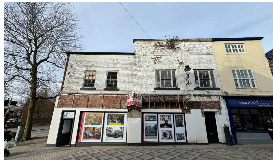
07. View of existing building on site
