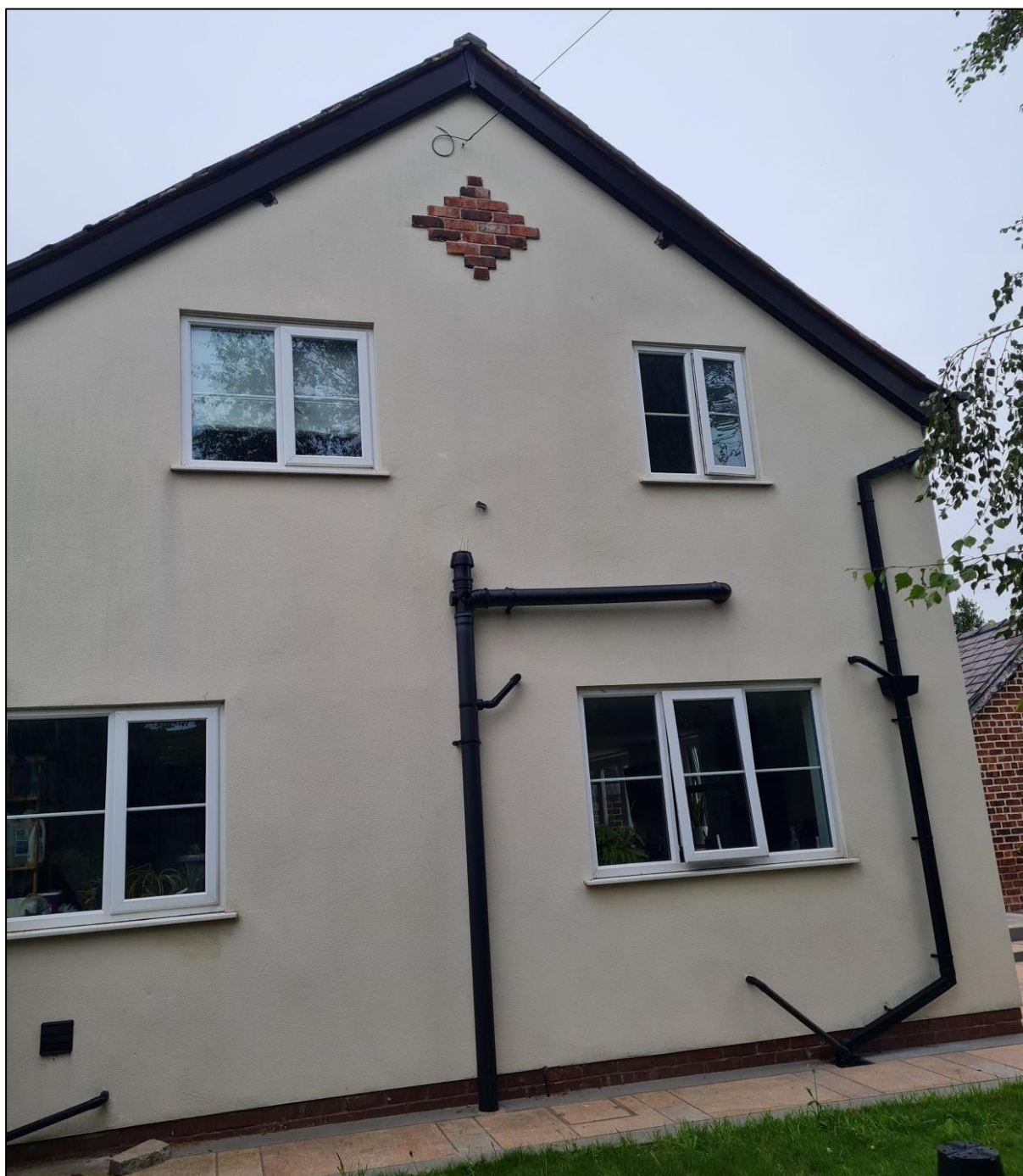
Plate 3 – Southeastern elevation of the building
