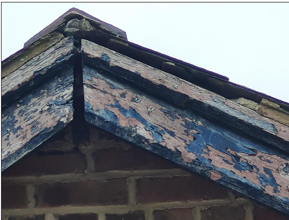
Plate 7 – Gap beneath roof tiles at wall plate of outbuilding
