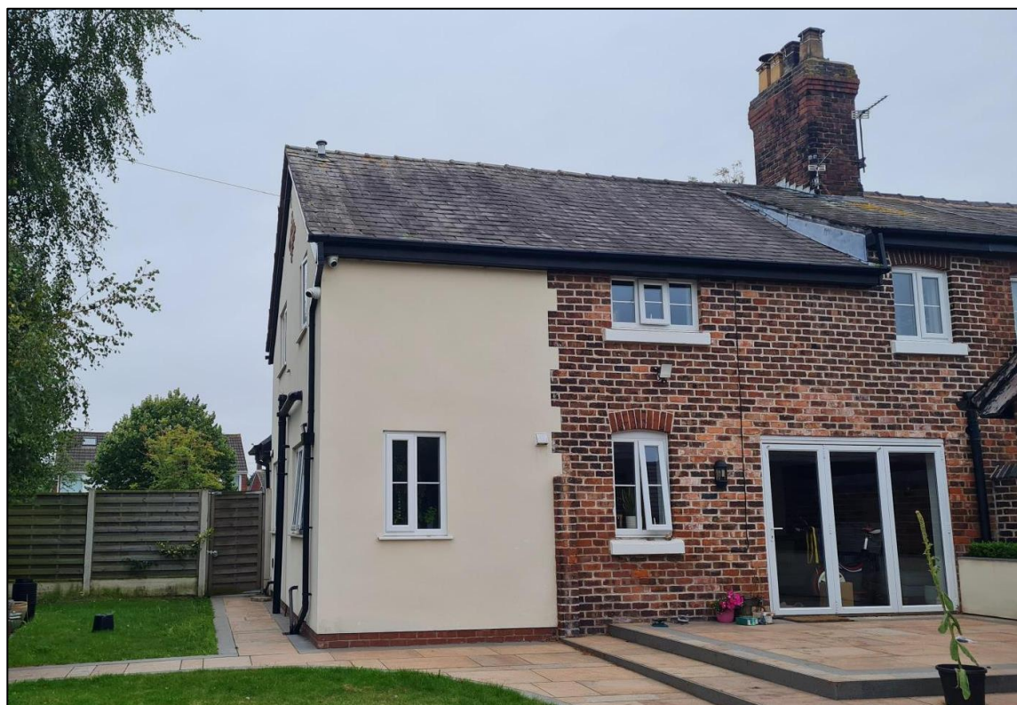
Plate 2 – Rear elevation of the building
