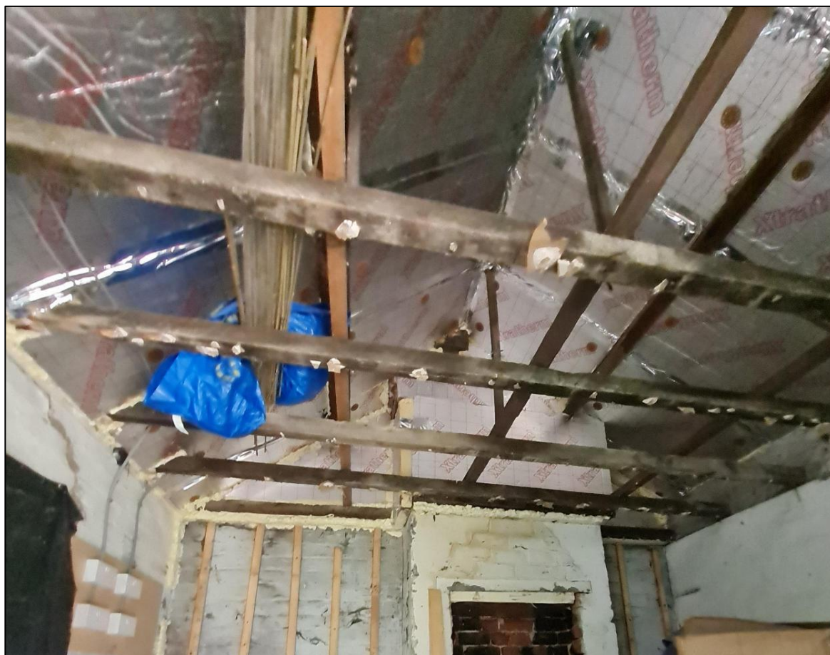
Plate 9 – Interior of western portion of outbuilding
