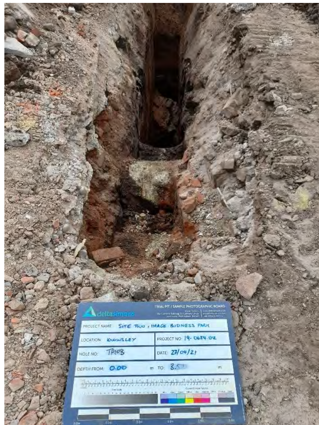
Photograph 6 – TP103 Trial Pit 0.0 to 3.5 m.
