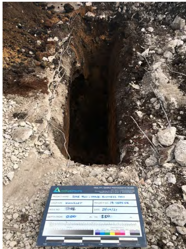
Photograph 4 – TP102 Trial Pit 0.0 to 3.5 m.
