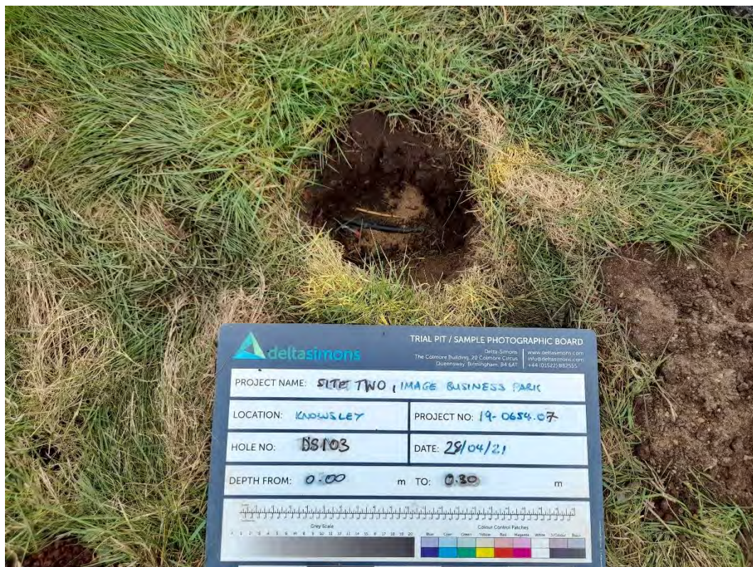
Photograph 18 – DS103 hand dig hole with services. Location was abandoned.
