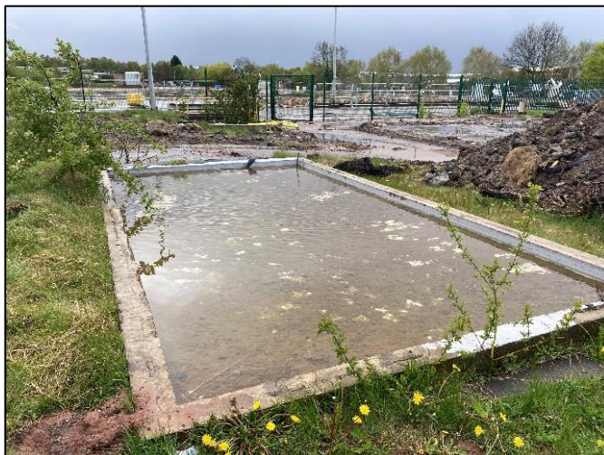
Photograph 6: Concrete basin filled with standing rain water in footprint of Building 30
