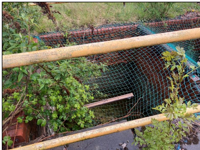
Photograph 5: Brick-lined pits present within the south of the Site
