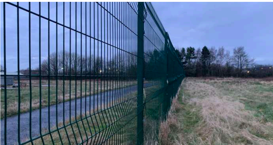
1. View north along eastern boundary
