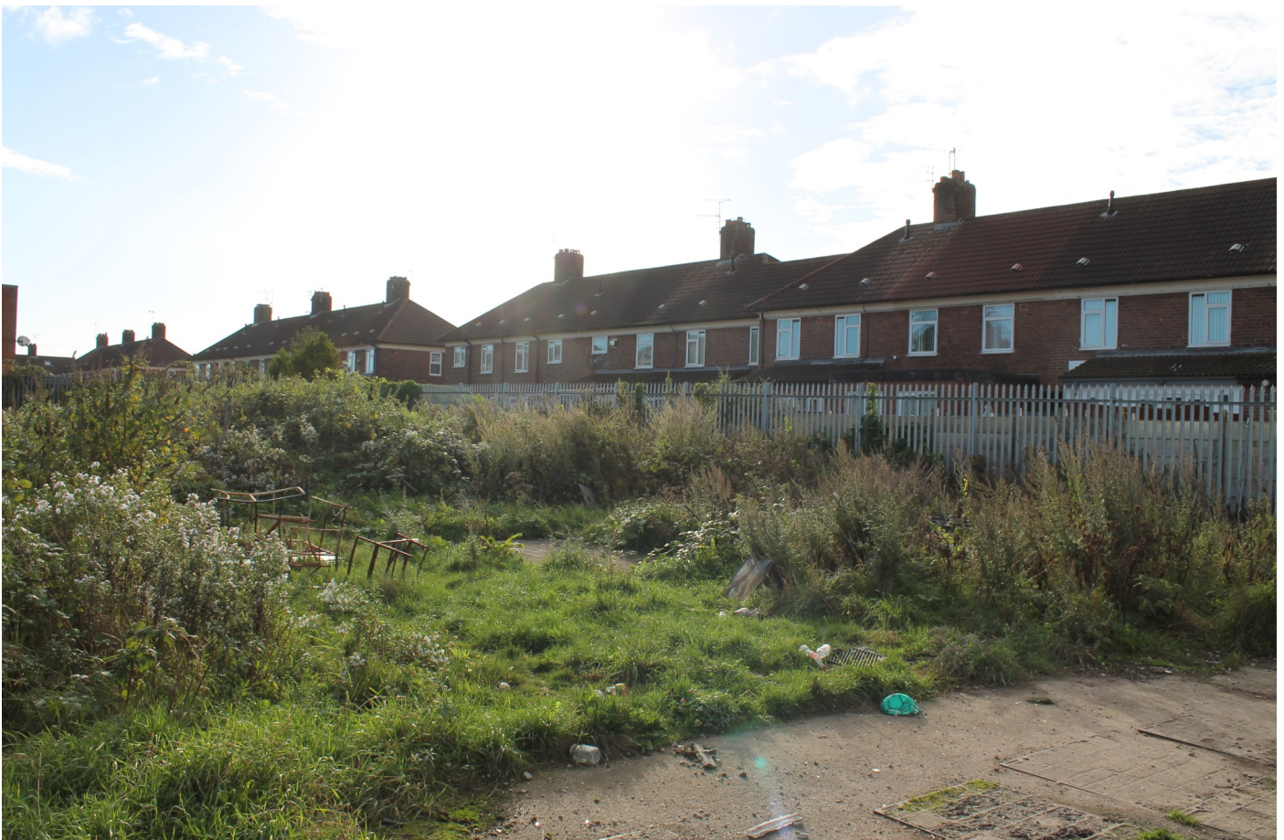
Figure 2.6: Rear of properties on Huyton House Road
