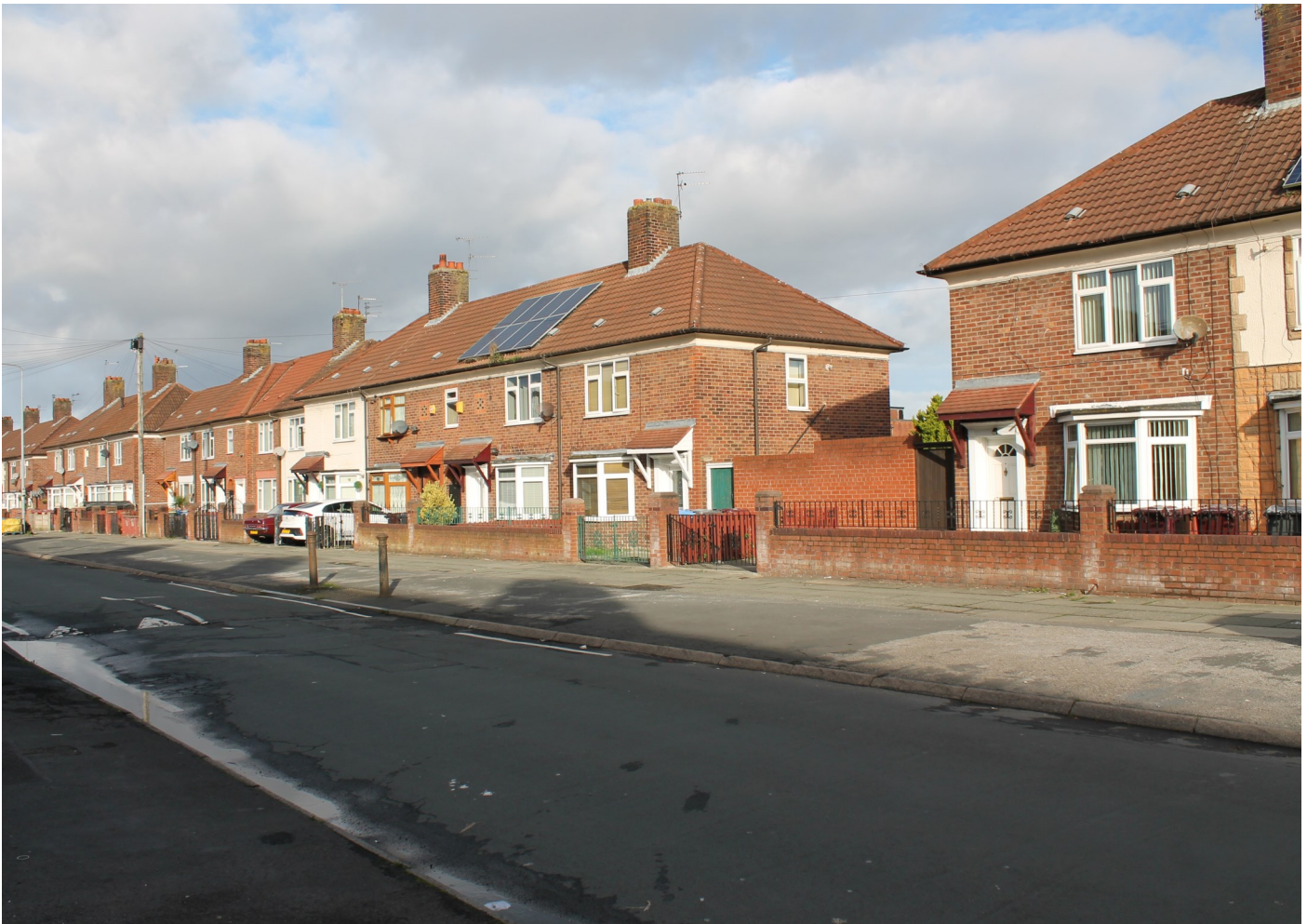
Figure 2.7: Front of properties on Huyton House Road
