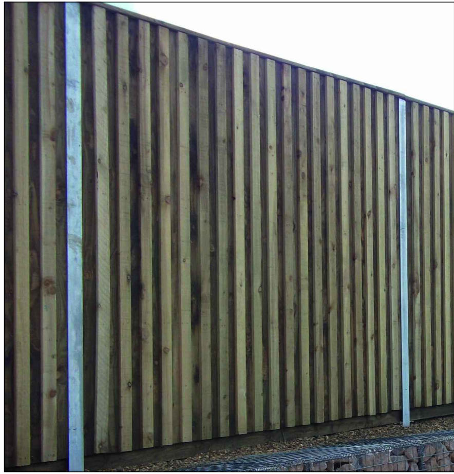
Acoustic Fencing 3.7m high acoustic timber fencing.
