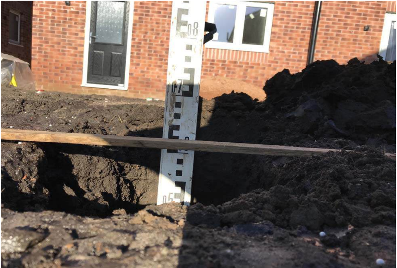
PLATE 7: Depth of soil cover in Plot No.71 (610mm)
