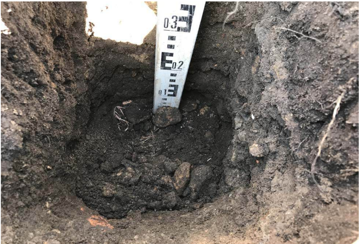
PLATE 6: Base of inspection pit in Plot No.79, showing membrane
