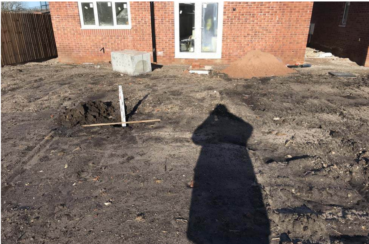
PLATE 4: Overview of inspection of Plot No.70
