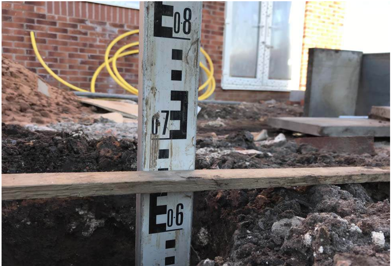
PLATE 9: Depth of soil cover in Plot No.72 (650mm)
