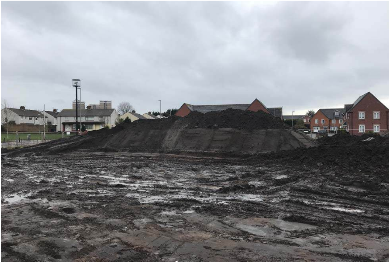
PLATE 1: Overview of larger topsoil stockpile in the southwest of Phase 1.
