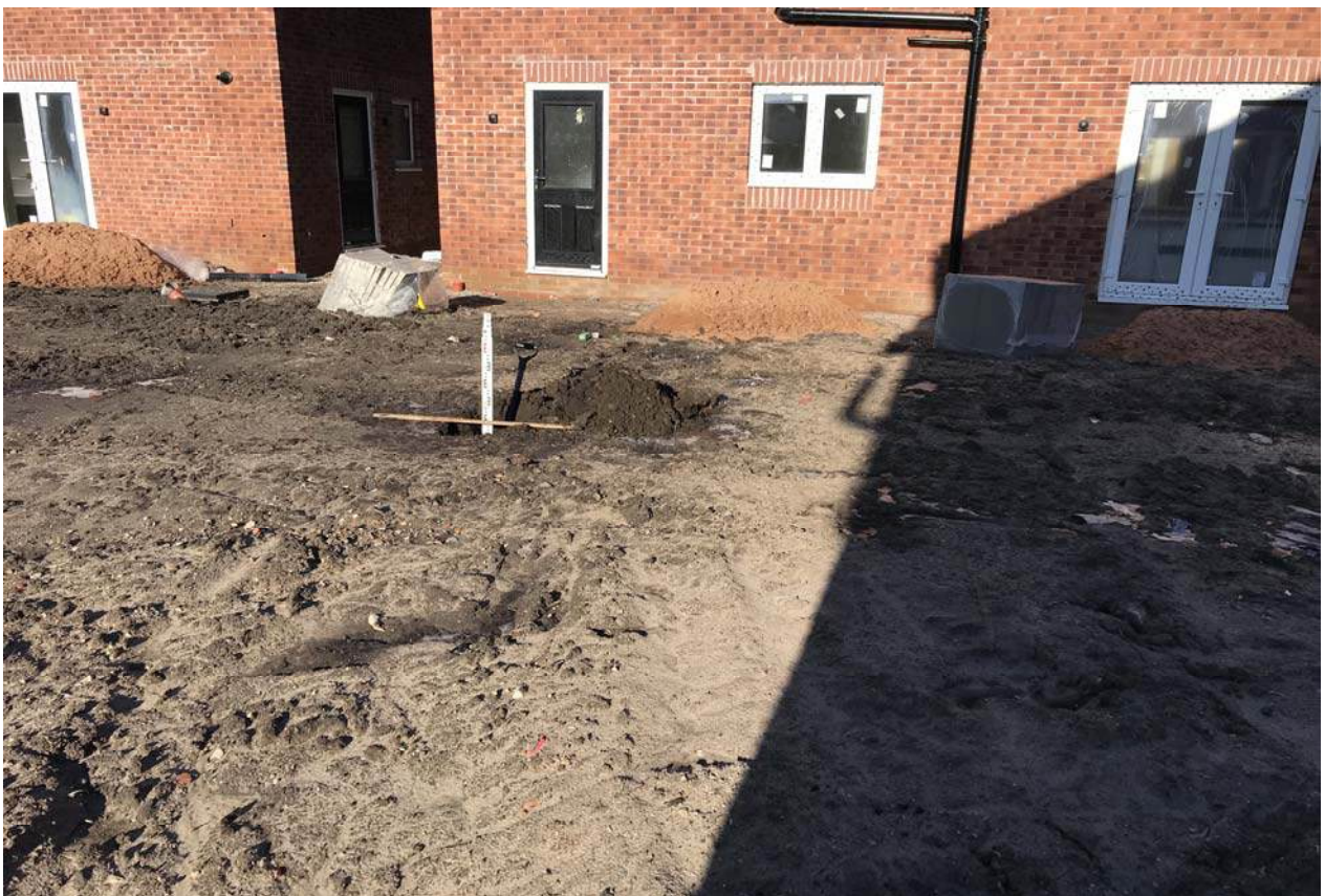
PLATE 6: Overview of inspection of Plot No.71
