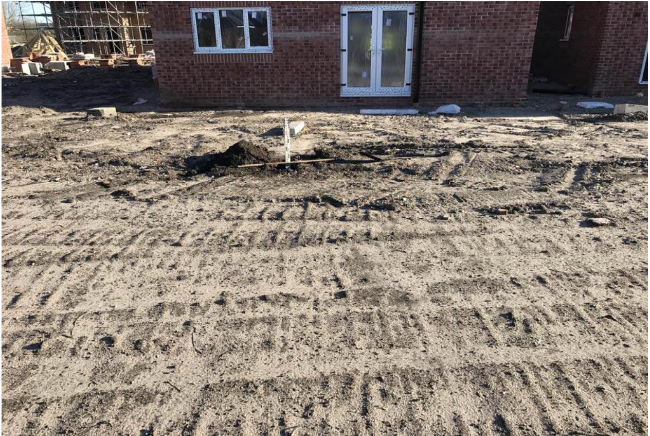
PLATE 1: Overview of inspection in Plot No.69
