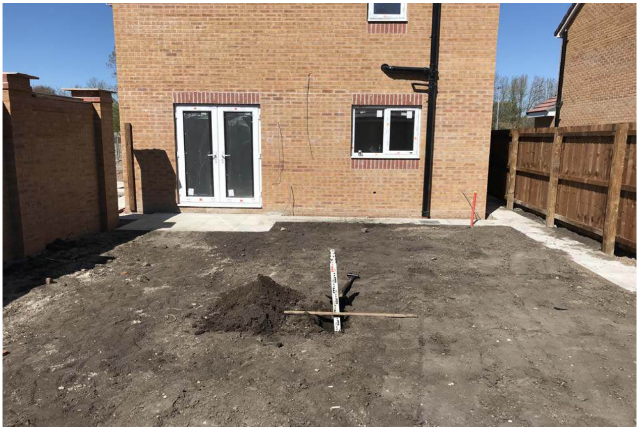
PLATE 4: Overview of inspection of Plot No.79
