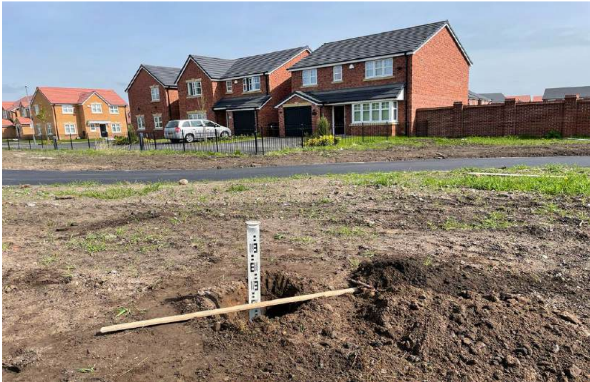
PLATE 1 – Inspection Pit IP1 in area of designated public open space (facing plot No.70) @ May 2022.
