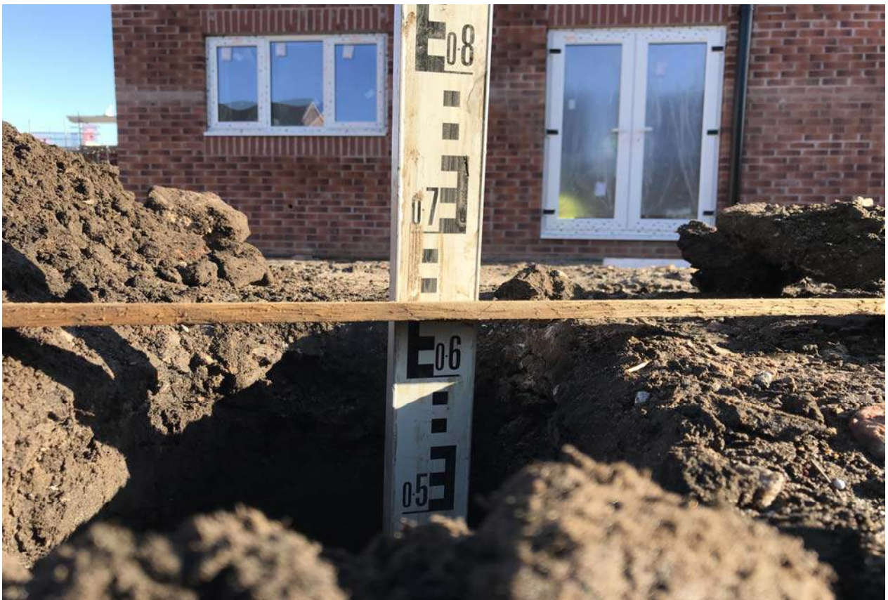
PLATE 2: Depth of soil cover in Plot No.69 (640mm)
