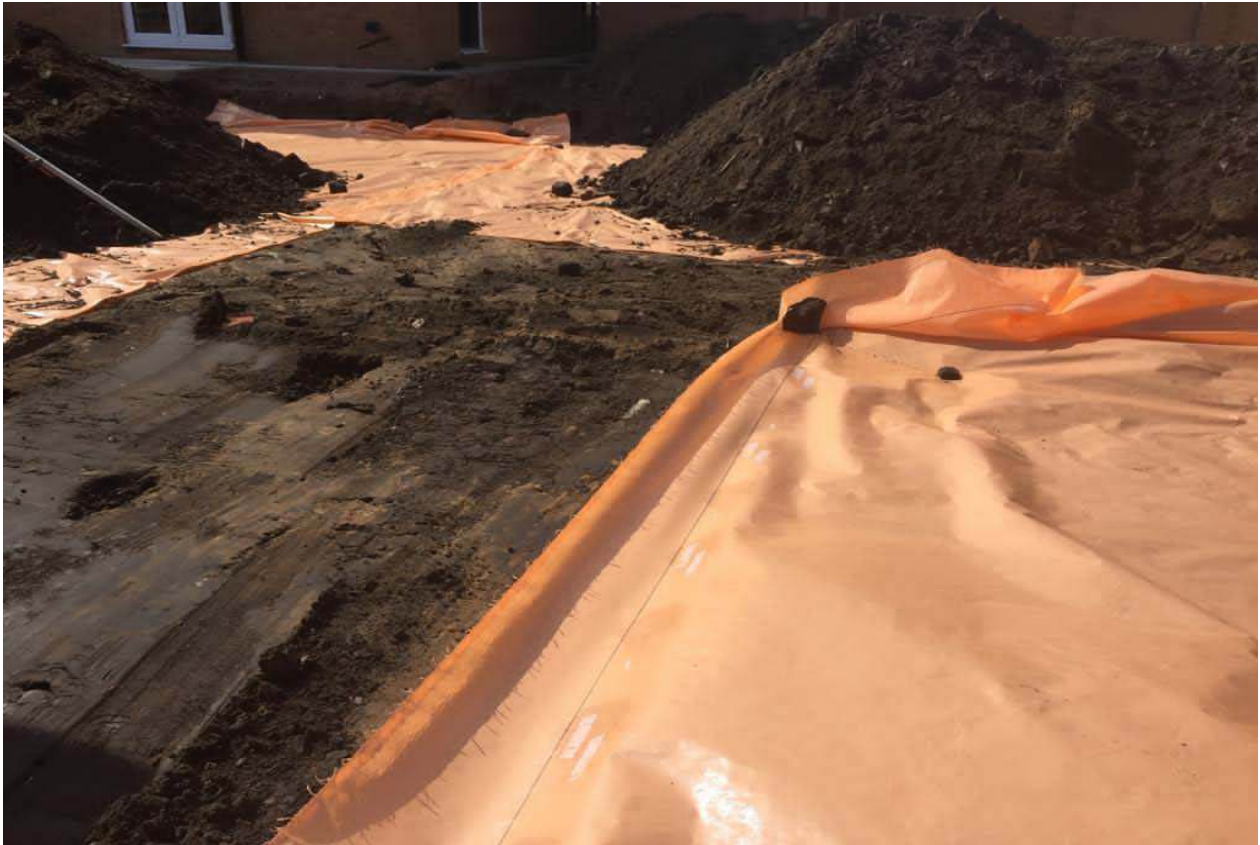
PLATE 1: Placement of membrane beneath Plots 78, 80 and 81
