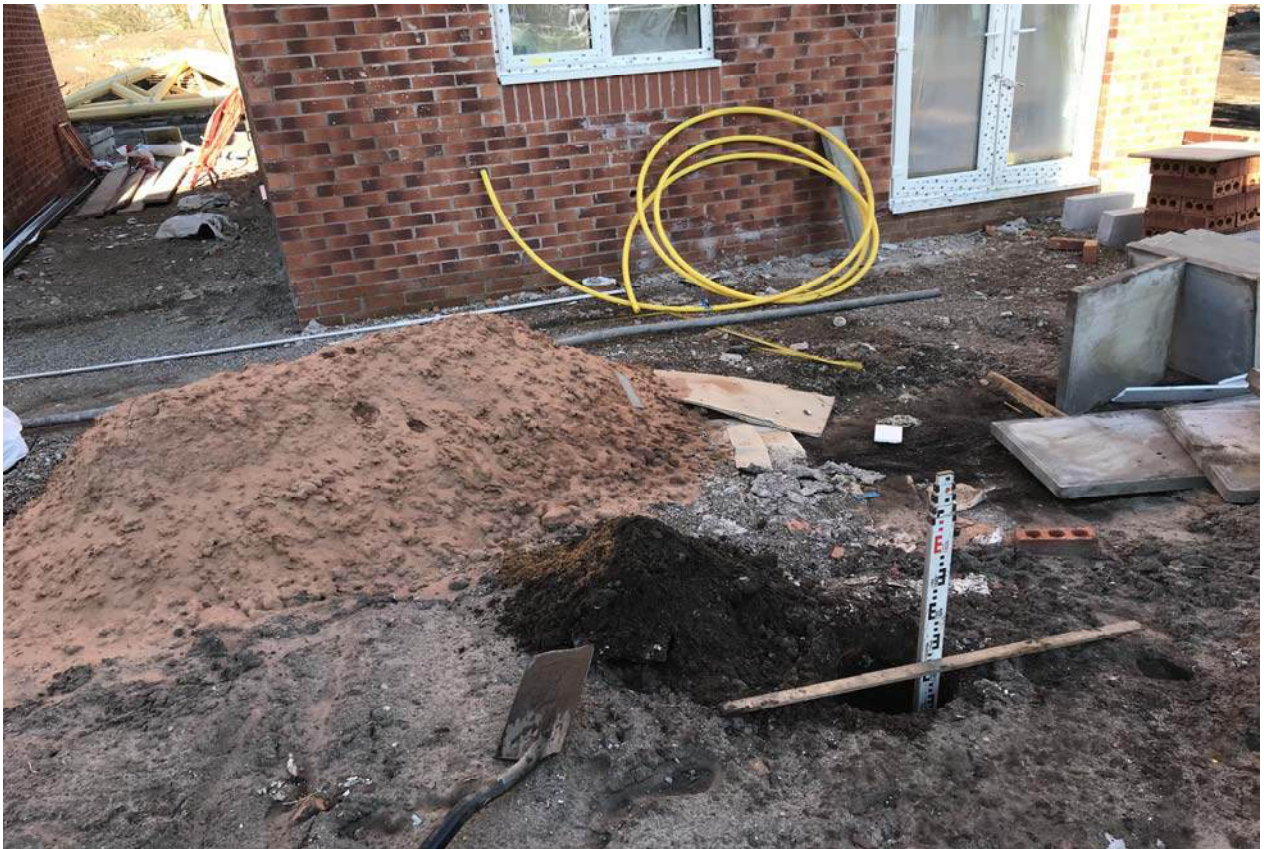
PLATE 8: Overview of inspection in Plot No.72
