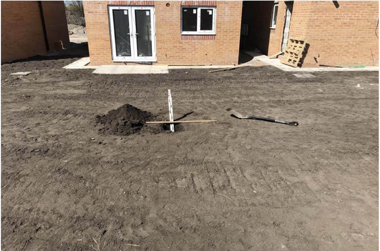
PLATE 9: Overview of inspection in Plot No.81
