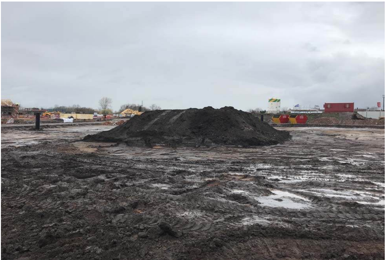
PLATE 2: View of smaller topsoil stockpile near Plots 153-154.
