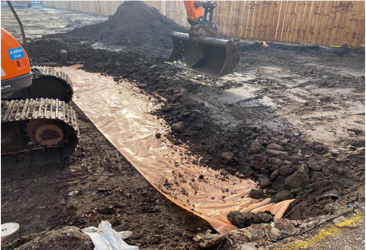
PLATE 3: Placement of membrane beneath soil cover in Plot No.70
