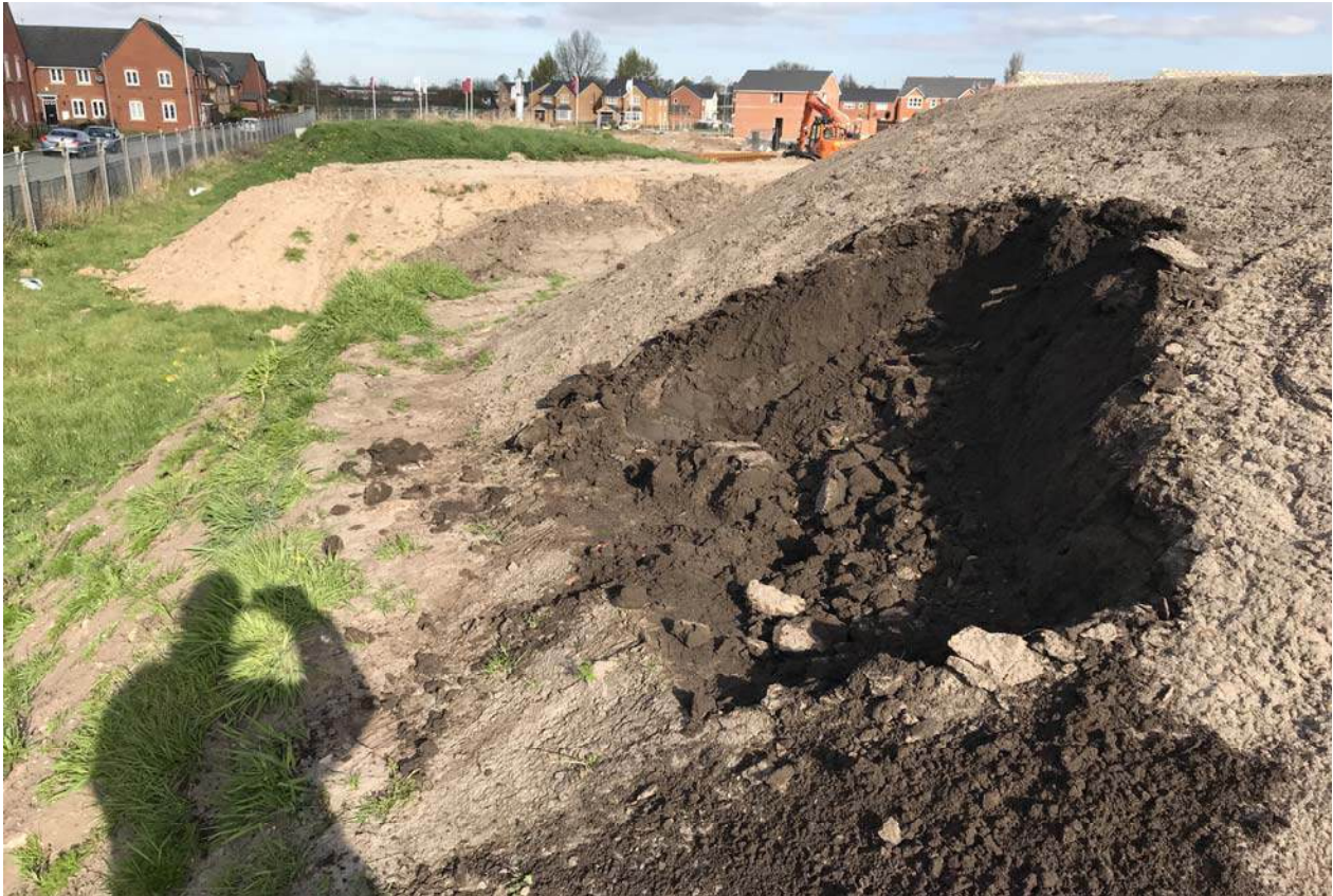
PLATE 3: Overview of validation area following removal of asbestos impacted soils.
