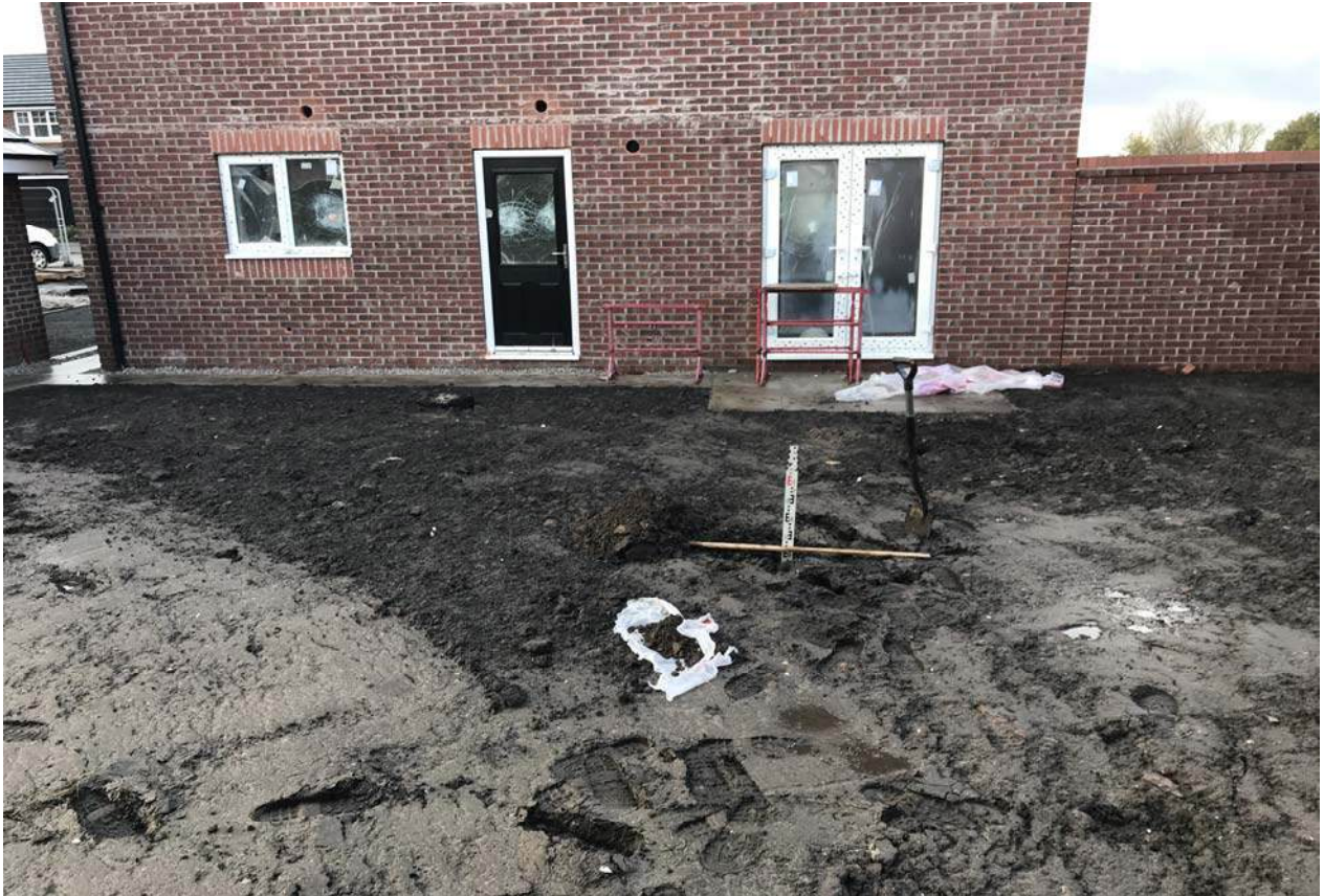
PLATE 1: Overview of inspection in Plot No.54
