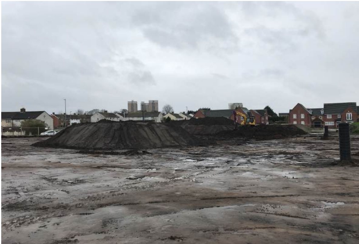
PLATE 3: Topsoil stripped from the southern half of Phase 1.
