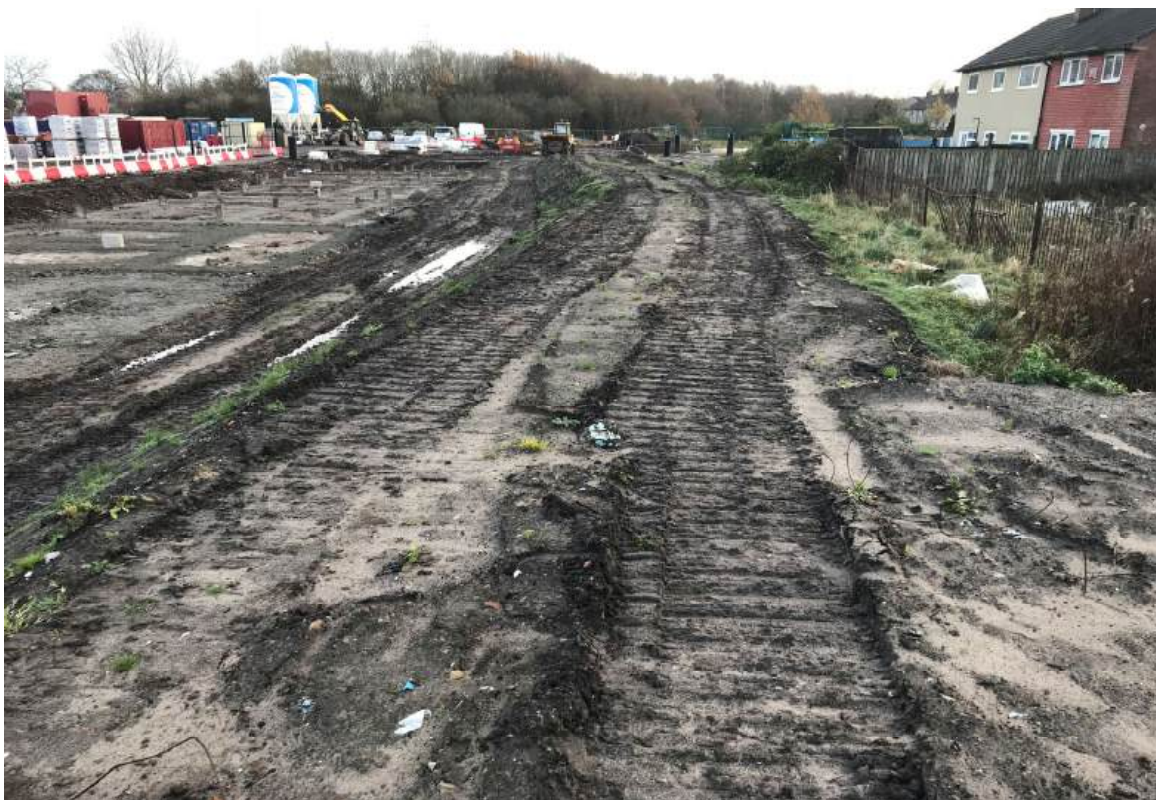
PLATE 11: Topsoil stockpile along southern edge of Phase 4.
