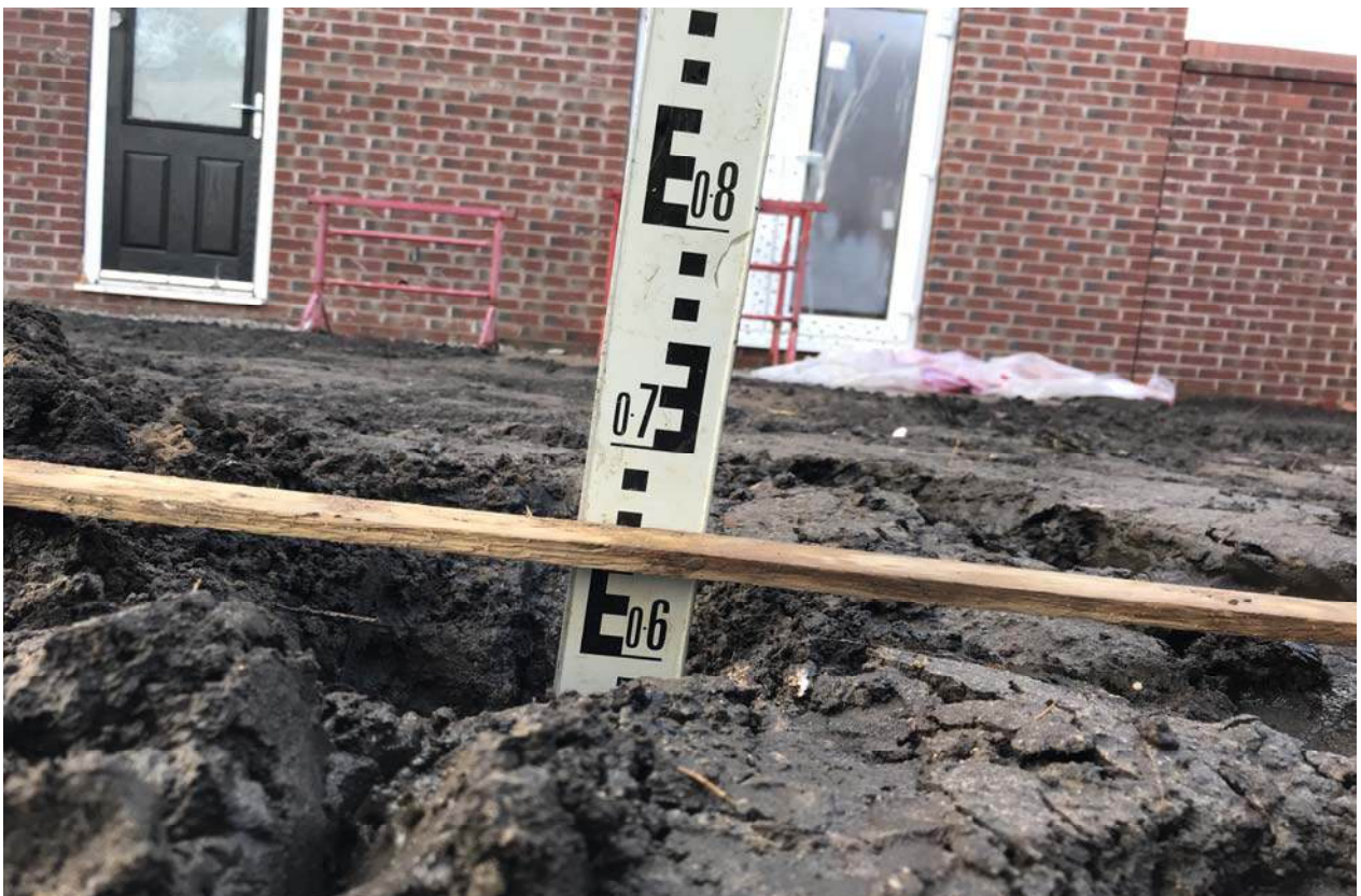
PLATE 2: Depth of soil cover in Plot No.54 (>650mm)
