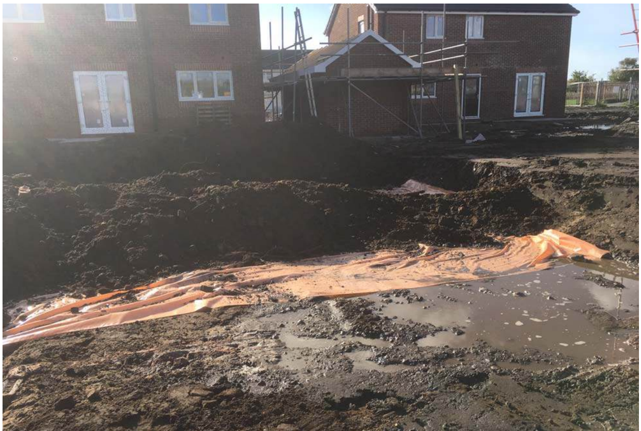
PLATE 6: Placement of membrane beneath clean soil cover in Plot No.55
