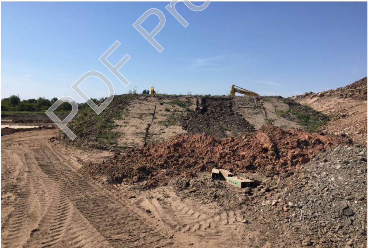
PLATE 2: View of smaller topsoil stockpile above Plots 36-38.
