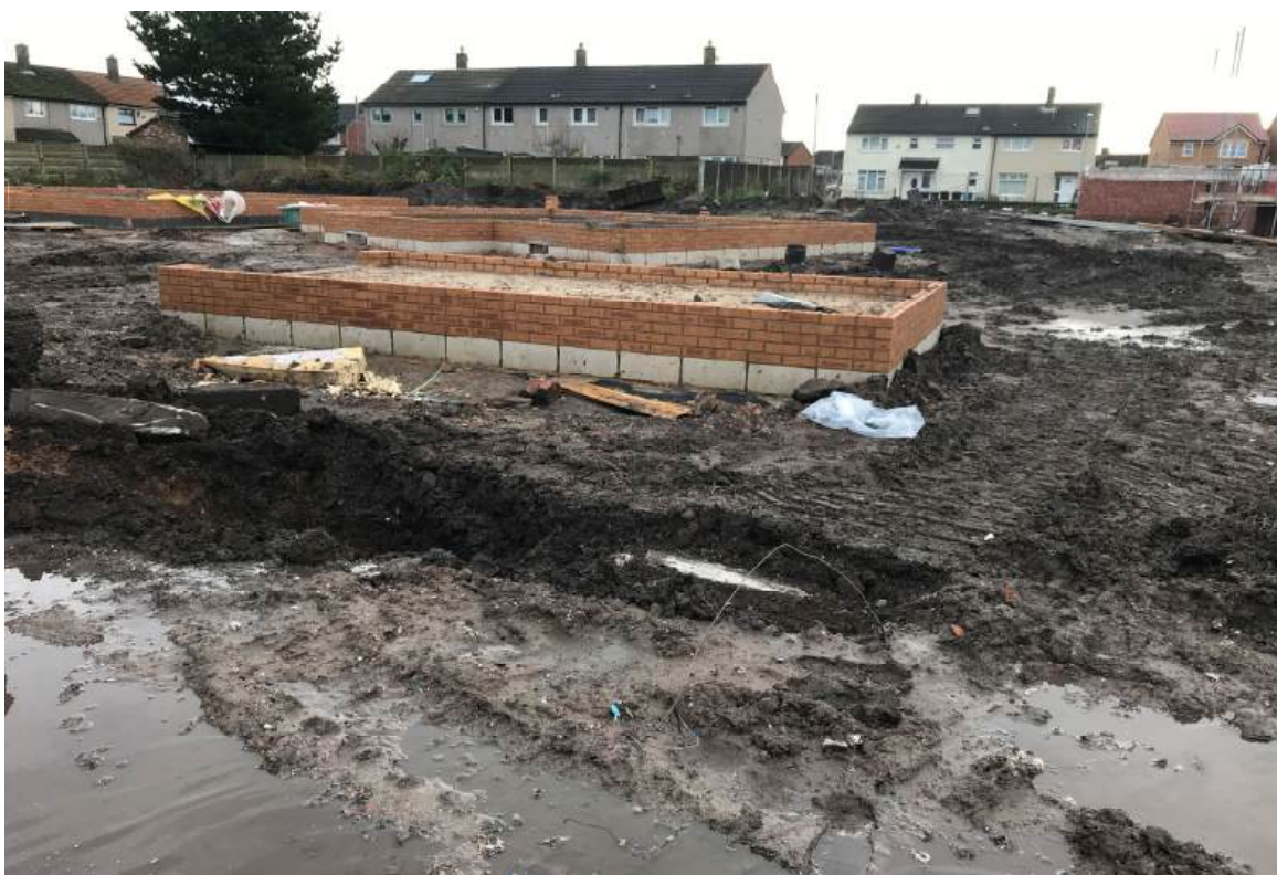
PLATE 12: Exposed surface at location of former Electricity Sub Station (near Plot 83).
