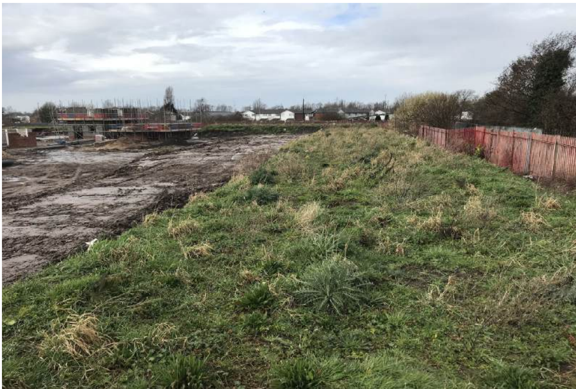
PLATE 4: Topsoil stripped from the Phase 2 area.
