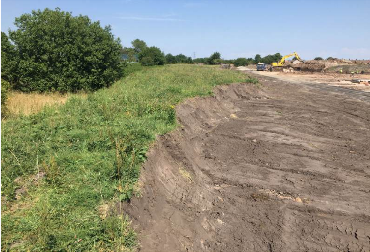
PLATE 1: Topsoil stripped from the northern part of Phase 1.
