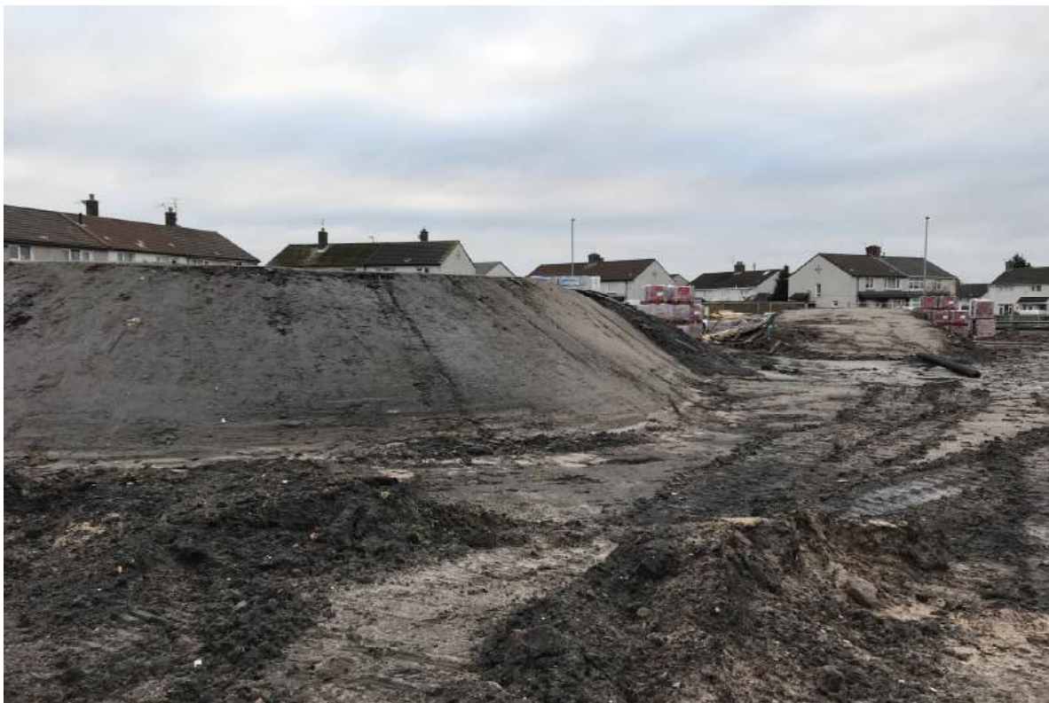
PLATE 8: Topsoil stripped from the Phase 3 area.
