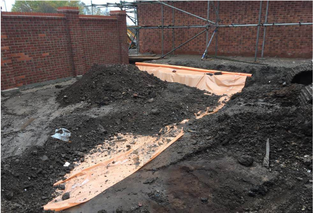
PLATE 3: Placement of membrane beneath clean soil cover in Plot No.54
