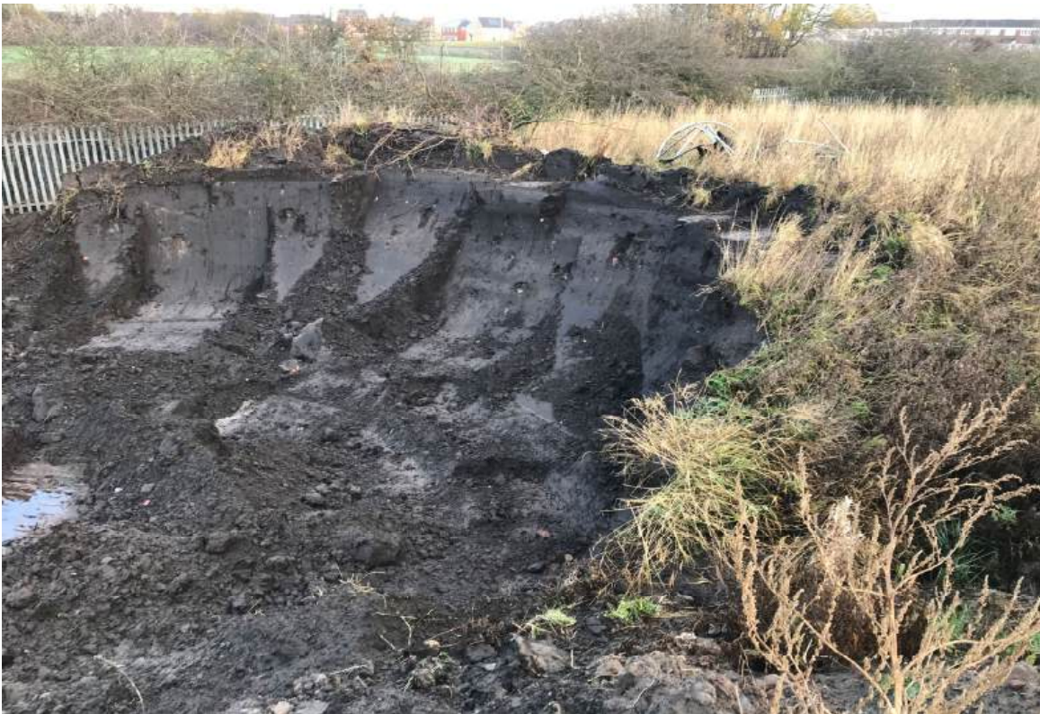
PLATE 10: Cross-section through the large Phase 4 topsoil stockpile.
