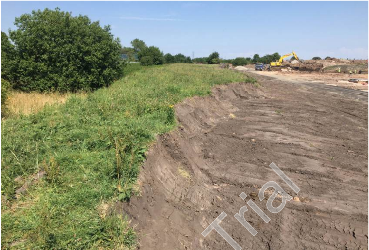
PLATE 1: Overview of larger elongate topsoil stockpile in the northwest.
