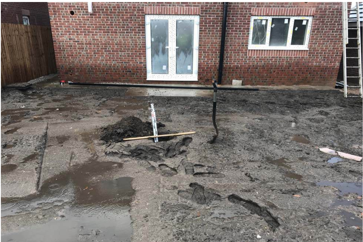
PLATE 4: Overview of inspection of Plot No.55
