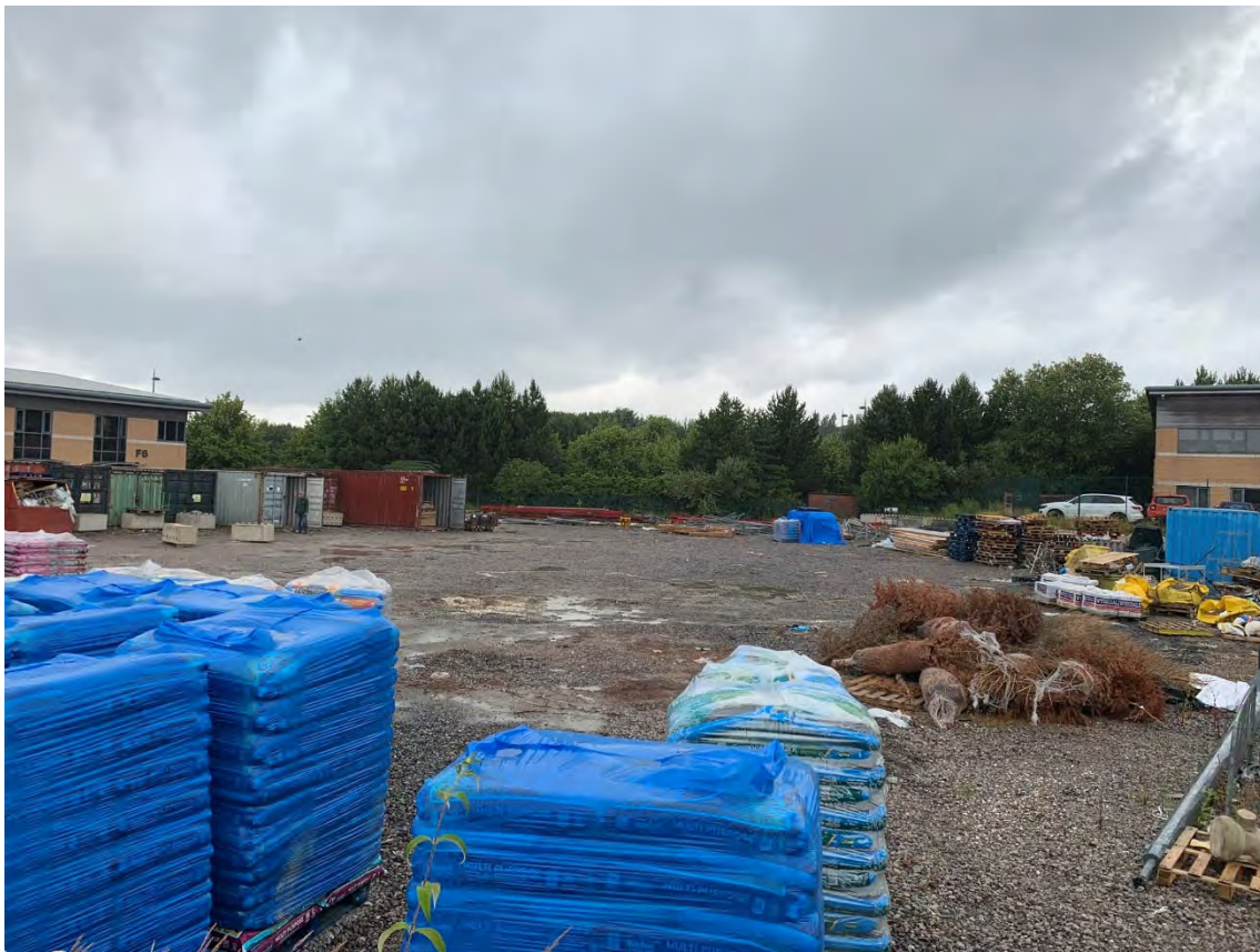
Existing storage yard – artificial unvegetated, unsealed surface..
