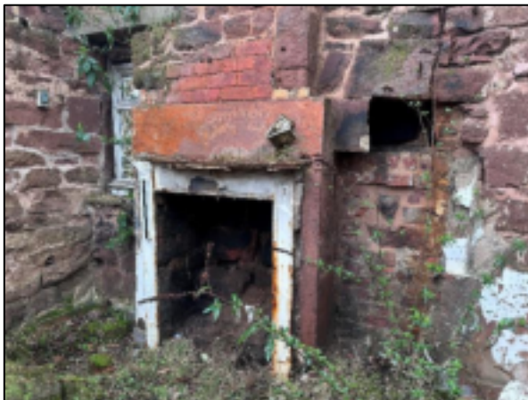
Figure 27: The old fireplace present inside the building.
