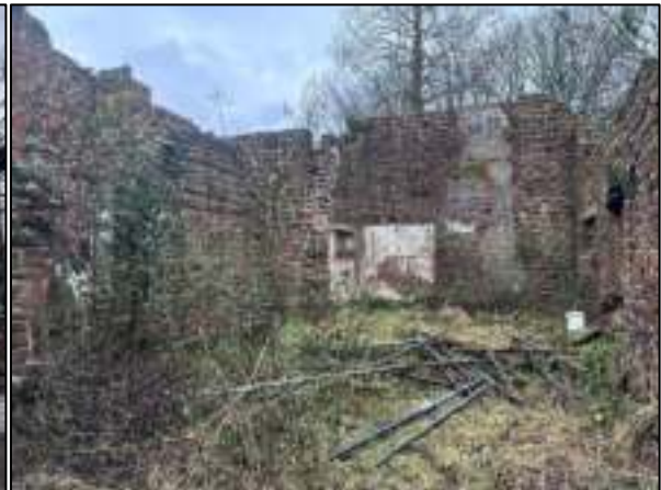
Figure 24: The interior of building B2.
