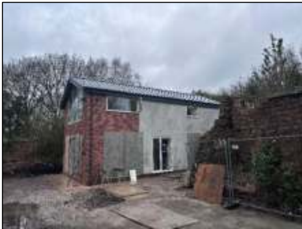
Figure 13: The more modern building on the site.
