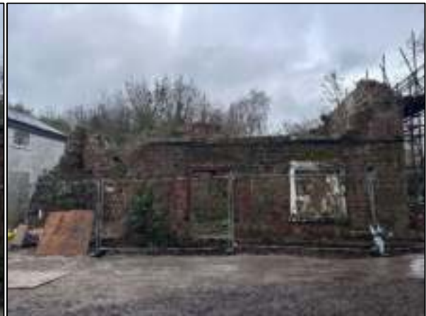
Figure 14: The ruined building.
