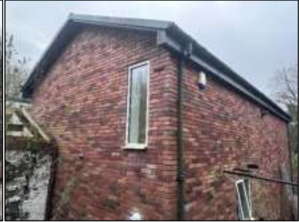
Figure 22: Building B1, viewed from the north.
