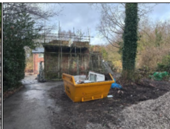
Figure 12: Bare ground to the east of the buildings.
