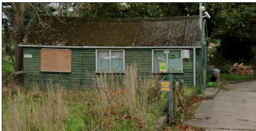
Photo 5. Image of building 12 within the Site, looking east
