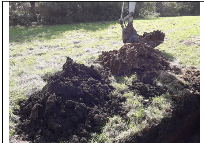
Trial Pit 143 Spoil
