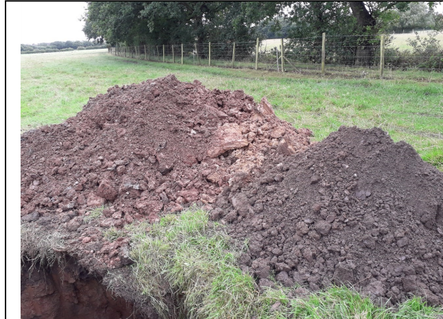
Trial Pit 132 Spoil
