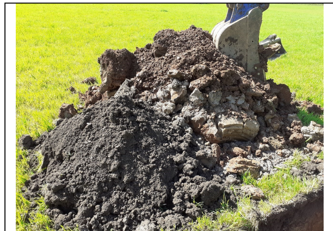
Trial Pit 114 Spoil
