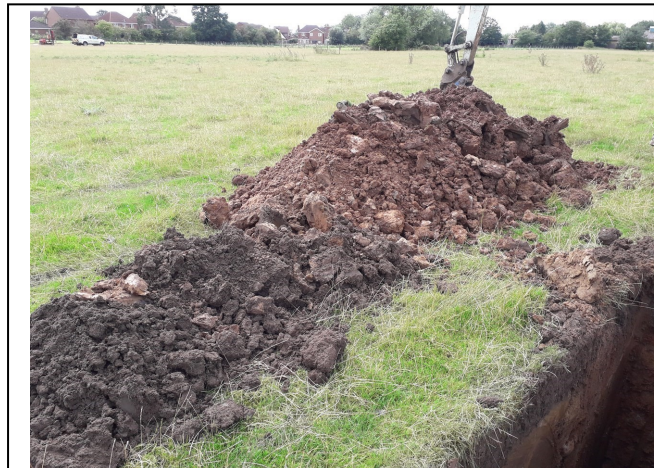
Trial Pit 138 Spoil
