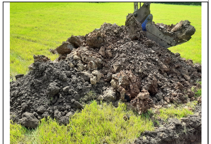
Trial Pit 113 Spoil
