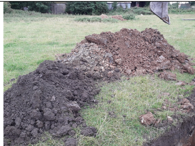
Trial Pit 135 Spoil
