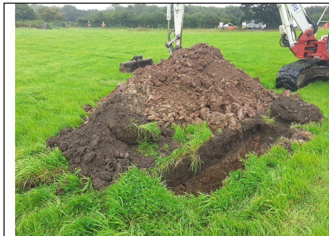
Trial Pit 122 Spoil
