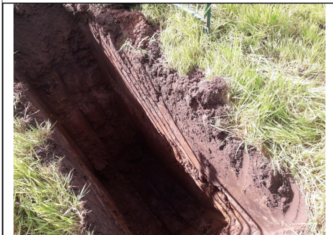
Trial Pit 104/ Soakaway 102
