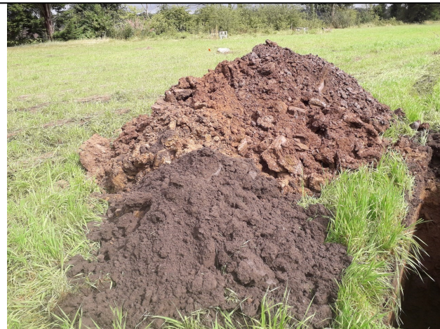
Trial Pit 134 Spoil
