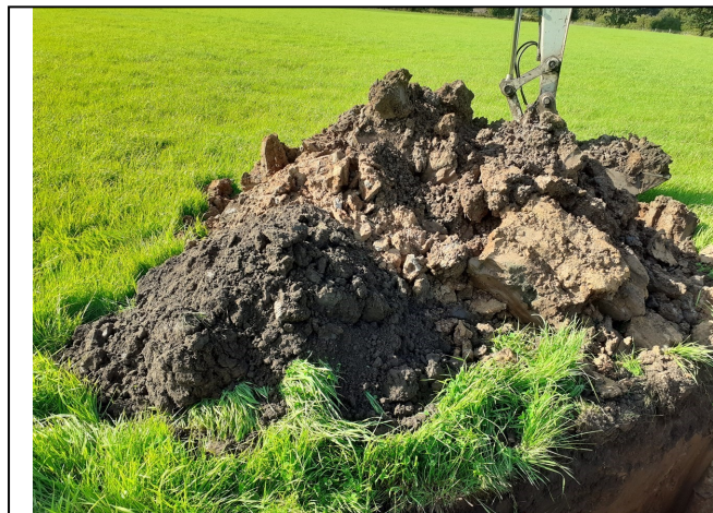
Trial Pit 119 Spoil
