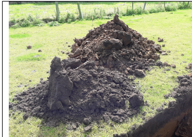
Trial Pit 141 Spoil
