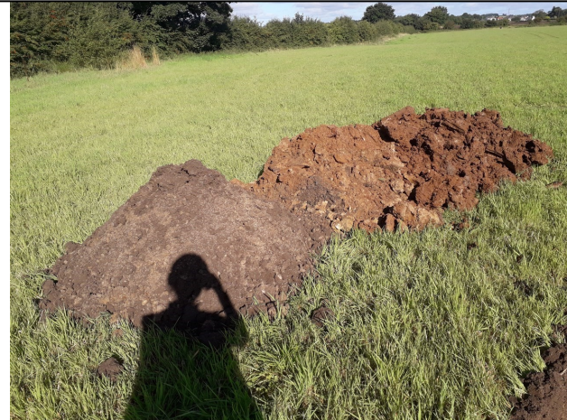
Trial Pit 102 Spoil
