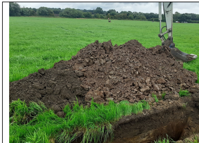
Trial Pit 127 Spoil
