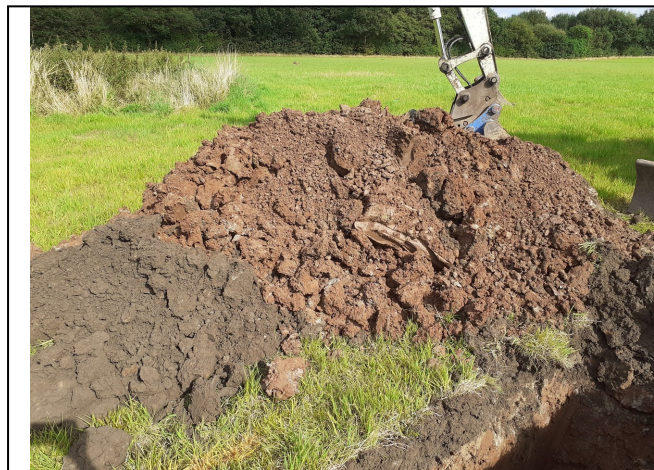
Trial Pit 118 Spoil
