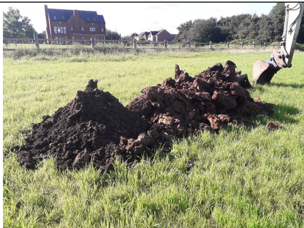
Trial Pit 101/ Soakaway 101 Spoil
