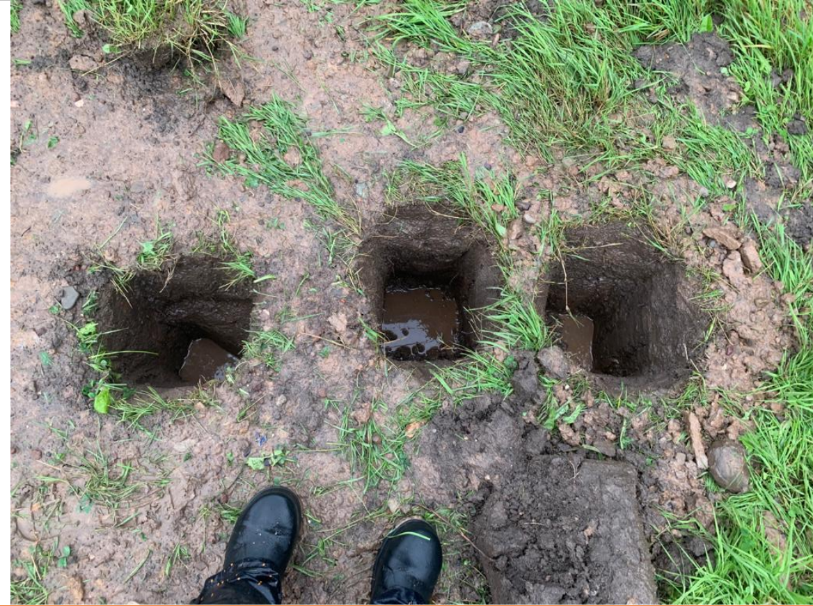
PLATE 7 HP101 LOCATING SURFACE WATER PIPE WITHIN CENTRAL FIELD
