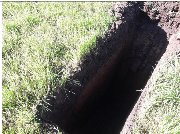
Trial Pit 101/ Soakaway 101
