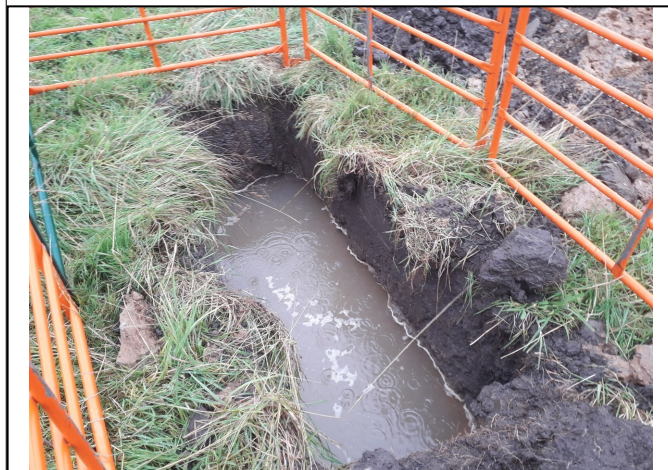
Trial Pit 105/ Soakaway 103
