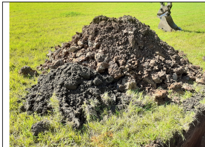
Trial Pit 115 Spoil
