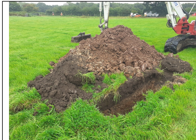
Trial Pit 122 Spoil
