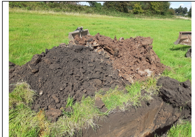
Trial Pit 112 Spoil
