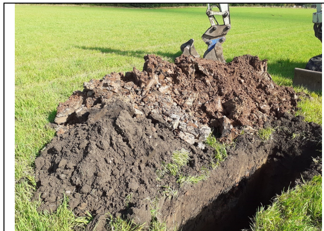
Trial Pit 117 Spoil
