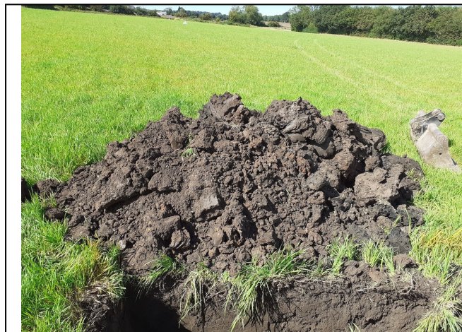
Trial Pit 116 Spoil
