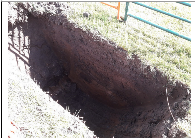
Trial Pit 108/ Soakaway 106
