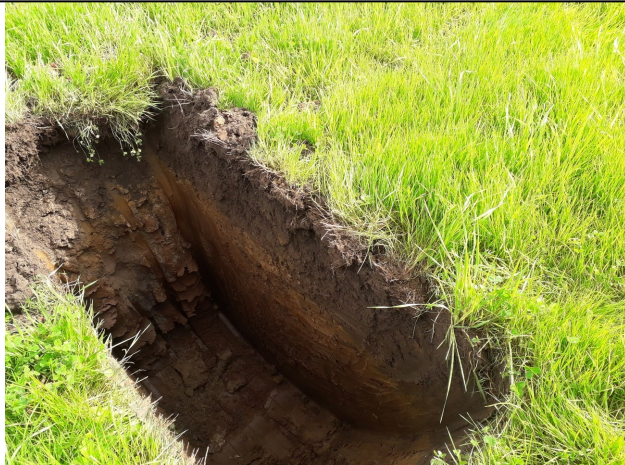
Trial Pit 107/ Soakaway 105
