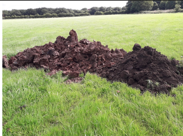
Trial Pit 107/ Soakaway 105 Spoil
