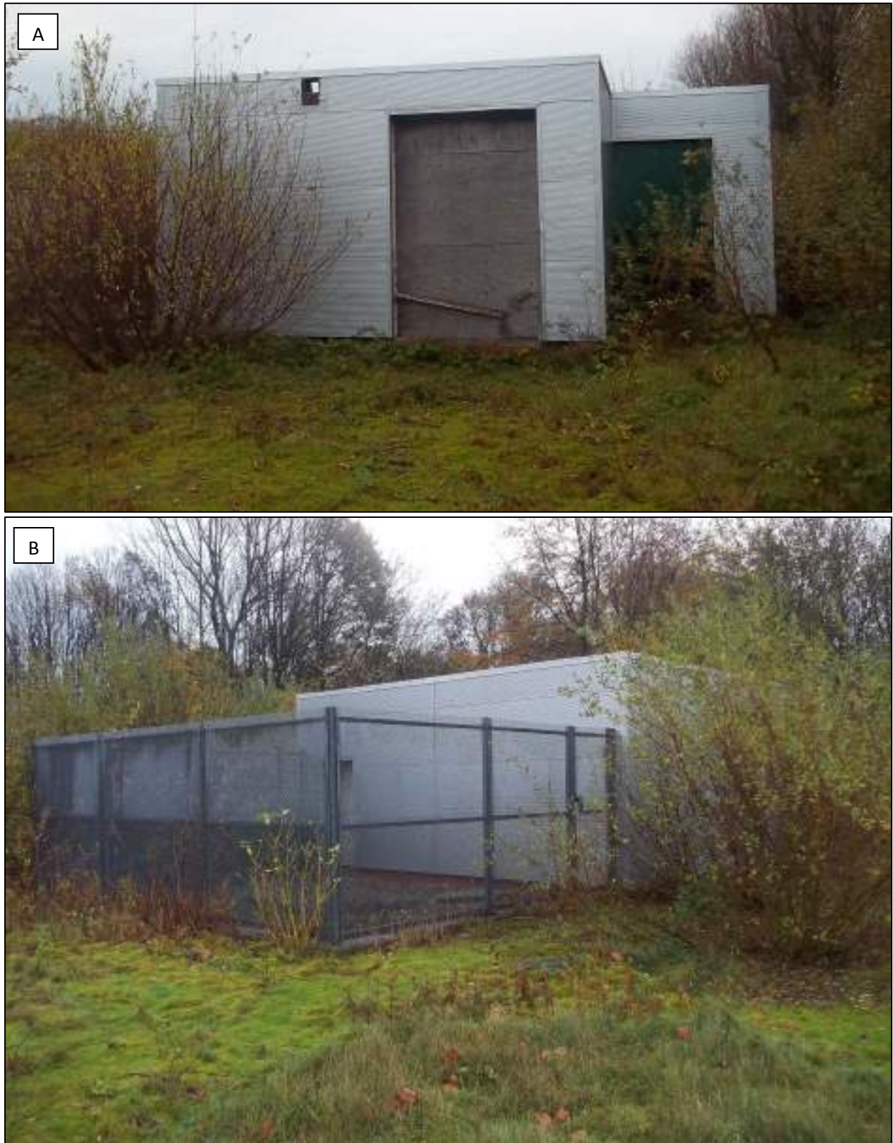
Photograph 5: View northeast and east of derelict structure near the southern corner of the site.
