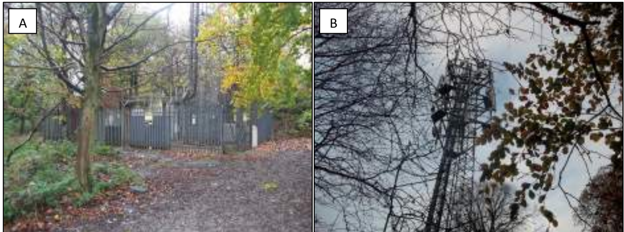
Photograph 14: View of substation and communications tower off site (close to the north western corner).
