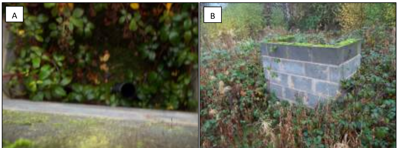
Photograph 11: View of brick structure surrounding a pipe adjacent to the north western site boundary in the west of the site.
