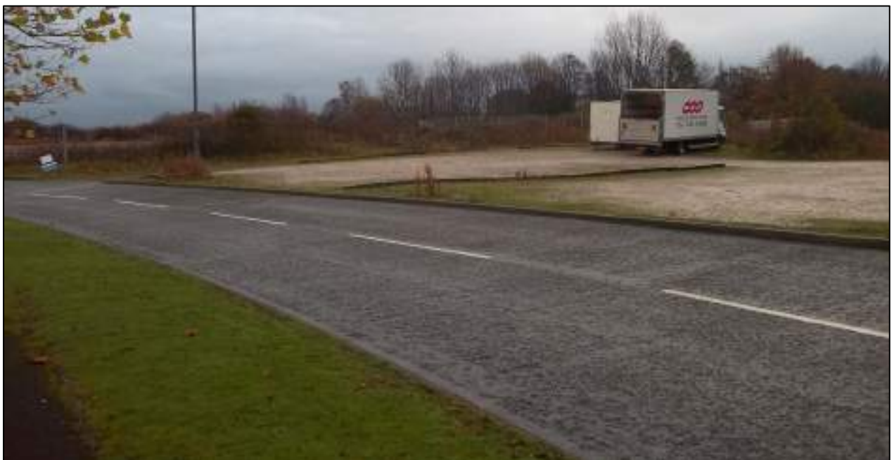
Photograph 2: View east of site entrance and temporary gravel carparks from the western corner of the site.
