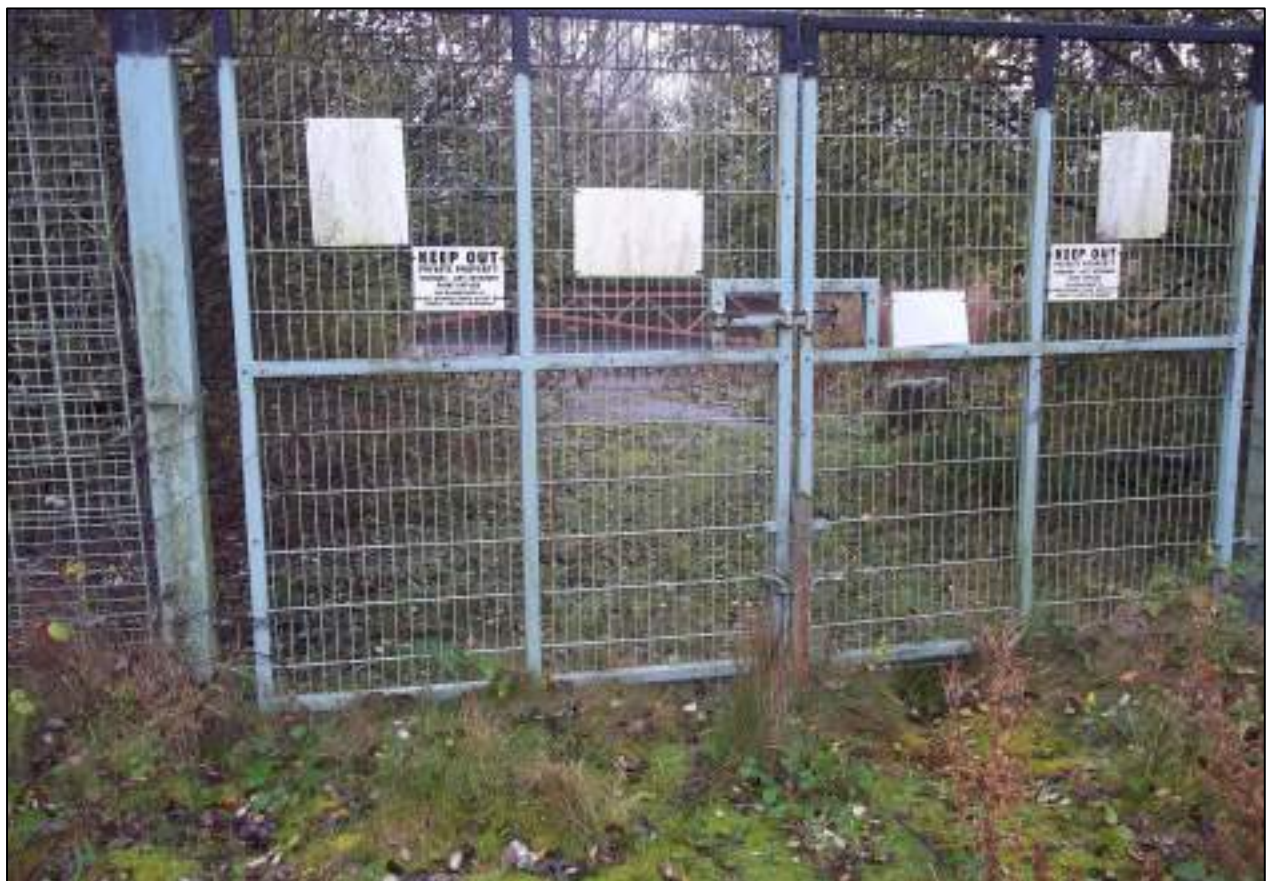
Photograph 4: View southeast of gated alternate site entrance from Huyton Lane in the southern corner of the site.
