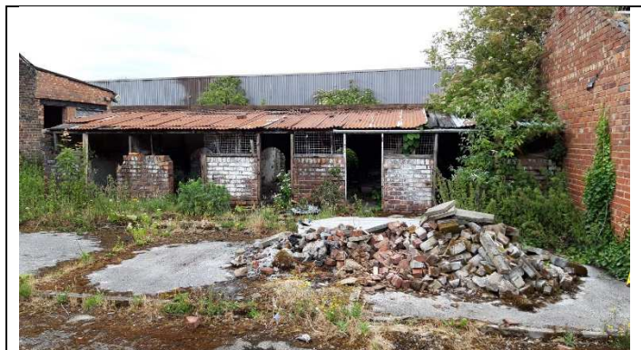
Fig.08 – Western Kennel Building Viewed from South
