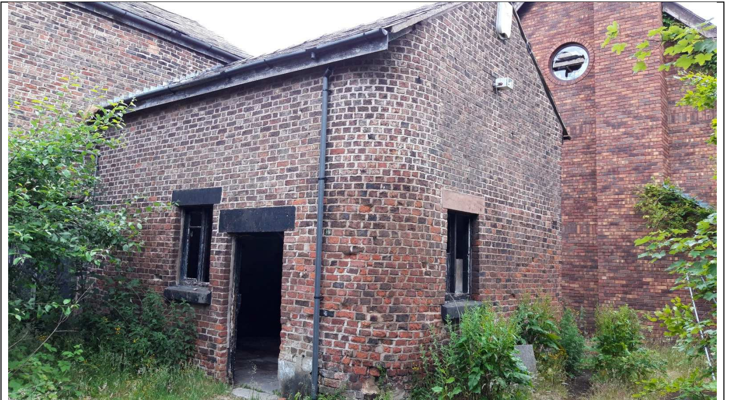
Building F8 – Outrigger Building to South East
