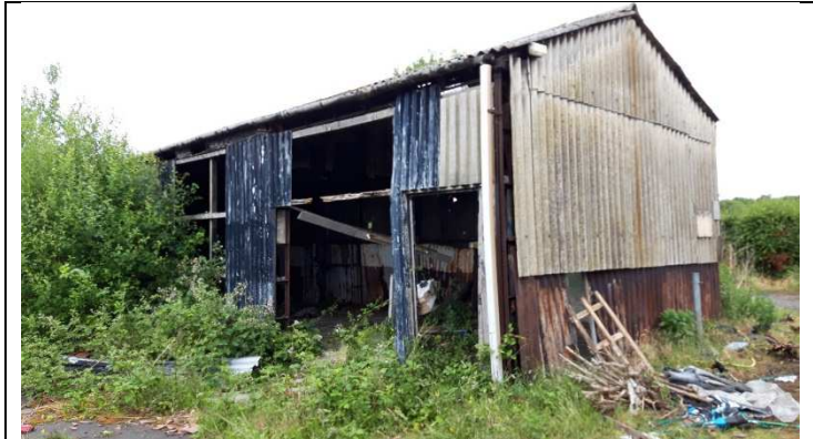
Fig.05 – Shed at South End of Block, From West
