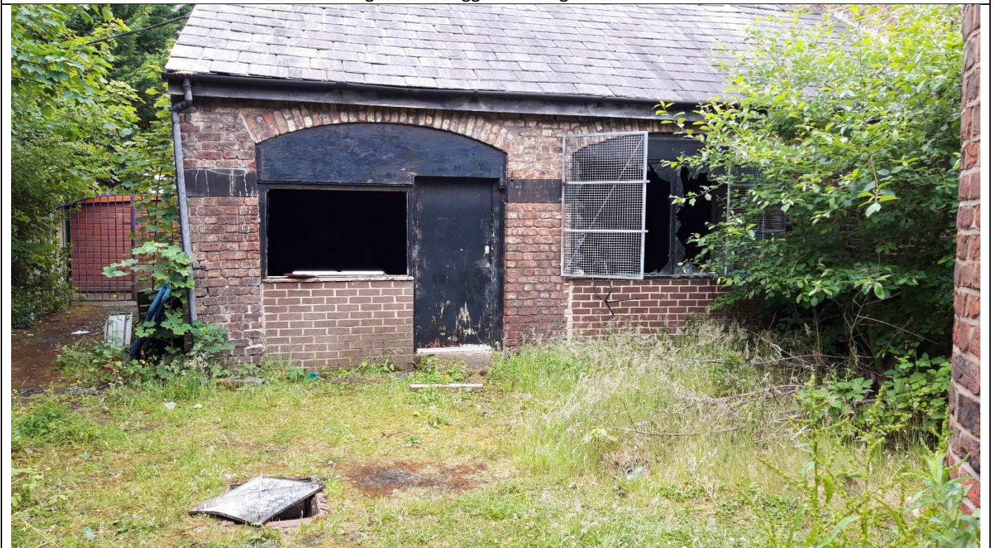
Building F8 – Outrigger Building to Midpoint of South Elevation
