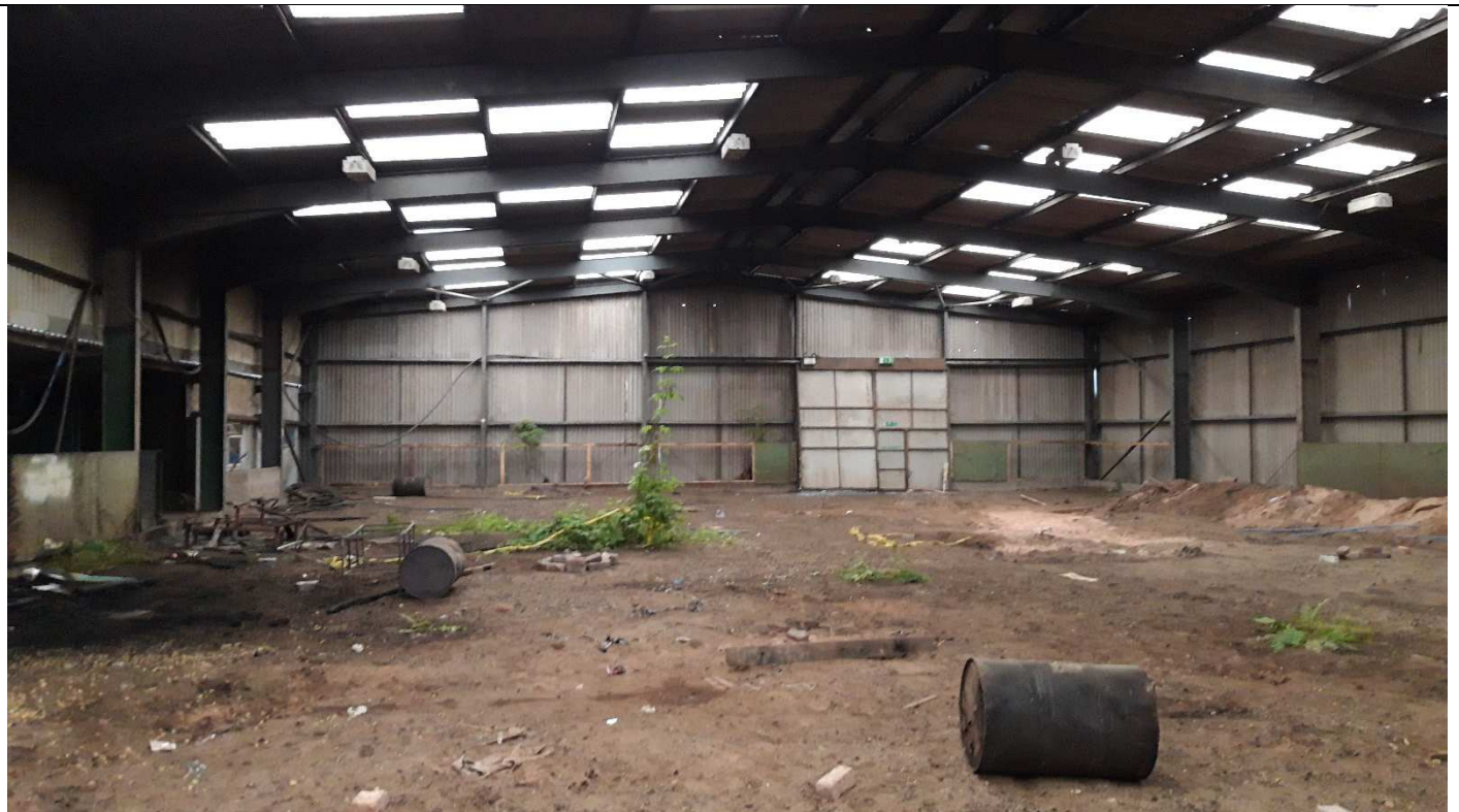
Internal View of Building F3 – Main Portal Frame Building
