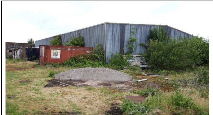
Fig.03 – Min Portal Seen from South East
