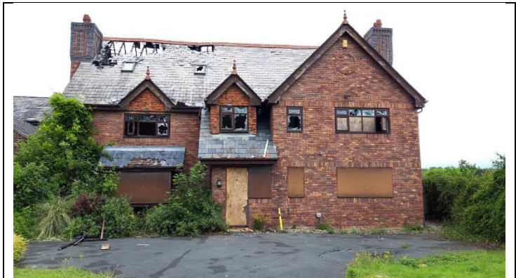
Fig.10 – Dwelling House Viewed from South
