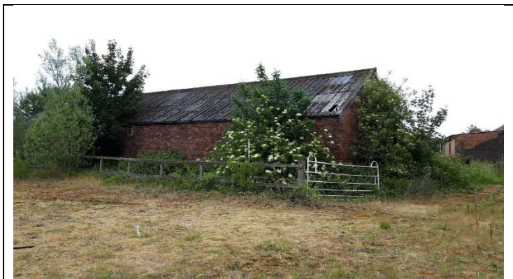
Fig.04 – Building Viewed from South West
