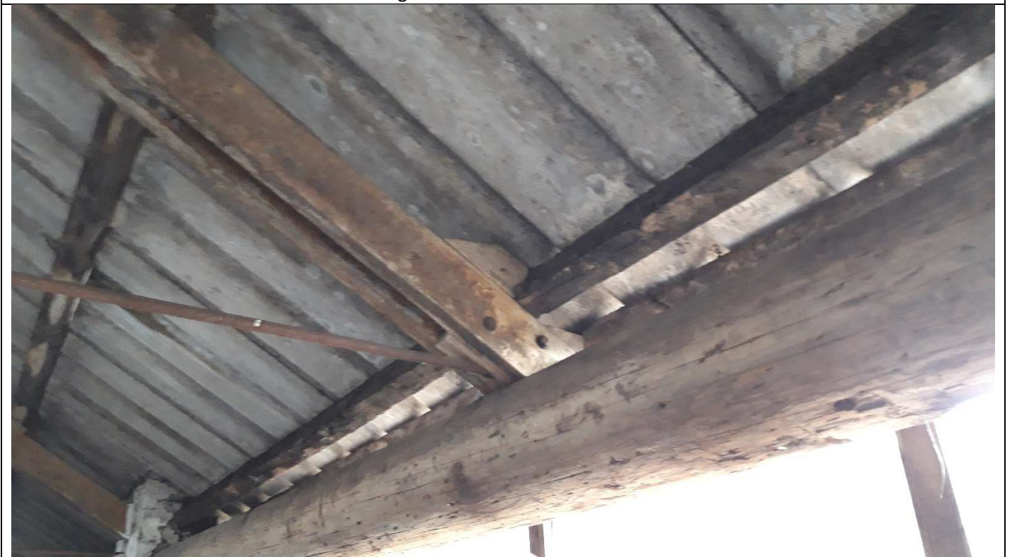
Building F4 – Detail of Truss & Large Eaves Timber Member
