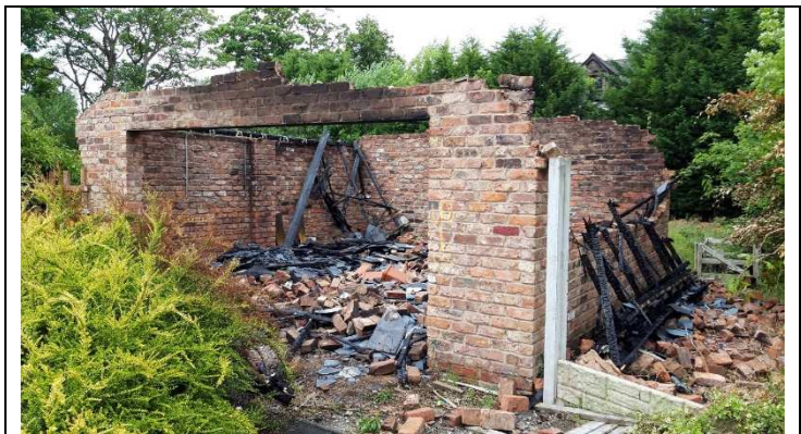
Fig.11 – Remains of Garage, Viewed from East
