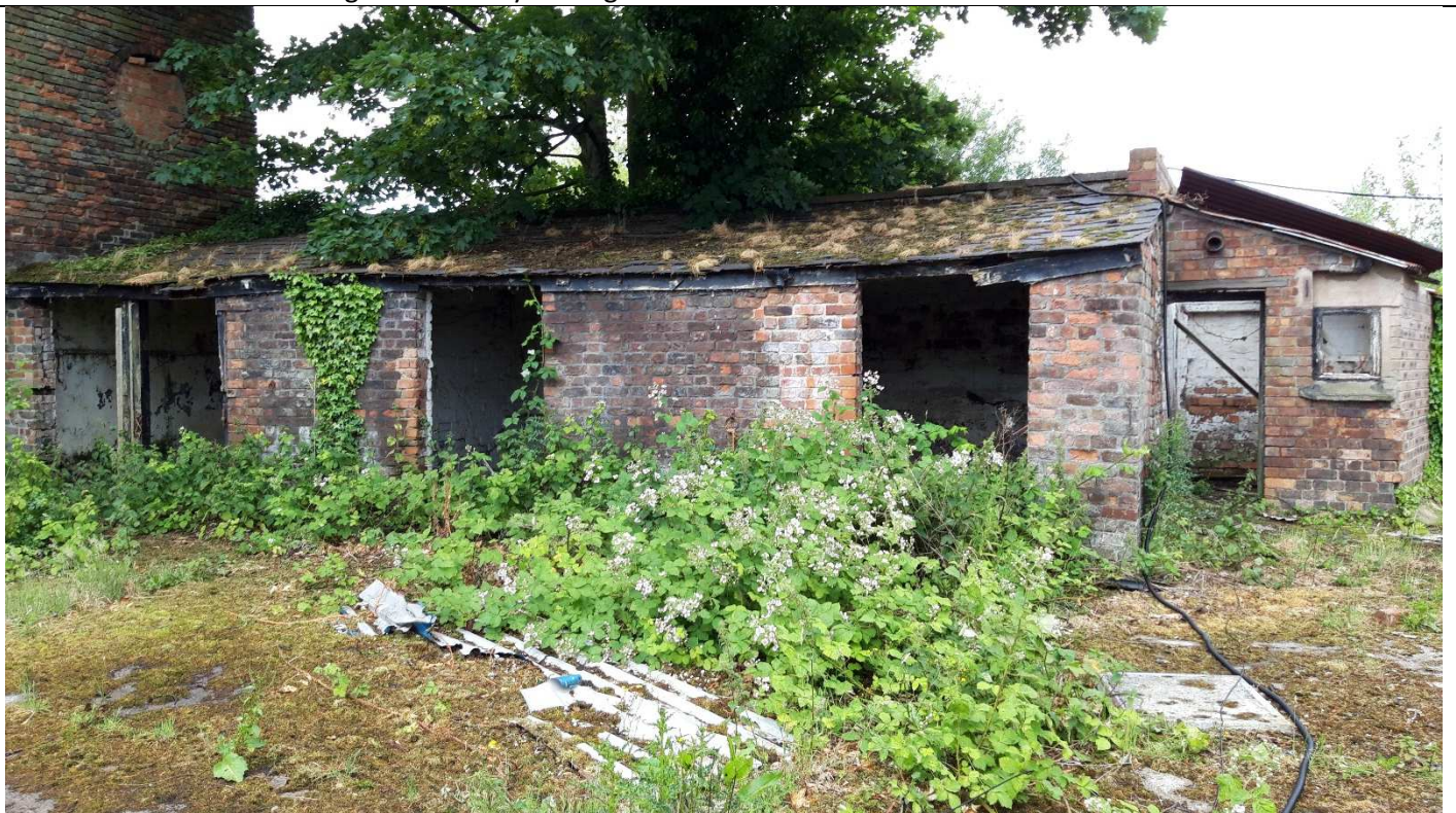
Building F8 – Outrigger Required for Removal at North West
