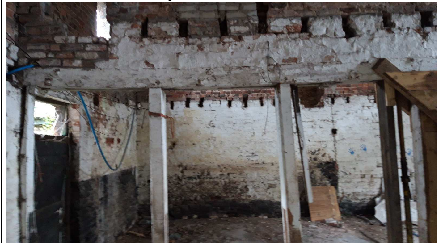
Building F8 – Propping to Partition Wall at East End
