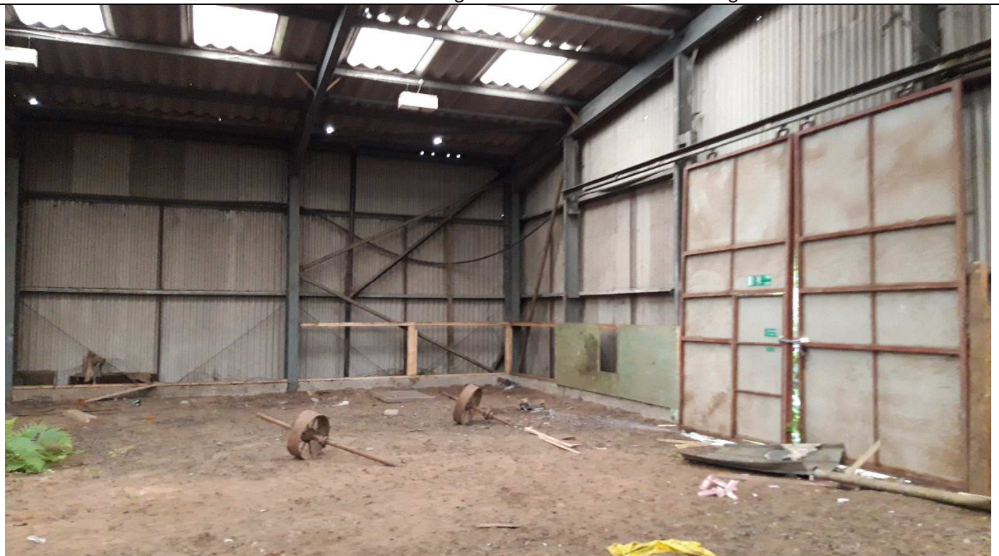
Building F3 – Typical Bracing at Corner of Building & Earth Floor
