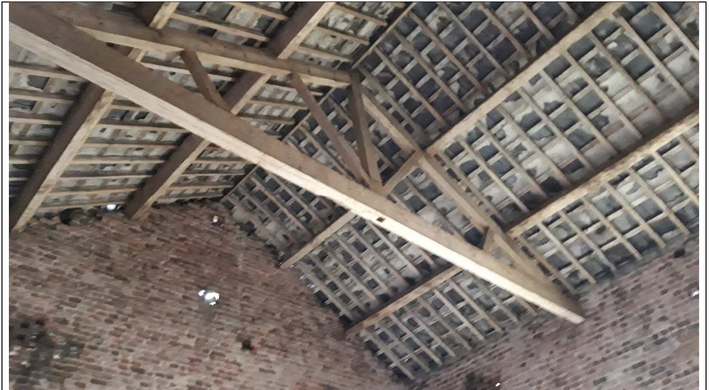
Building F8 – Detail of Main Roof Structure
