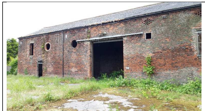
Fig.09 - Barn Viewed from North West
