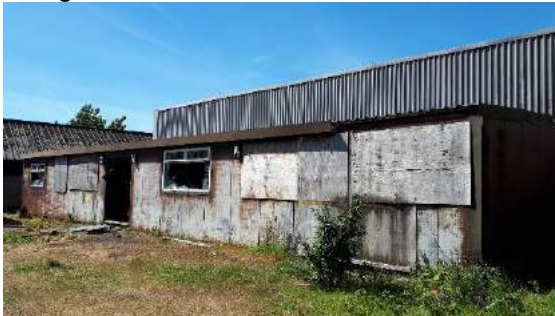
Photograph 42: B16b in foreground, B16a in the background.
