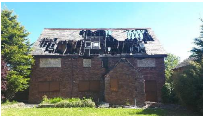
Photograph 30: B11 northern aspect.
