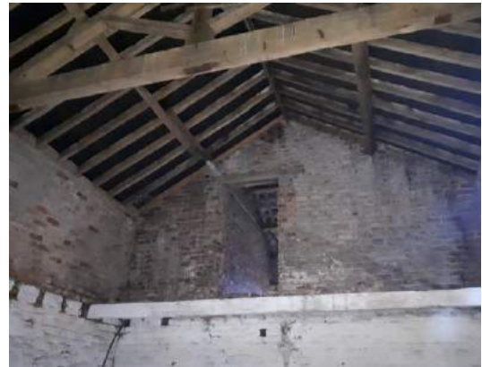
Photograph 24: Interior aspect of B2.
