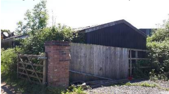
Photograph 47: B19 north-eastern aspect.
