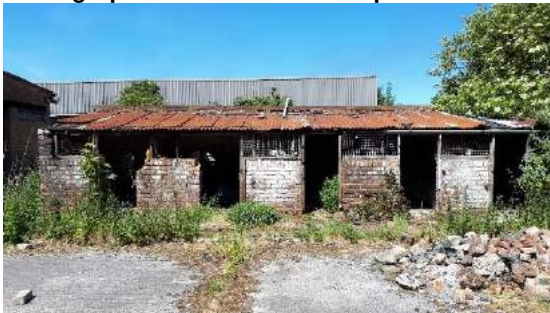
Photograph 34: B13 southern aspect.
