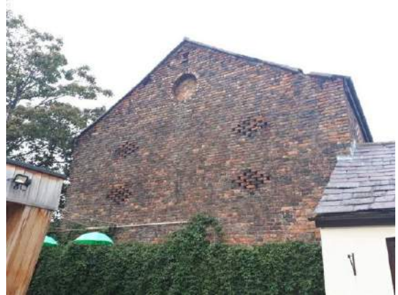
Photograph 21: South-western gable end of B1.
