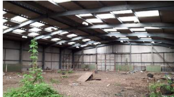
Photograph 43: Interior of B16a.
