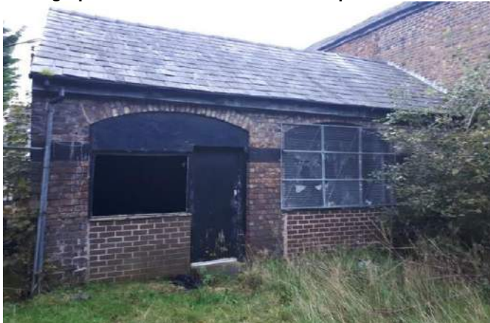
Photograph 25: External north-eastern aspect of B3.
