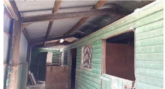
Photograph 48: Interior of B19.
