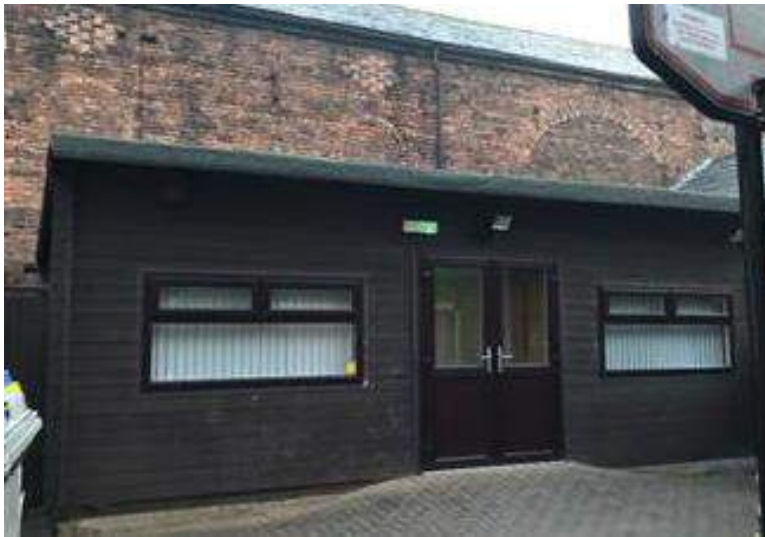
Photograph 26: External south-eastern aspect of B4.
