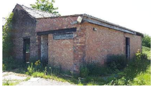
Photograph 37: B14 north-eastern aspect.
