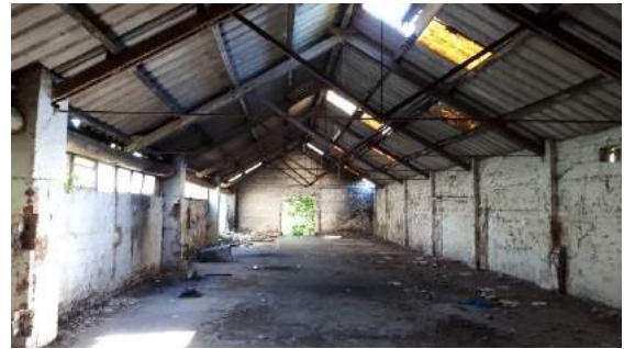
Photograph 41: Interior of B15a.
