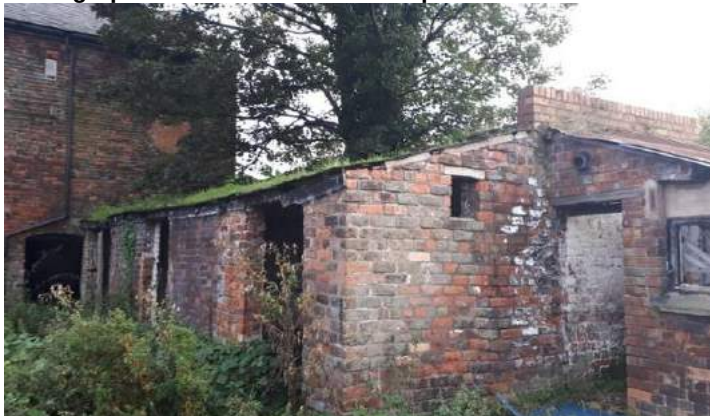
Photograph 27: External northern aspect of B5.
