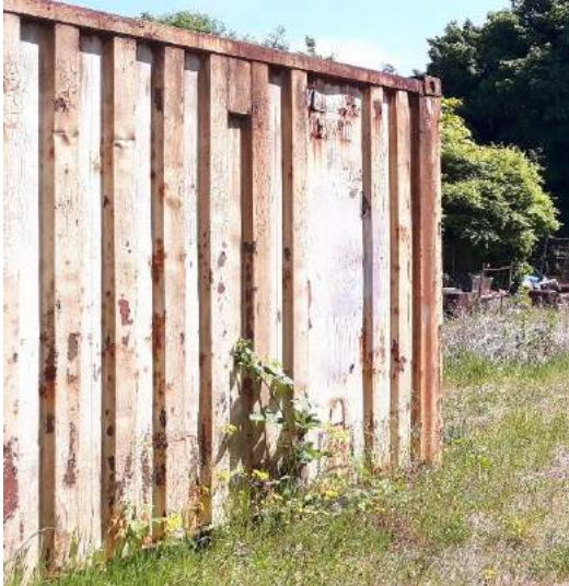
Photograph 28: Western aspect of B9.
