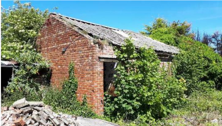
Photograph 32: B12 south-western aspect.
