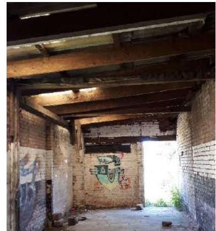
Photograph 39: Internal roof structure of newer part of building B14.
