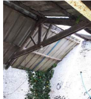
Photograph 33: Internal roof structure of B12.
