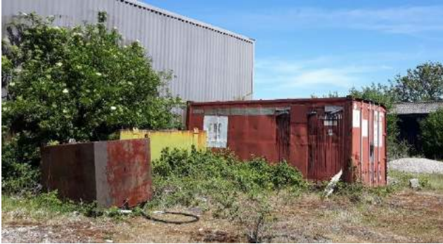
Photograph 44: B17 south-western aspect.
