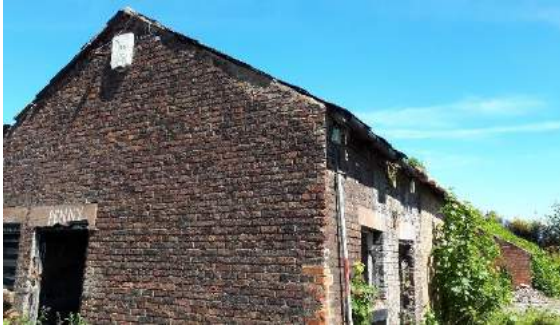
Photograph 36: B14 south-western aspect.
