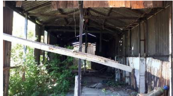
Photograph 46: Interior of B18.
