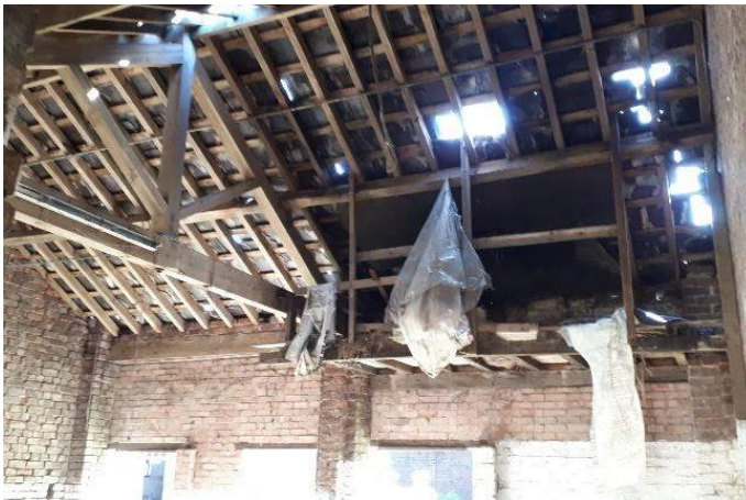
Photograph 38: Internal roof structure of older part of building B14.
