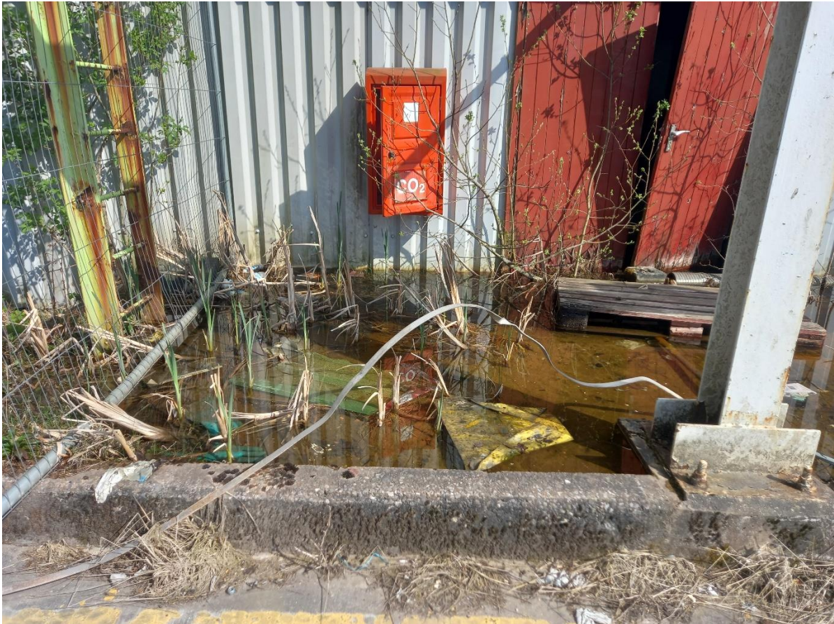
Photograph 3: Shallow pool in footing of Building 82 with “Poor” suitability for great crested newts (TN2)
