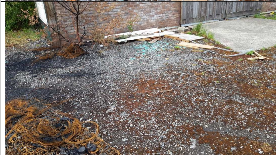
Photo 27: General detritus located in the area encompassing the cluster farm buildings and associated yard areas (north-east of the site)
