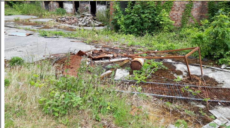
Photo 11: Rubble/steel/timber detritus located in the area encompassing the cluster farm buildings and associated yard areas
