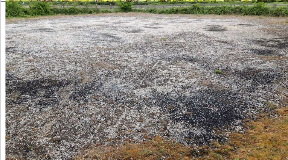
Photo 17: Ash within flint surfacing materials located in the yard areas present in the west of the site.
