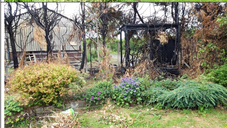
Photo 05: Fire damaged trees and pergola to house rear garden
