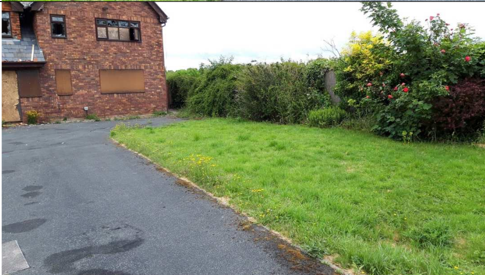
Photo 02: Eastern Boundary to Residential Property. Property is of brick construction with a slate roof.
