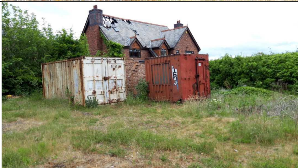
Photo 09: 2No. metal containers present in front garden area belonging to Whitehill House (south-eastern section of the site). Contents Unknown
