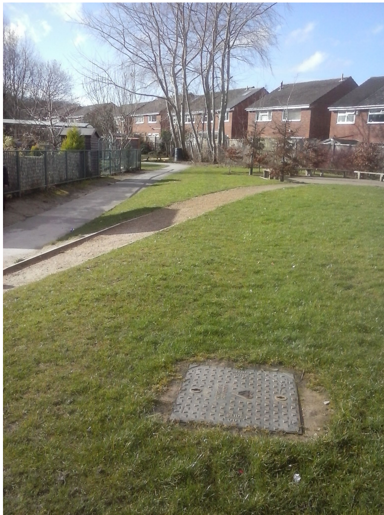
Presumed outfall for the northern cut-off drain
