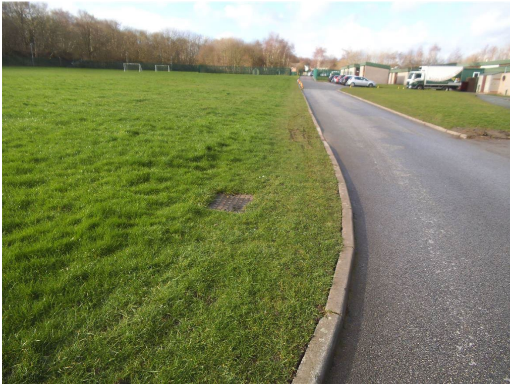
Manhole cover, north-east corner field
