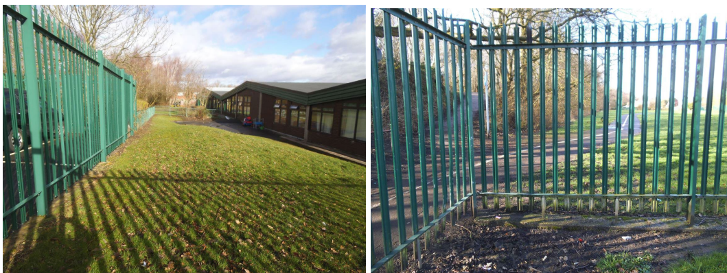
Security fencing to the perimeter
