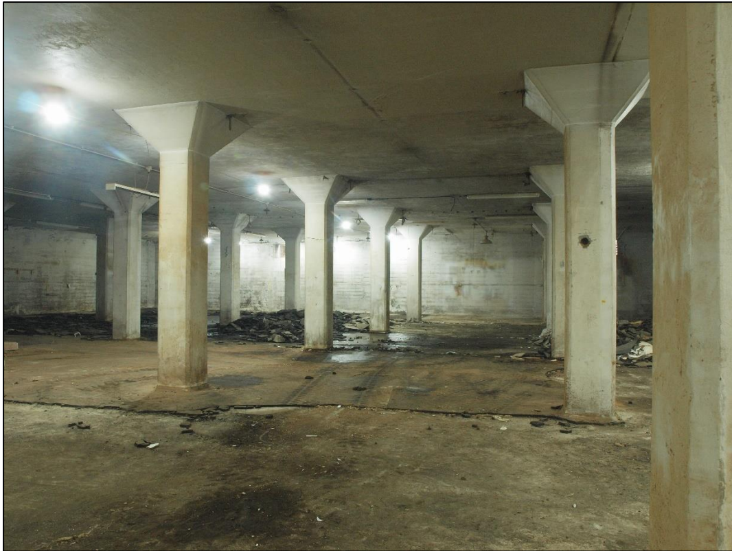
Plate 43: General shot of bunker
