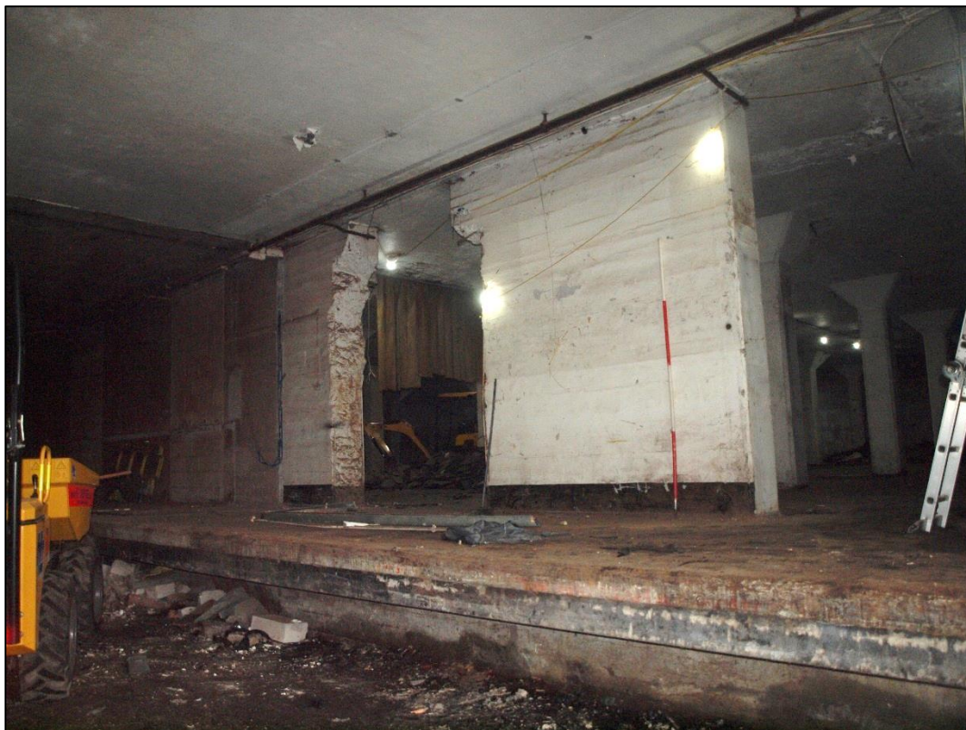
Plate 21: Loading bay showing widened opening to main bunker
