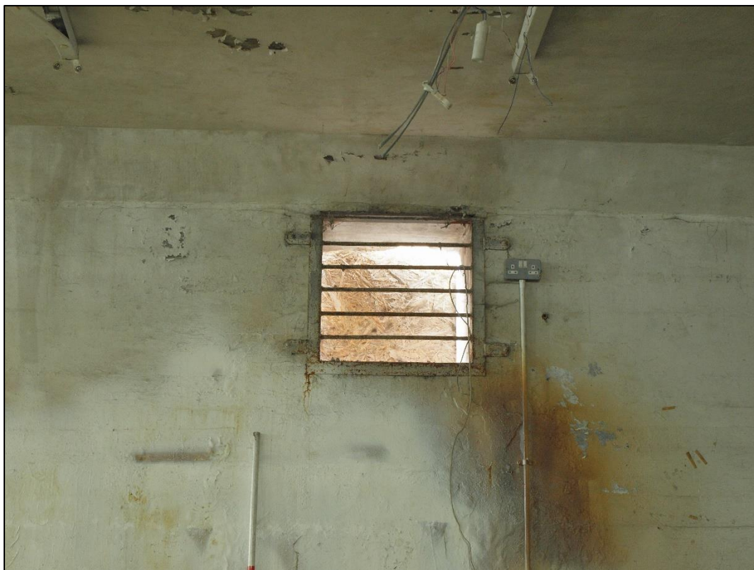
Plate 36: Detail of opening at northern end of west wall
