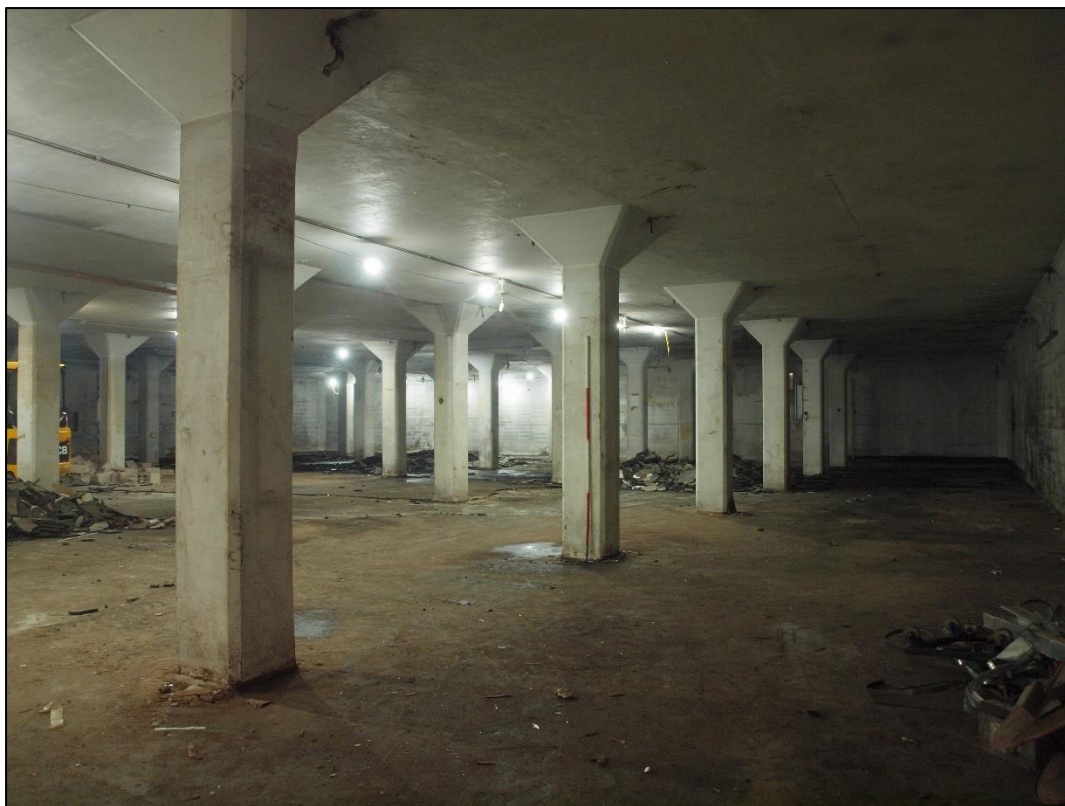
Plate 30: General shot of main bunker from northeast corner
