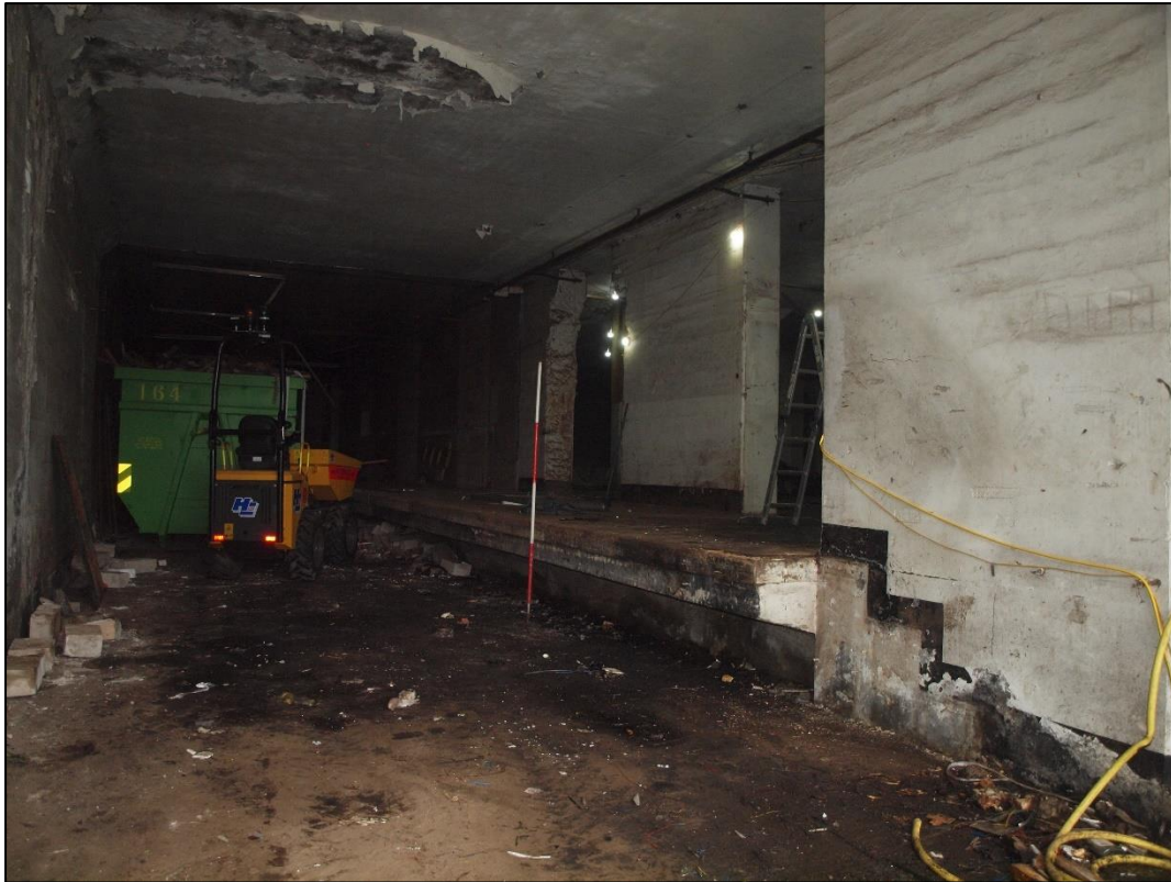
Plate 17: Northern end of loading bay looking south
