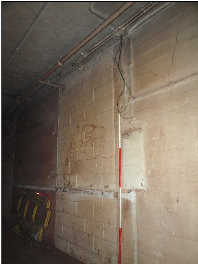
Plate 23: Blocked opening between loading bay and main bunker
