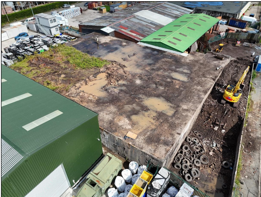
Plate 44: Roof after stripping
