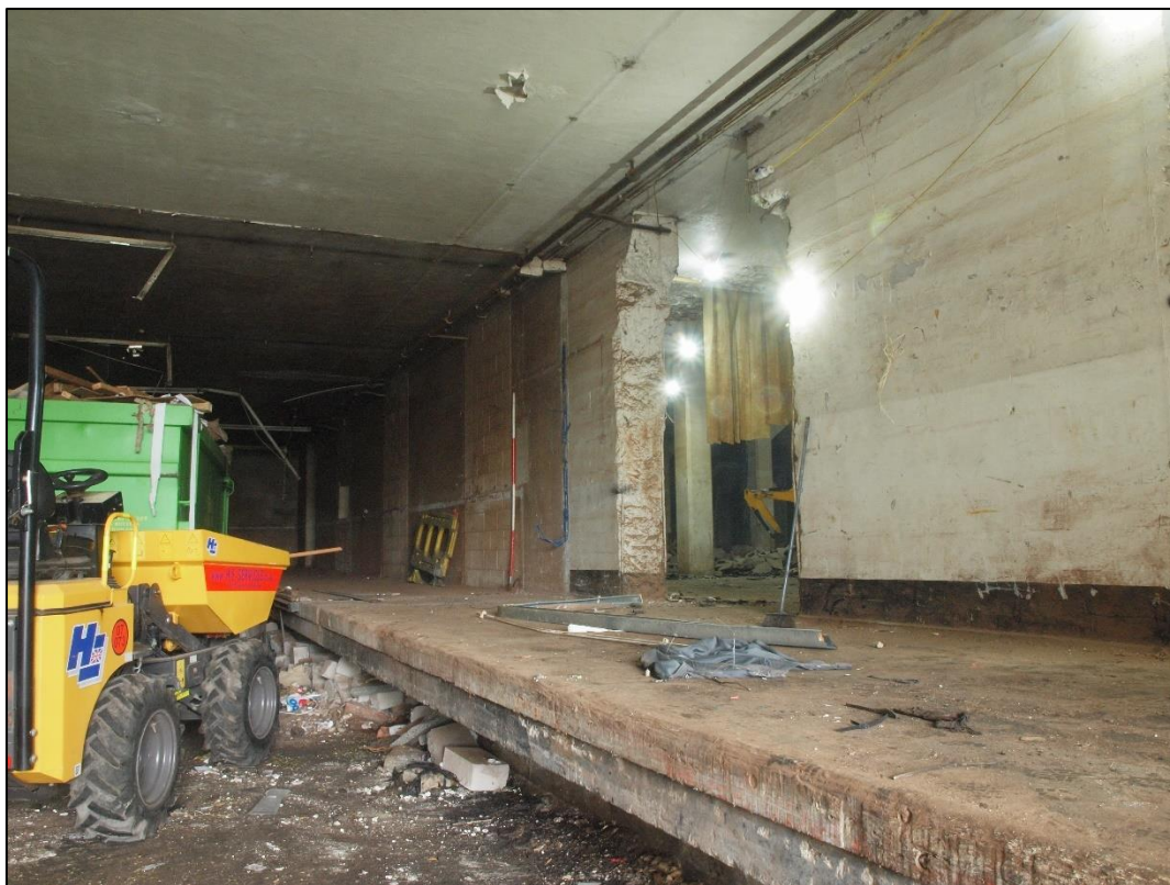
Plate 22: View along loading bay
