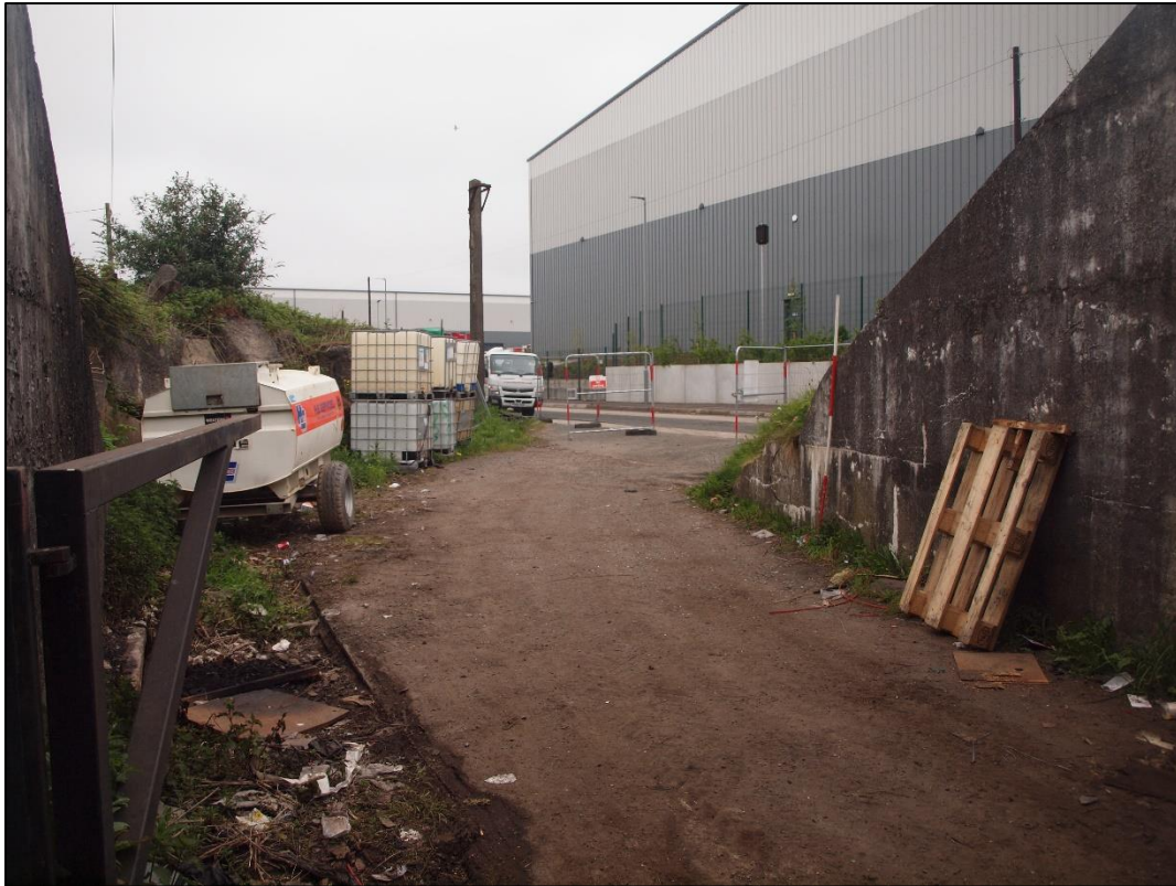
Plate 9: View out from the entrance showing remains of railway line
