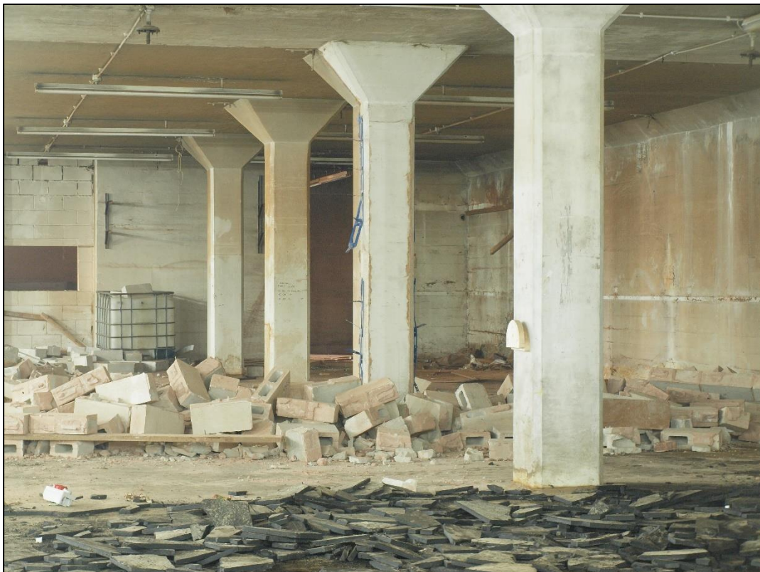
Plate 38: View east from southwest corner
