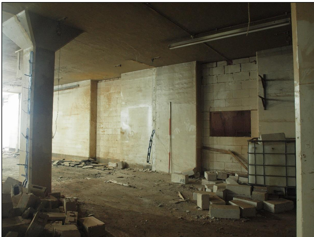
Plate 40: Wall to loading bay with blocked openings
