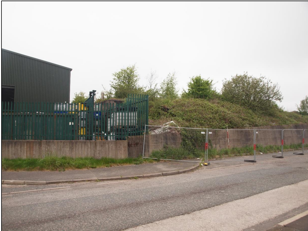
Plate 5: Overgrown foliage visible to east elevation
