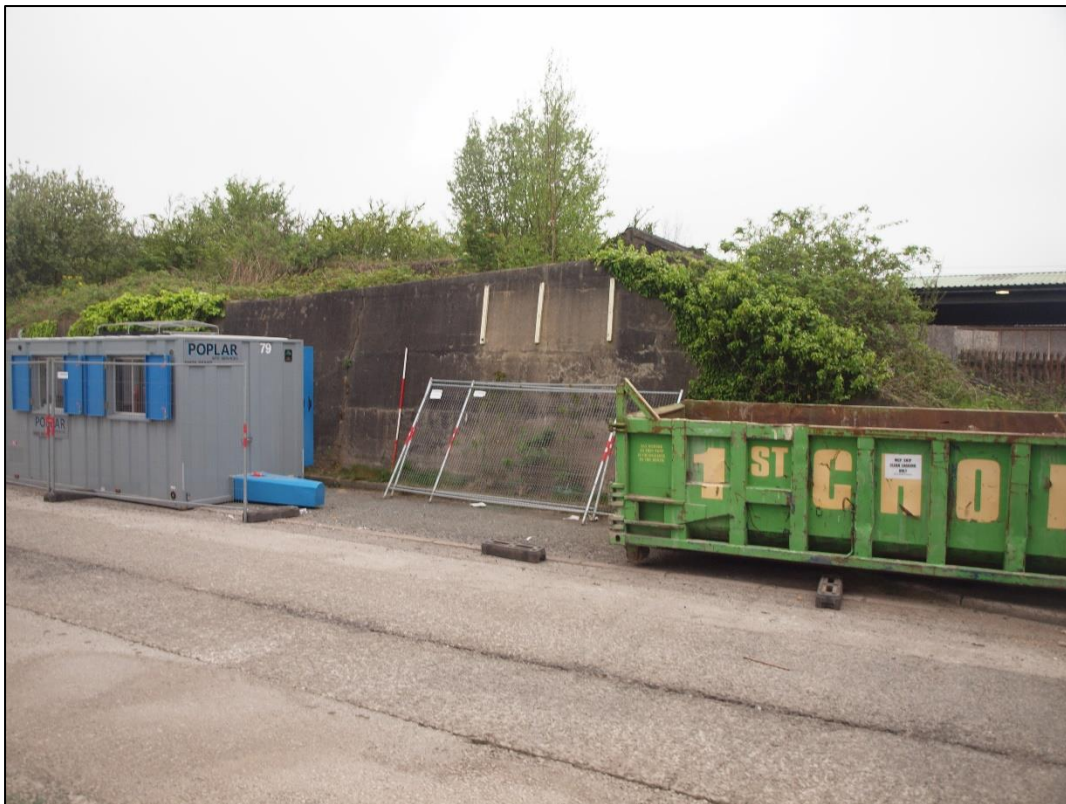
Plate 2: Northern end of east elevation
