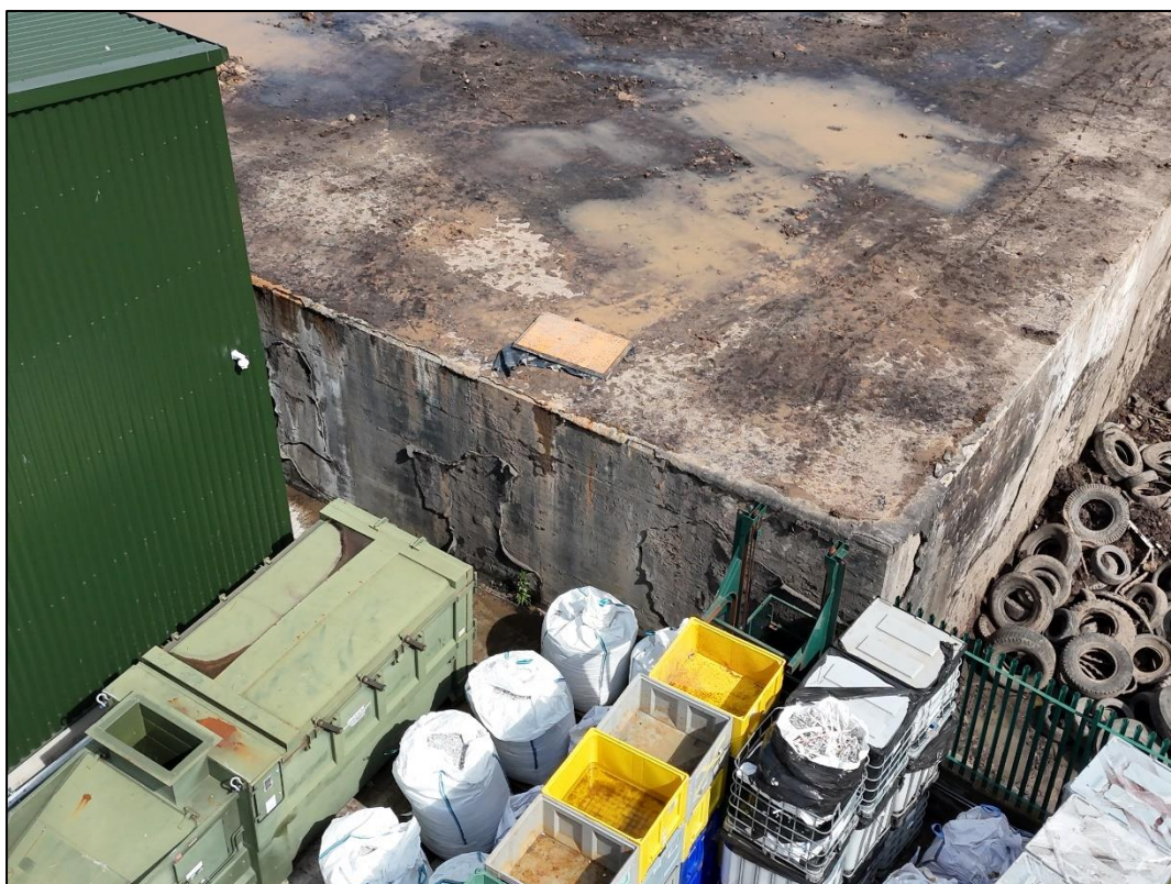
Plate 16: East end of southern wall visible
