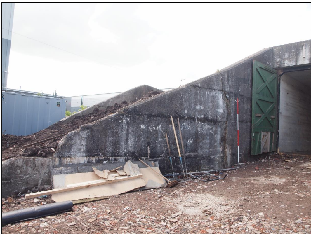
Plate 14: Eastern blast wall
