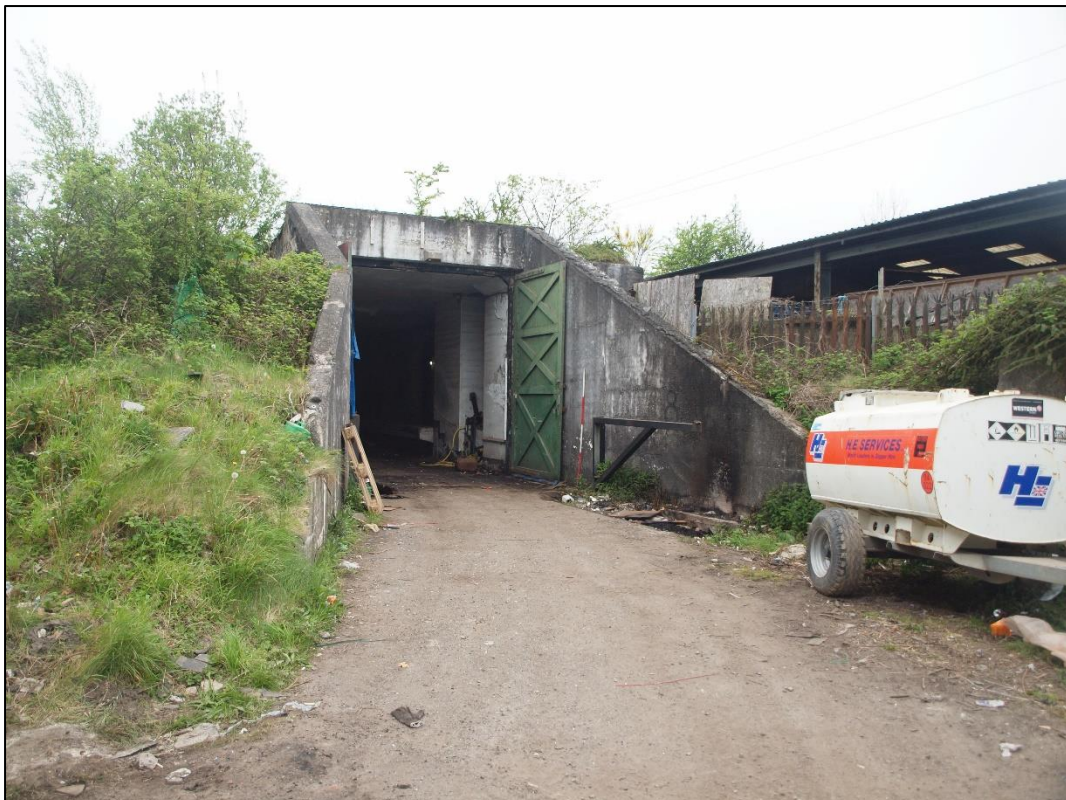
Plate 6: Entrance and blast walls to north elevation
