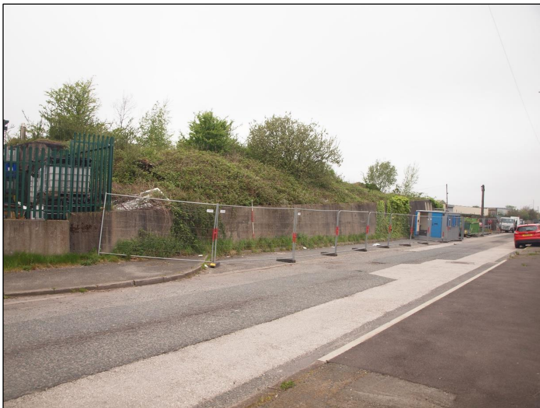
Plate 4: View of east elevation looking north up Draw Well Road
