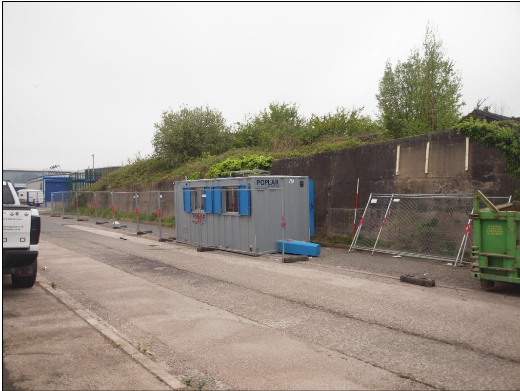
Plate 1: General shot of the bunker from Draw Well Road
