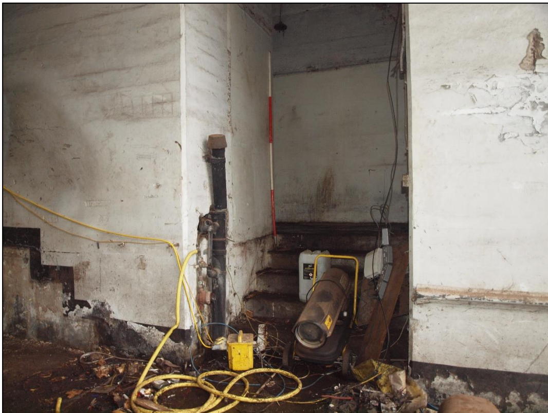
Plate 18: Staircase up to loading bay
