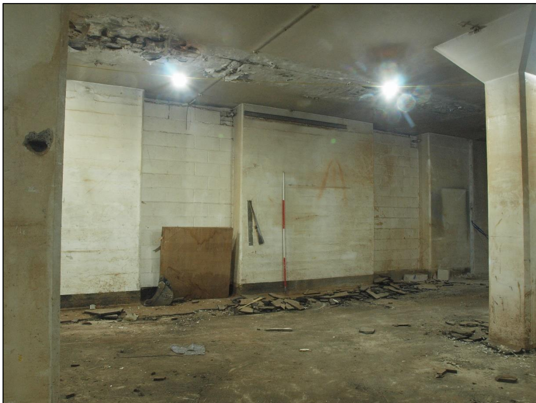
Plate 41: Detail of blocked openings
