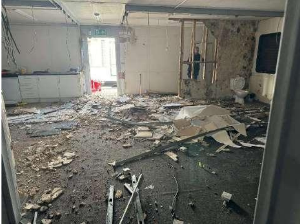
P10: Inside the temporary cabin
