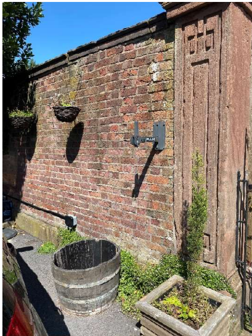
Plate 7 – Tv bracket installed to the southwest elevation of the enclosing brickwork wall which is to be removed.
