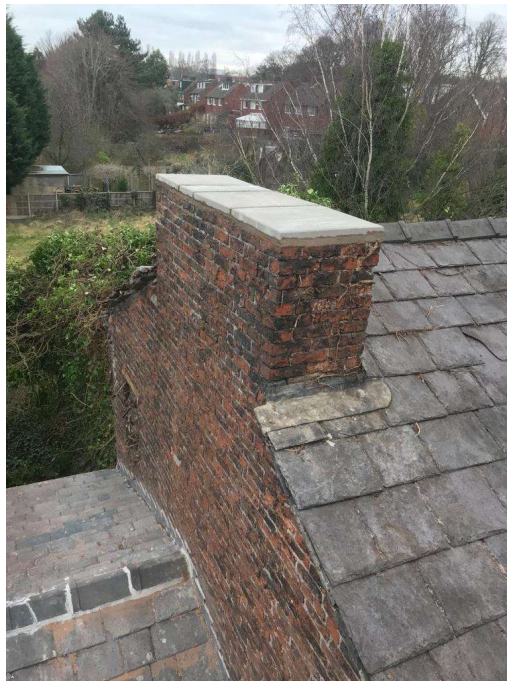
Plate 4 – Partially dismantled chimney stack to the stable block.
