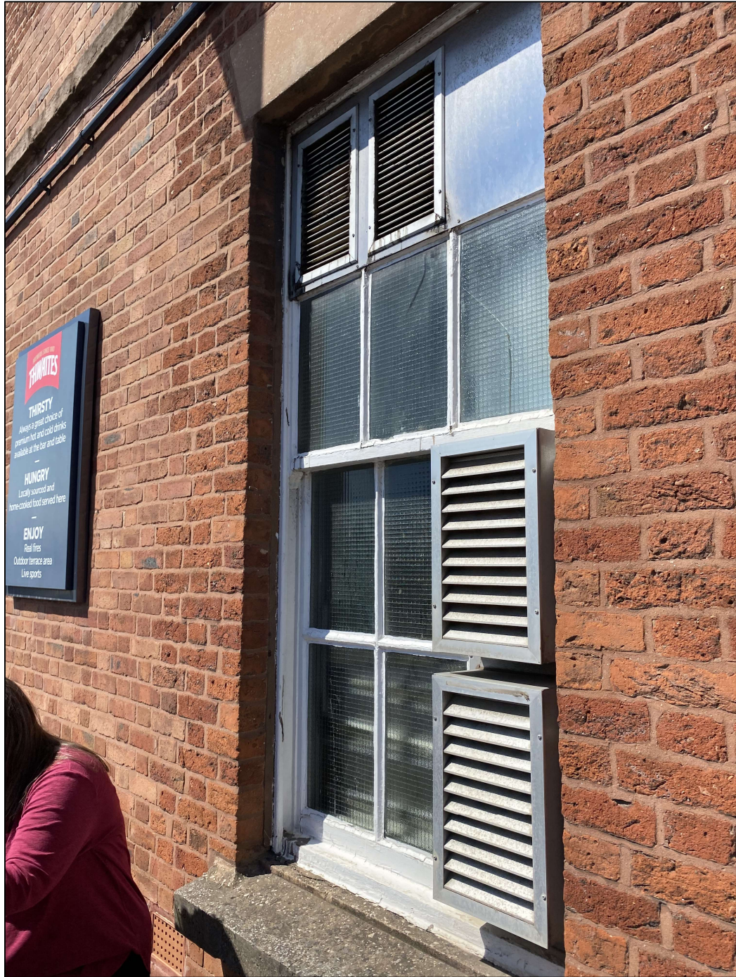
Plate 1 – Window as existing
