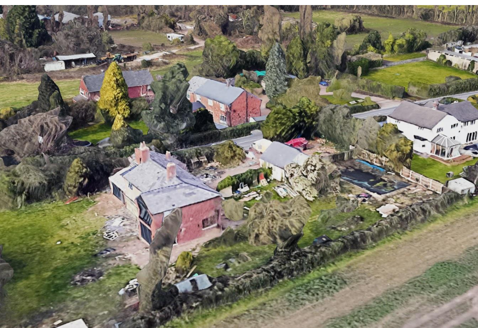
Figure 5.1 – Aerial View towards Entrance
