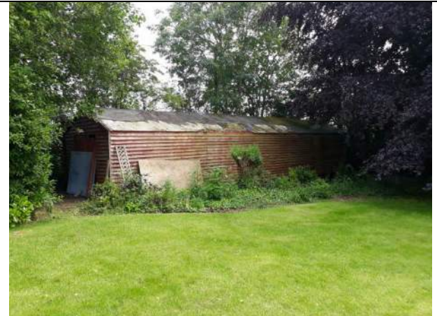
Photograph 7.10: Dwelling northern and western elevation
