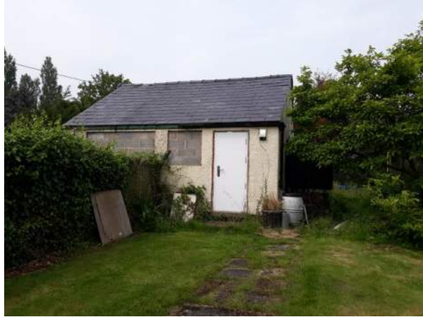
Photograph 7.5: Existing garage southern elevation
