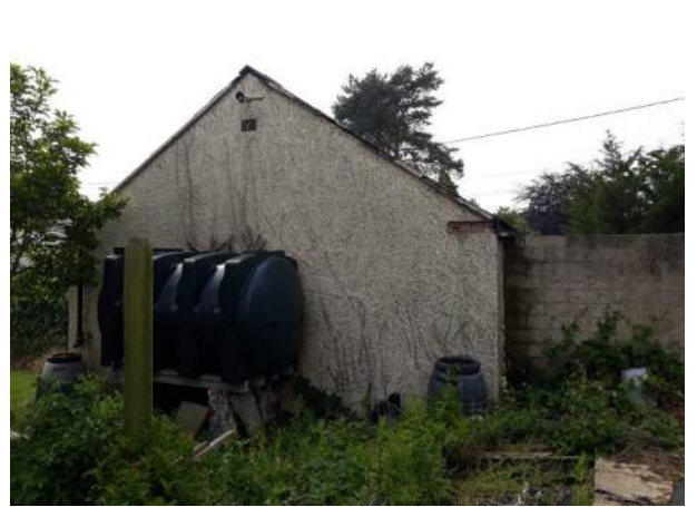
Photograph 7.6: Existing garage eastern elevation
