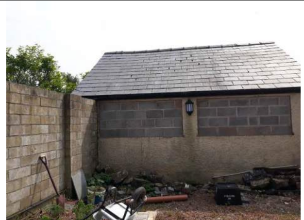
Photograph 7.8: Existing garage northern elevation
