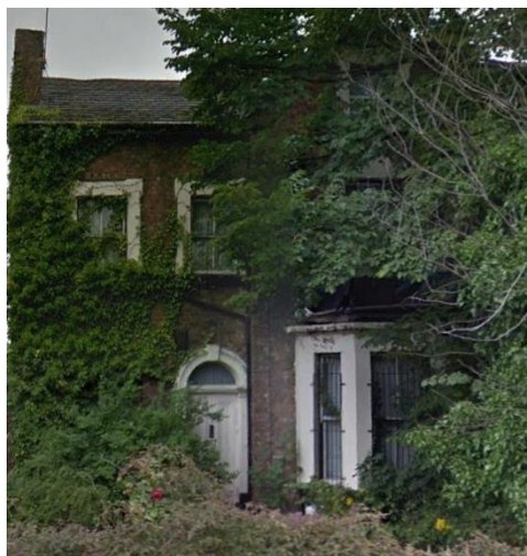
Above: Existing front door to be retained for separate access to the educational facilities
