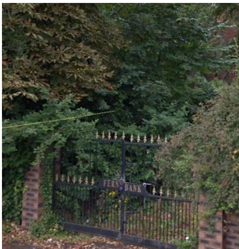
Above: Original gates to be replicated on new vehicle & pedestrian gates entering the proposed parking area.
