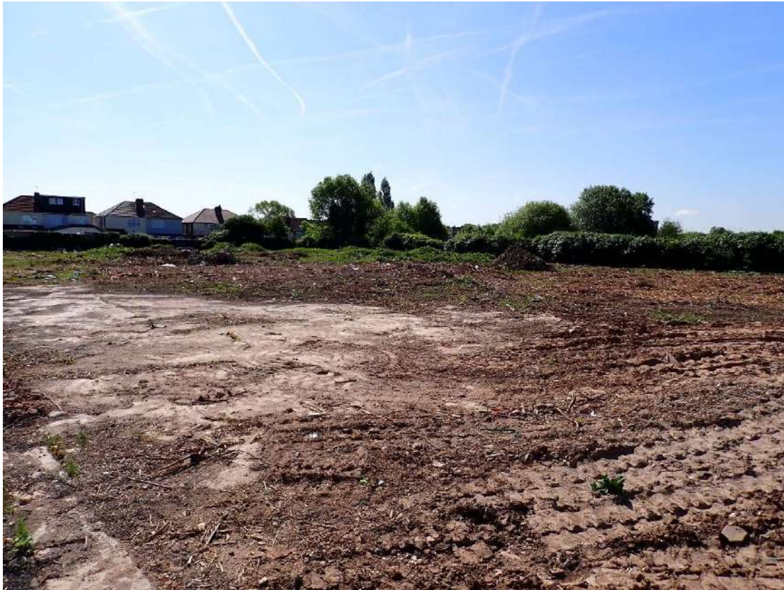
Photograph 1. Looking south across the proposed development site.
