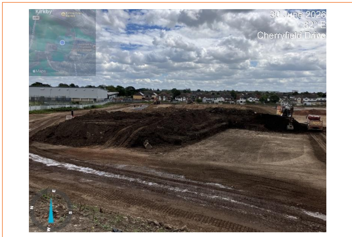
Plate 7 Removal of Topsoil from David Wilson Phase 1
