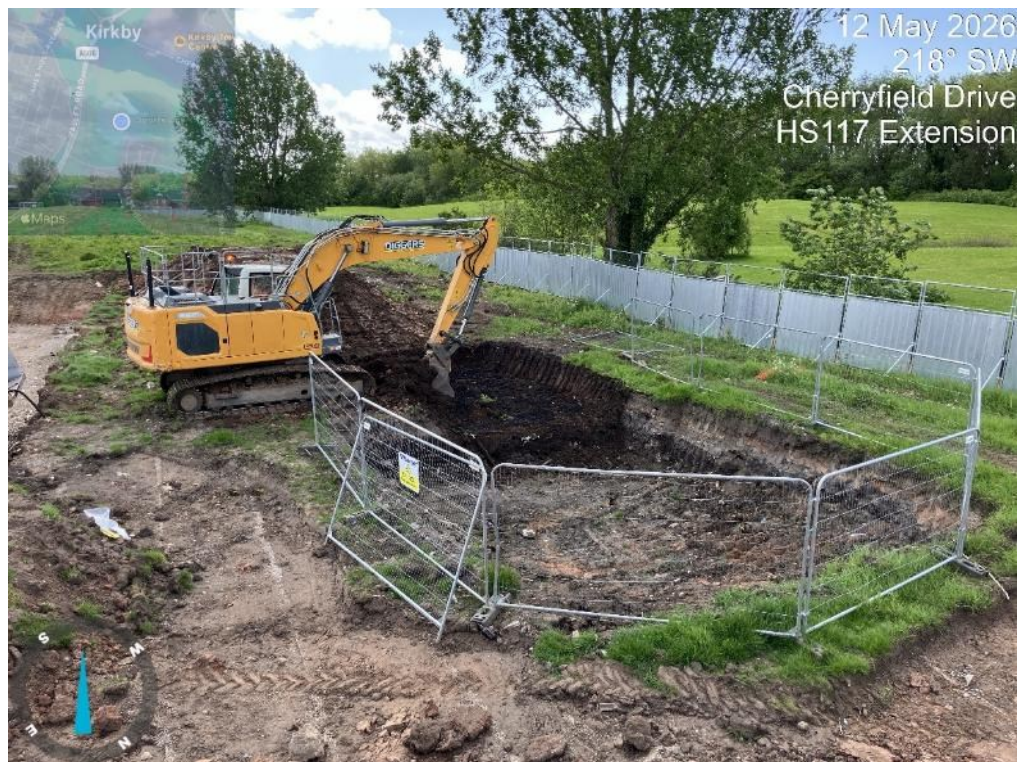
Plate 3 Fencing of Excavations and the Site Boundary
