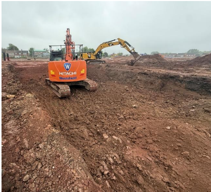
Plate 15 Removal of Heave Impacted Clay Soils
