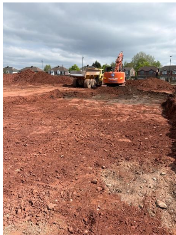
Plate 14 Removal of Heave Impacted Clay Soils
