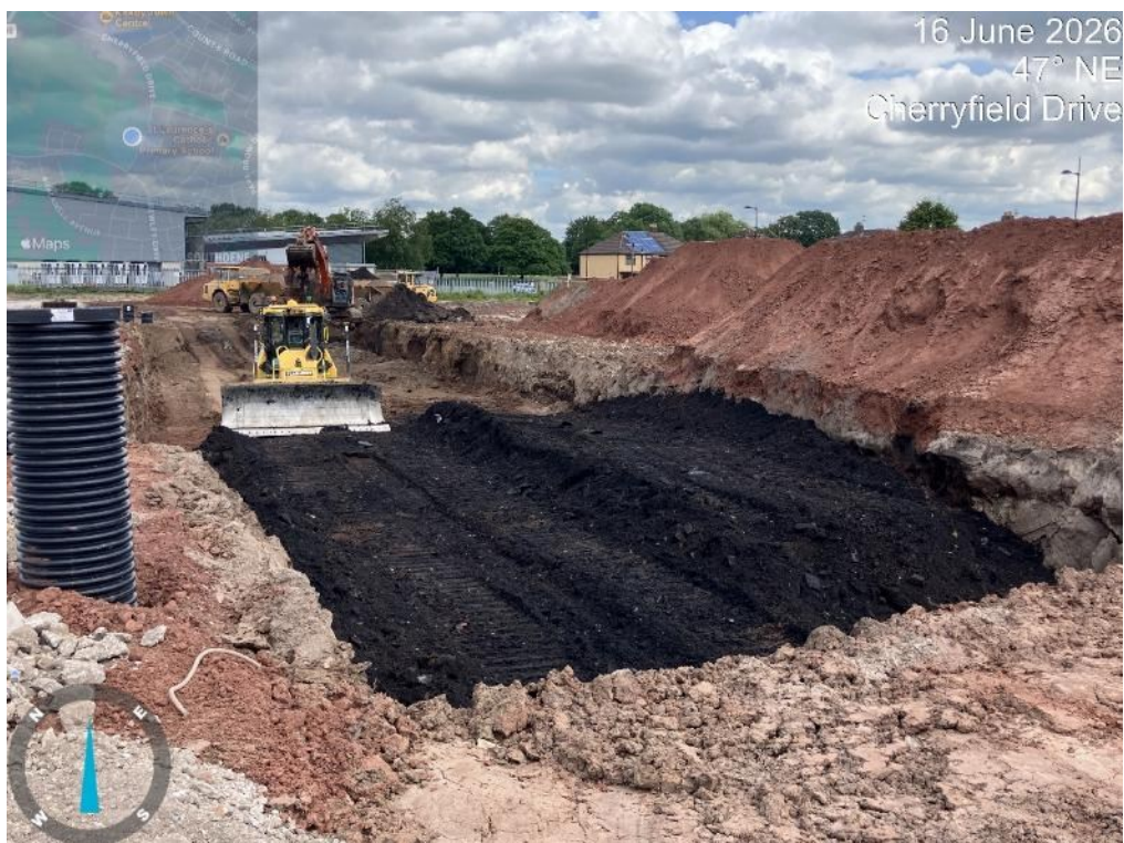
Plate 20 Upfill with Site-Won Granular / Non-Heave Impacted Cohesive Materials
