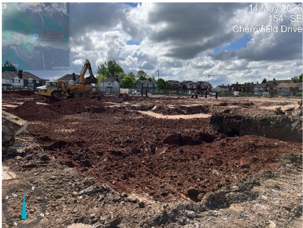
Plate 19 Upfill with Site-Won Granular / Non-Heave Impacted Cohesive Materials
