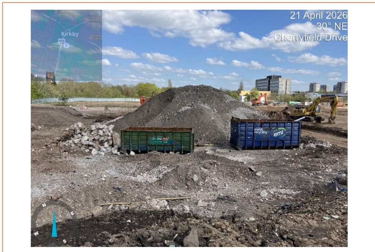
Plate 9 Segregation of Materials and Waste
