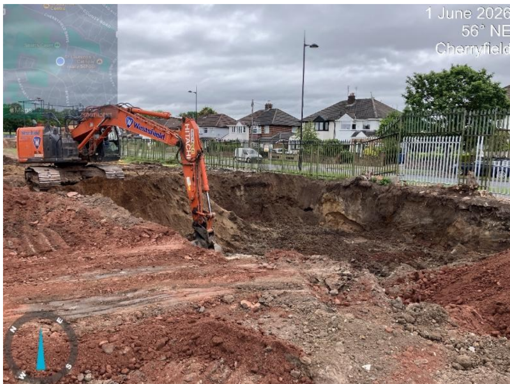
Plate 13 Removal of Heave Impacted Clay Soils
