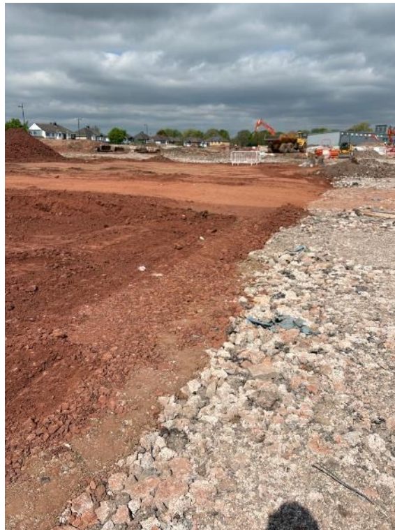
Plate 21 Upfill with Site-Won Granular / Non-Heave Impacted Cohesive Materials
