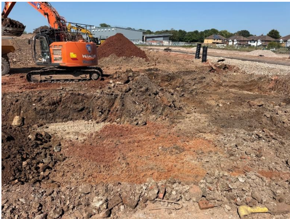
Plate 16 Removal of Heave Impacted Clay Soils
