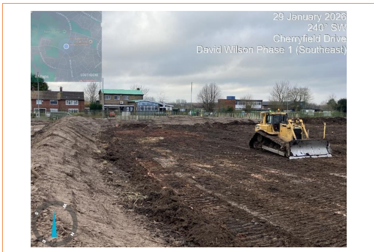
Plate 6 Topsoil Stripping Across David Wilson Phase 1
