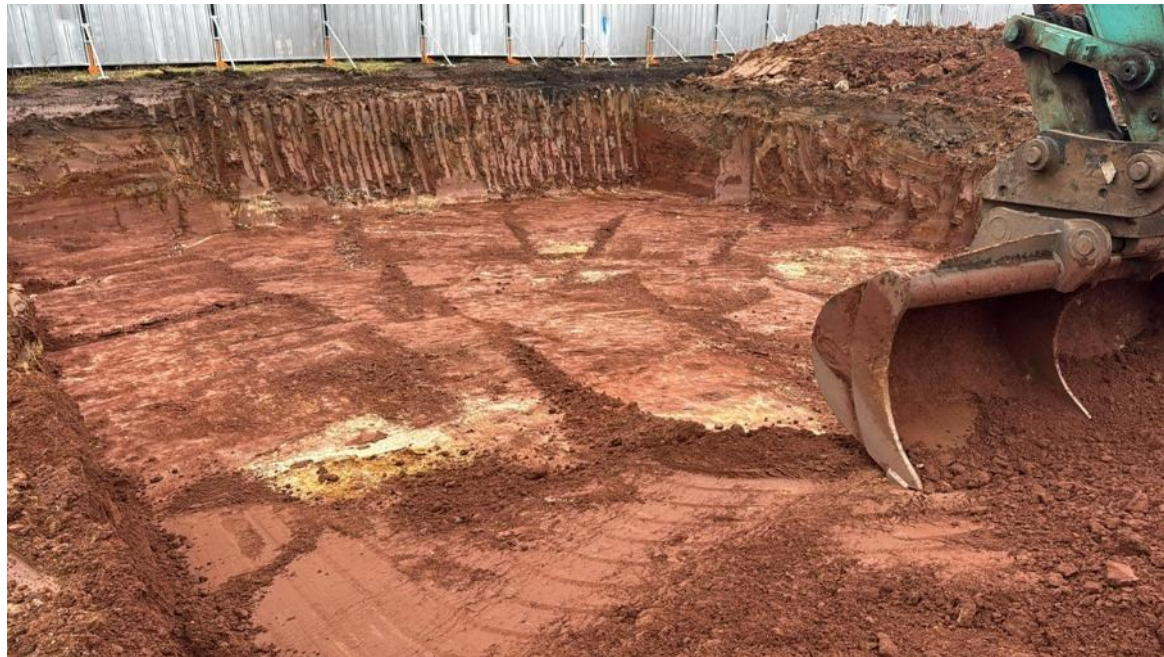
Plate 17 Removal of Heave Impacted Clay Soils
