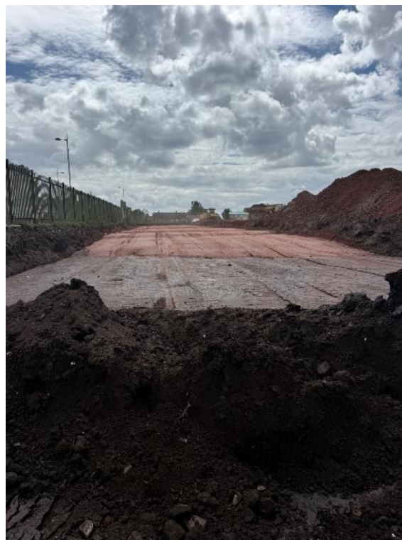
Plate 22 Upfill with Site-Won Granular / Non-Heave Impacted Cohesive Materials
