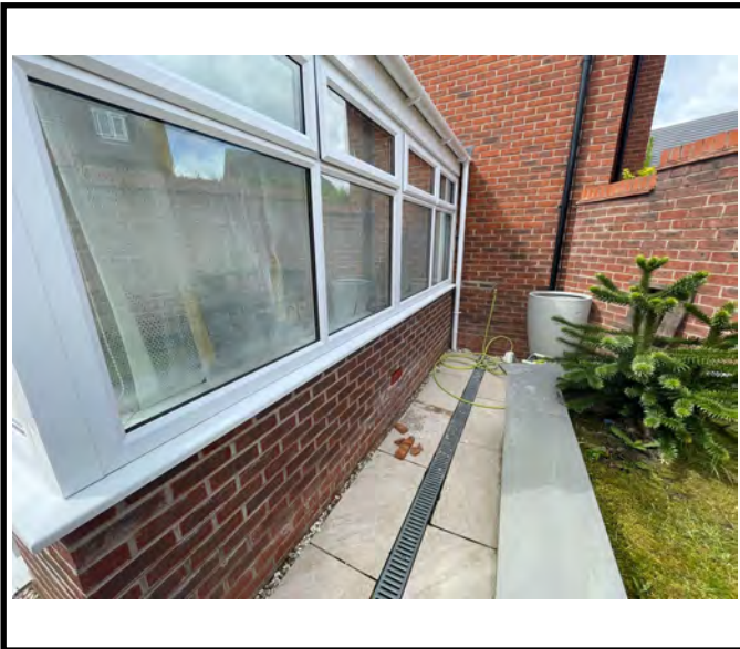
Air bricks installed around the external perimeter of the Conservatory.
